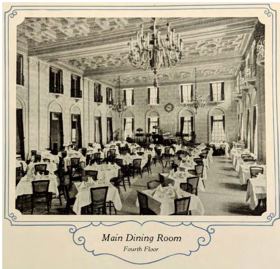
Figure 4: 1926 view of fourth floor Main Dining Room
