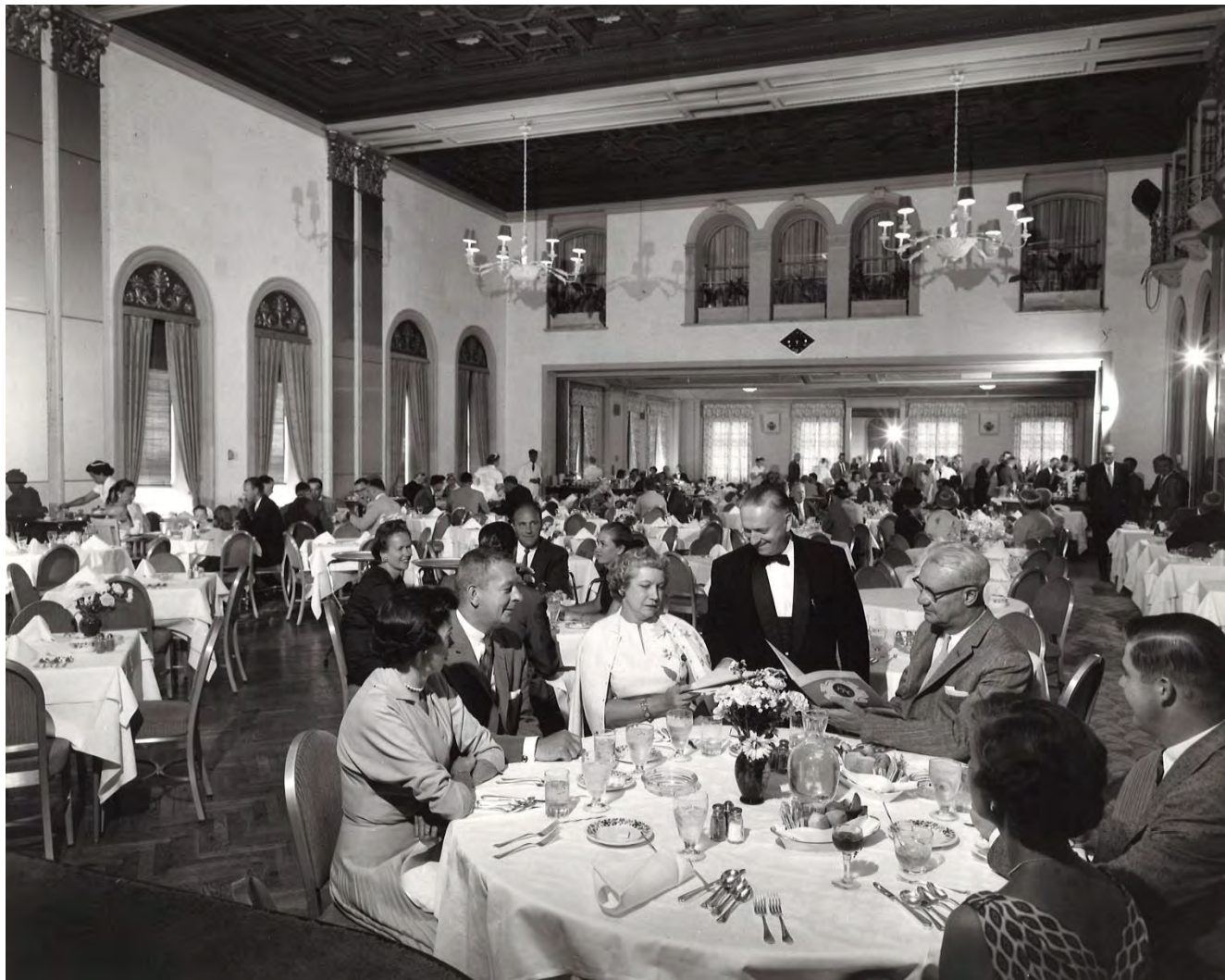
Figure 10: Fourth floor Main Dining Room, c. 1955
