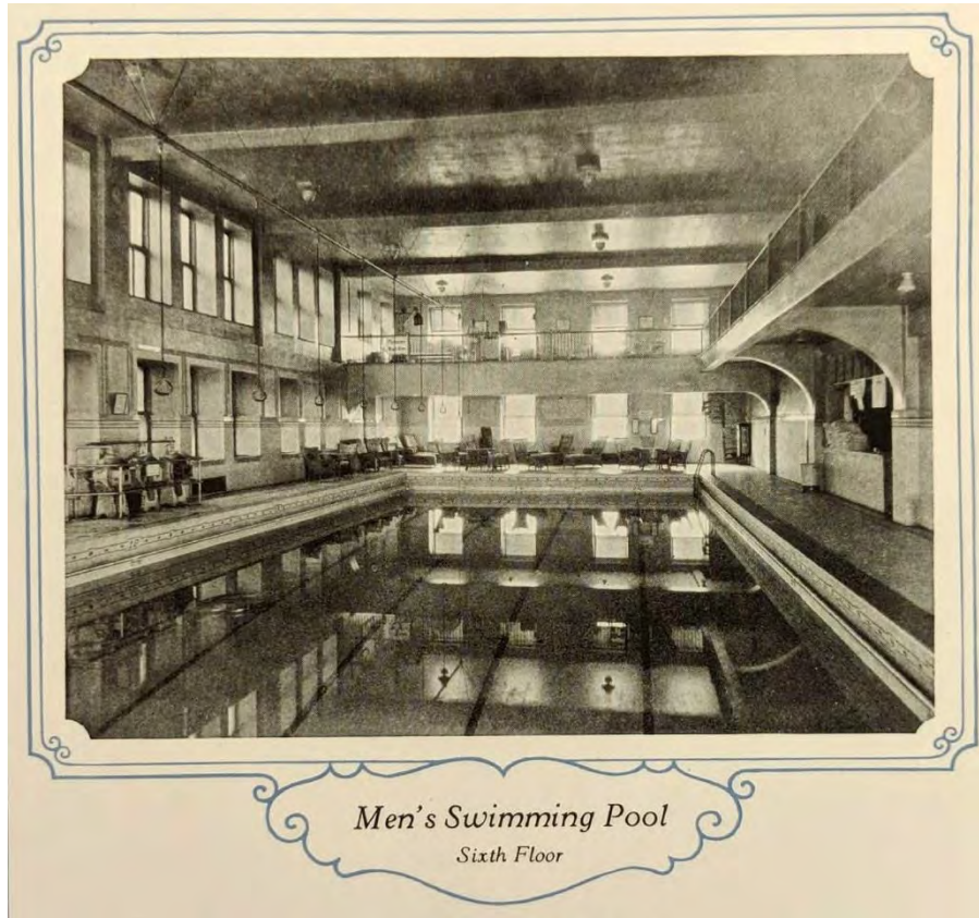
Figure 6: 1926 view of sixth floor Men's Swimming Pool
