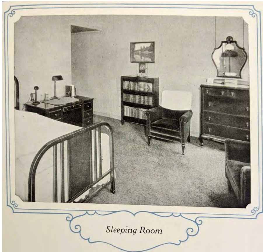
Figure 9: 1926 View of typical upper floor Sleeping Room
