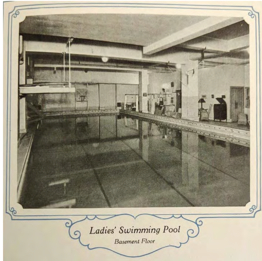
Figure 8: 1926 view of the basement Ladies' Swimming Pool
