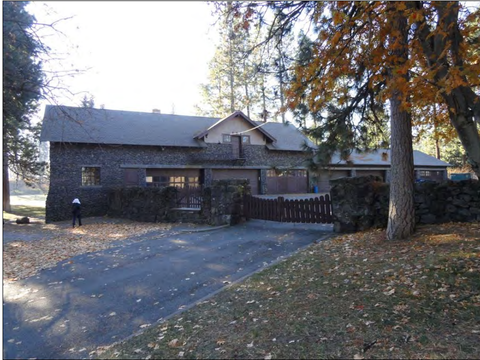
Photo 23. WA_SpokaneCounty_ManitoParkAndBoulevard_0023. Garage No. 2, view southwest.
