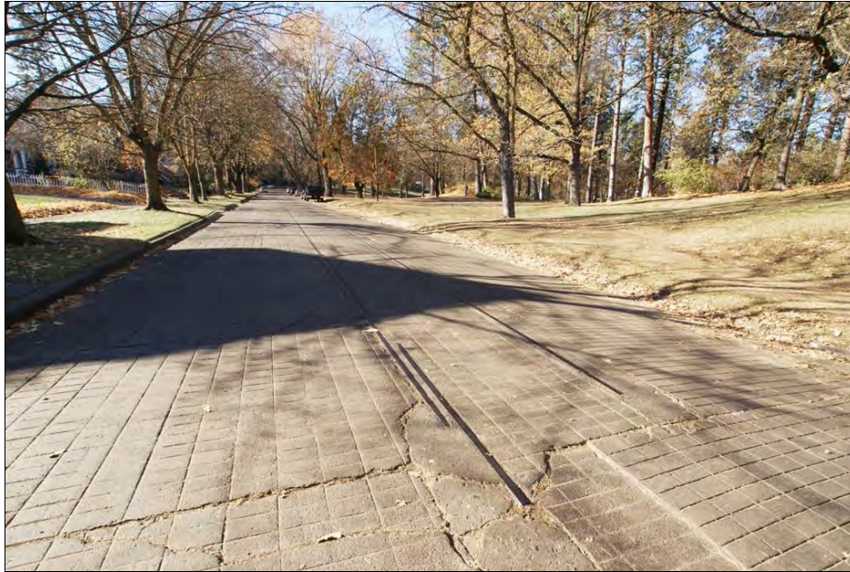
Photo 17. WA_SpokaneCounty_ManitoParkAndBoulevard_0017. Trolley Tracks, view west.
