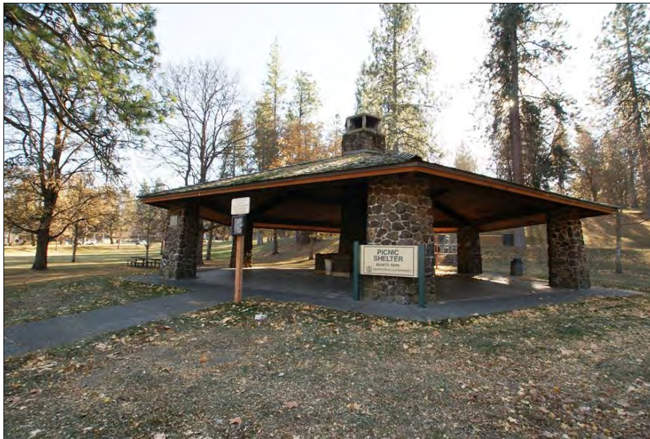
Photo 12. WA_SpokaneCounty_ManitoParkAndBoulevard_0012. Rotary Club Picnic Shelter, view southeast.
