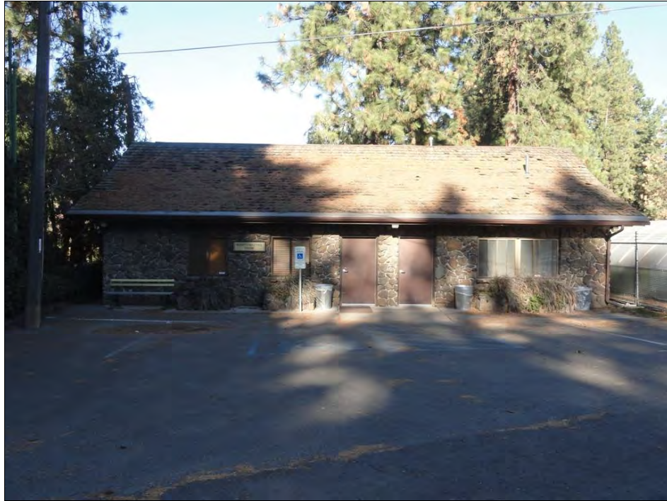
Photo 21. WA_SpokaneCounty_ManitoParkAndBoulevard_0021. Manito Meeting Room, view north.
