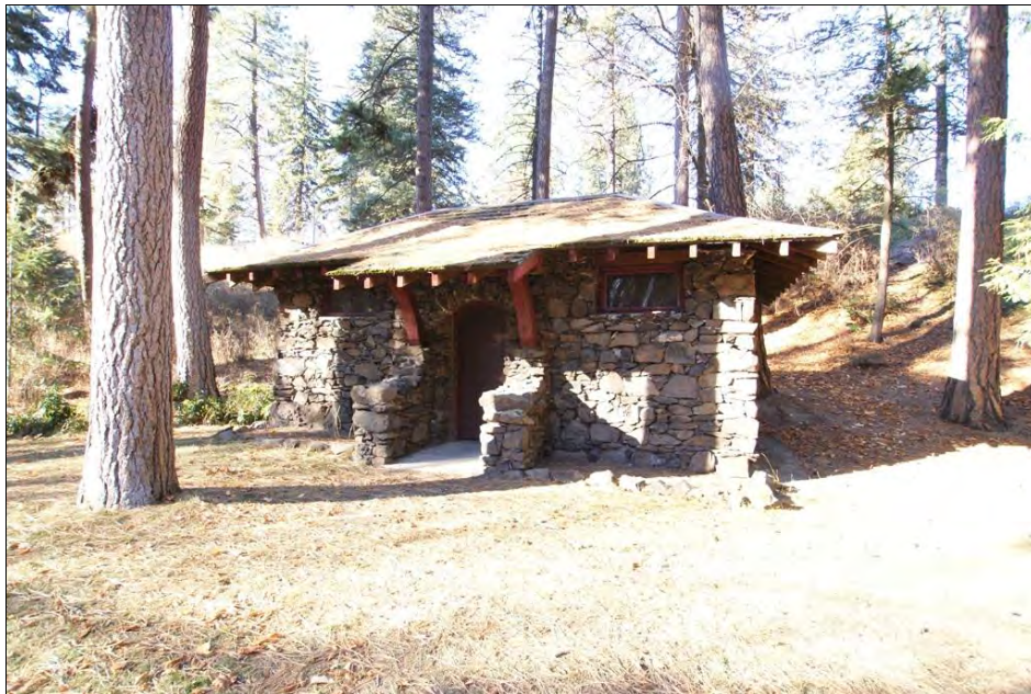
Photo 20. WA_SpokaneCounty_ManitoParkAndBoulevard_0020. Ancillary Building, view west.
