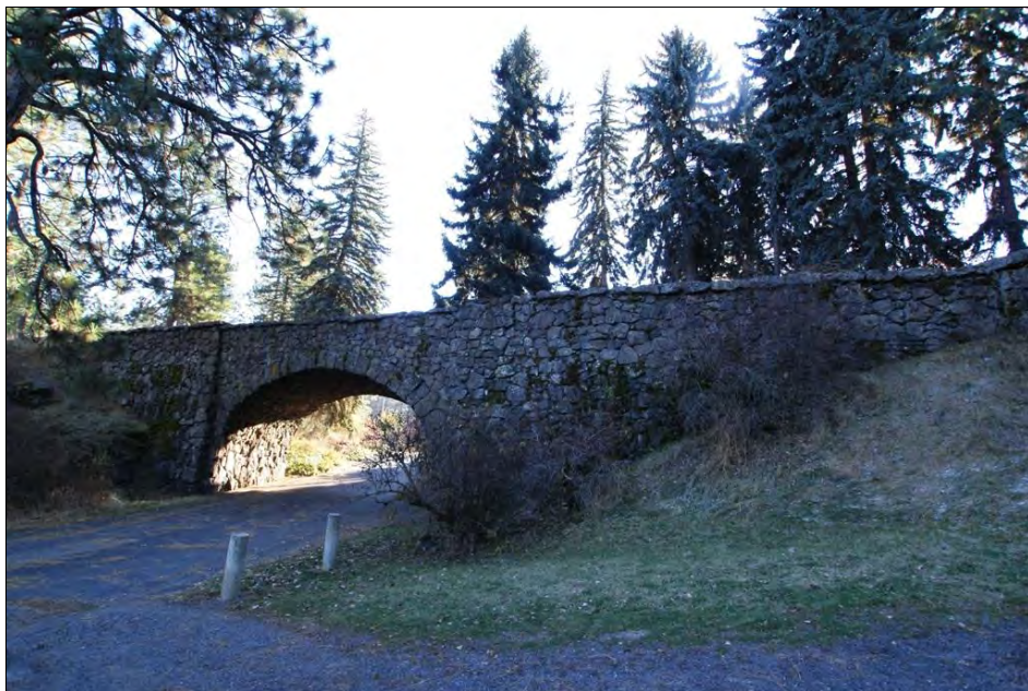
Photo 28. WA_SpokaneCounty_ManitoParkAndBoulevard_0028. Loop Road Bridge, view southwest.
