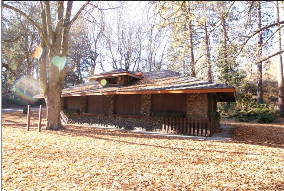
Photo 19. WA_SpokaneCounty_ManitoParkAndBoulevard_0019. Park Bench Café, view southwest.
