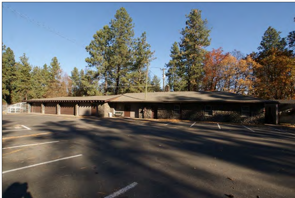
Photo 22. WA_SpokaneCounty_ManitoParkAndBoulevard_0022. Garage No. 1, view northeast.
