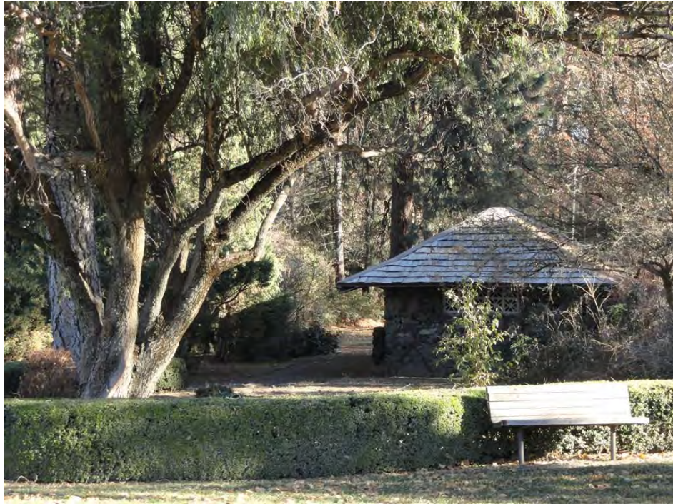
Photo 25. WA_SpokaneCounty_ManitoParkAndBoulevard_0025. Storage Shed, view east.
