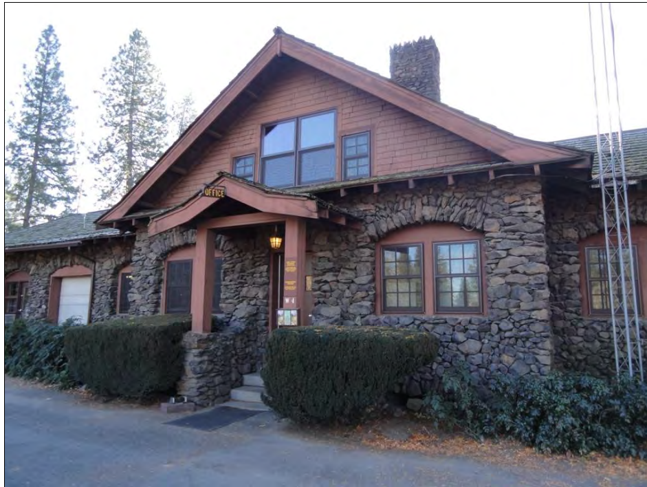
Photo 5. WA_SpokaneCounty_ManitoParkAndBoulevard_0005. Detail of Administrative Offices, view south.
