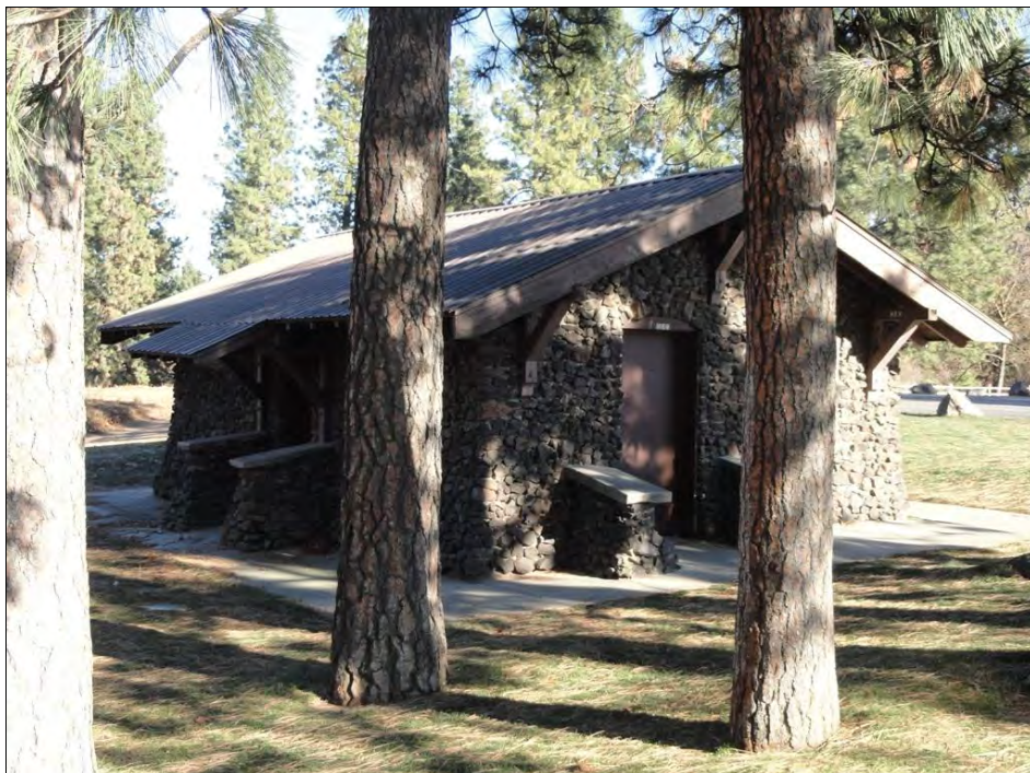
Photo 24. WA_SpokaneCounty_ManitoParkAndBoulevard_0024. Upper Manito Restroom, view northeast.
