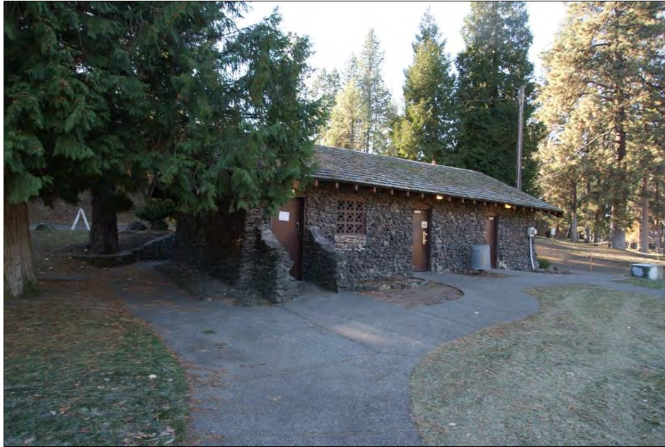
Photo 15. WA_SpokaneCounty_ManitoParkAndBoulevard_0015. Restroom No. 1, view southwest.
