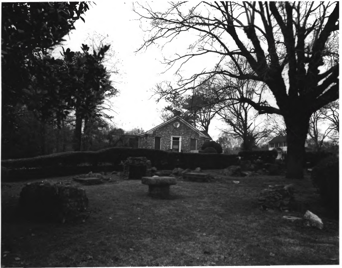
CEDARTOWN WATERWORKS, WOMAN'S BUILDING, AND BIG SPRING PARK HISTORIC DISTRICT CEDARTOWN, POLK COUNTY, GEORGIA PHOTOGRAPH 31 OF 32
