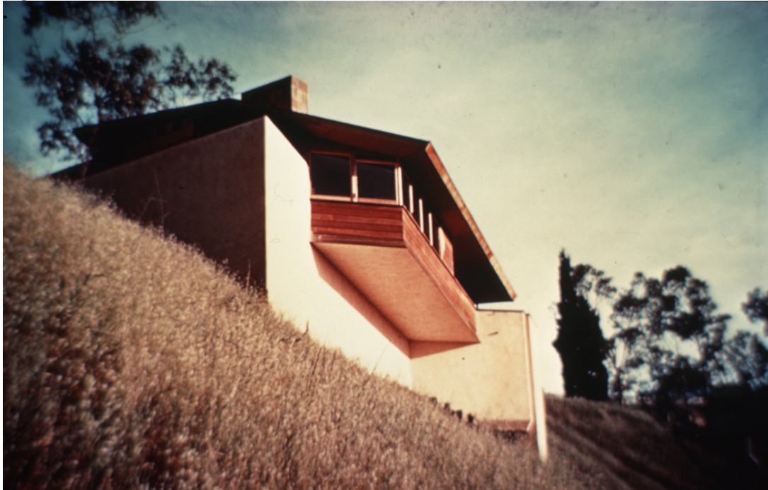
View of north and west façades, facing southeast (© The John Lautner Foundation, courtesy of Frank Escher, date of photograph unknown)
