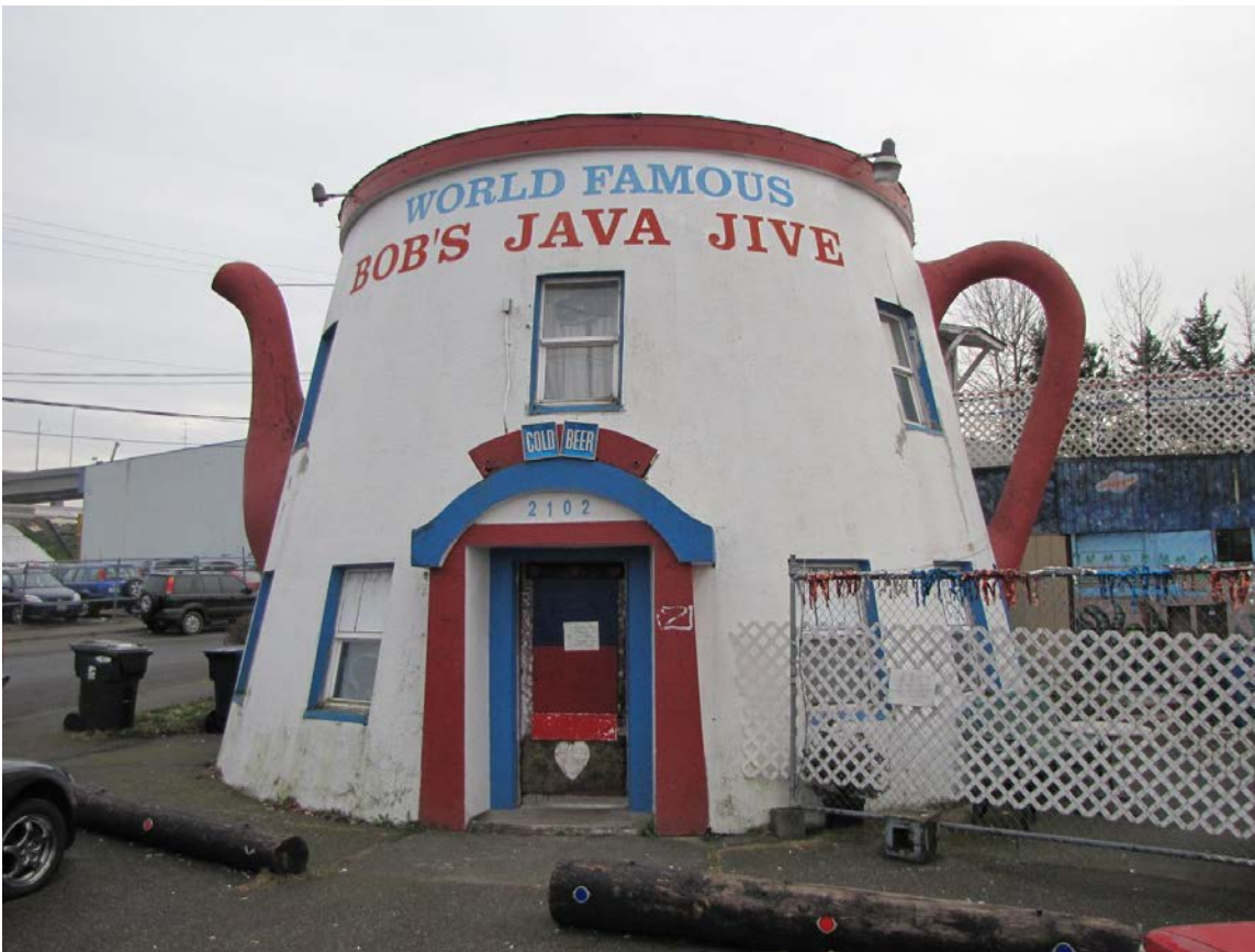
The Coffee Pot Restaurant – Main elevation: 1 of 19.
