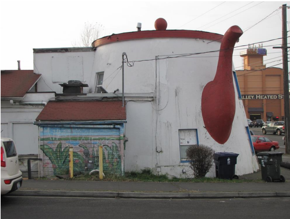
The Coffee Pot Restaurant – East elevation, showing part of rear additions: 3 of 19.
