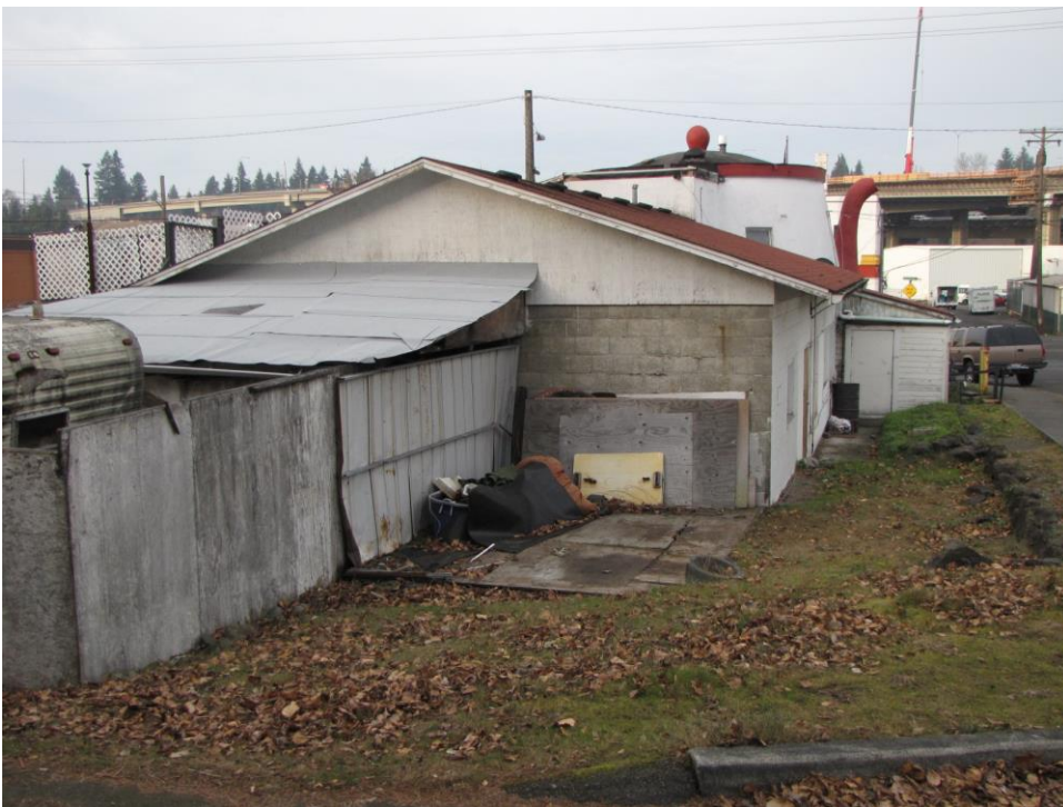
The Coffee Pot Restaurant – South elevation, showing rear additions: 6 of 19.
