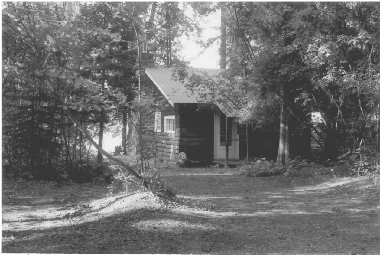
Mars Cabin, Howes' Lake McDonald Cottage Sites Historic District Glacier National Park, Flathead County, Montana Photograph No. 4
