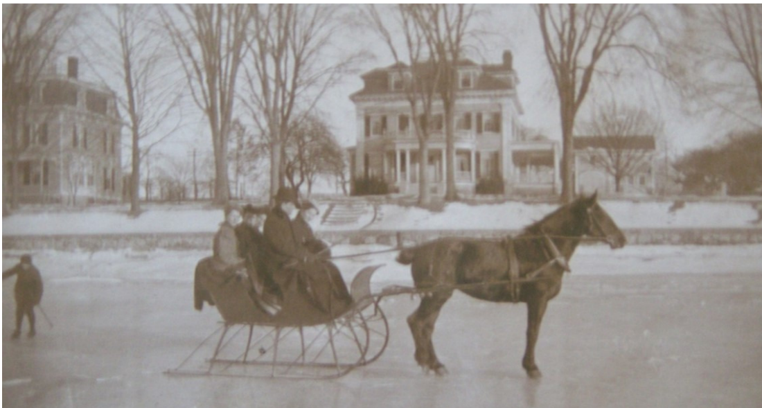
Fig. 5 View looking east across Pawcatuck River, toward Thomas Perry, Jr. House (2 Margin Street) on left and Charles Perry House (4 Margin Street) on right, early 20 th century. Collection of Harvey C. Perry II, Westerly, RI.
