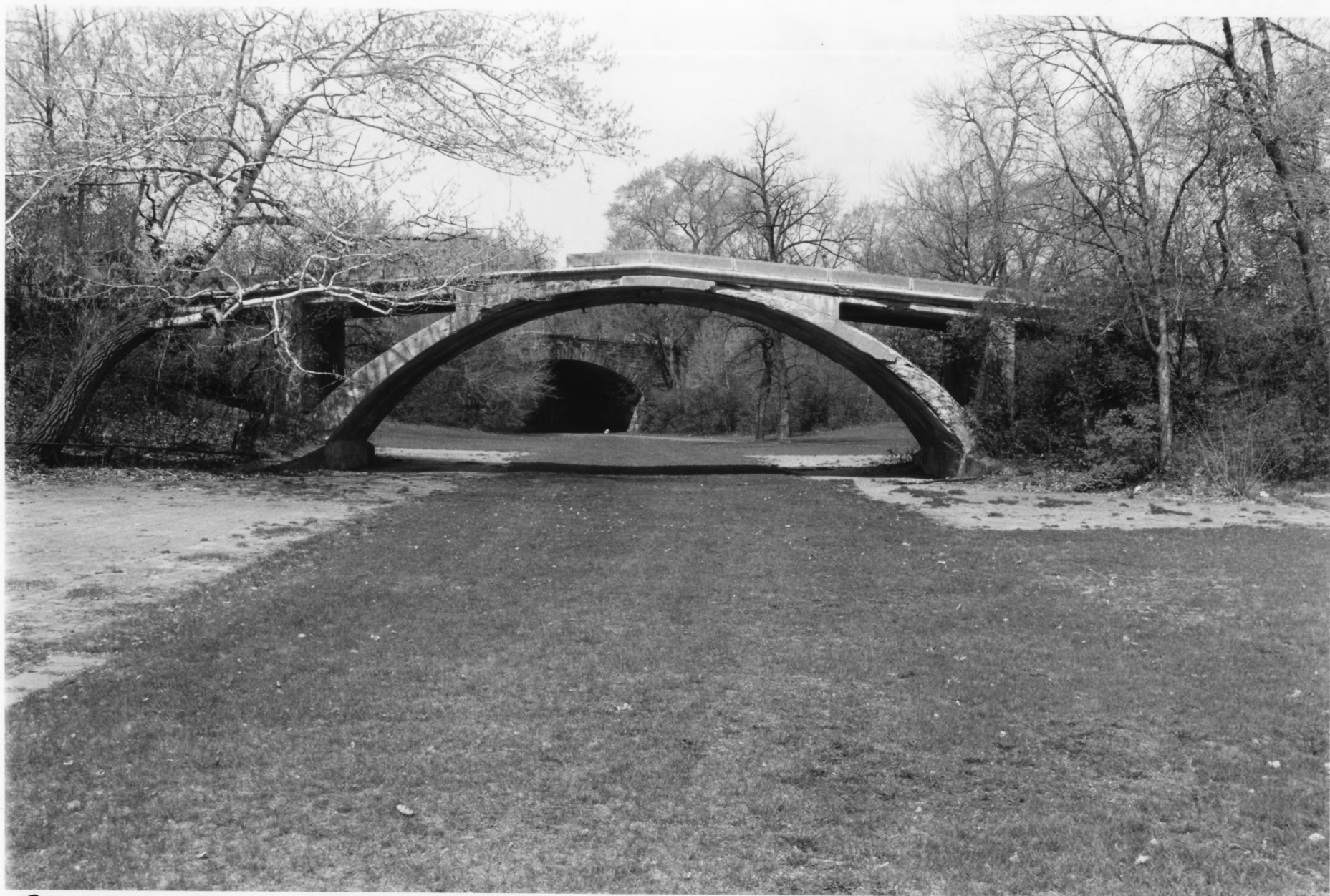
BRIDGE NO. L-5853 ST. PAUL, RAMSEY CO., MN PHOTO I.D. 09738# 15
