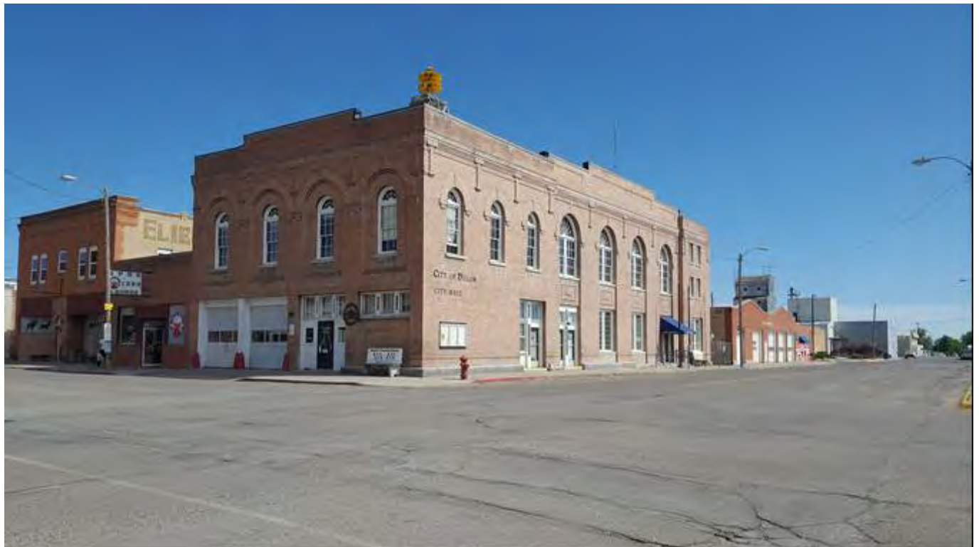
Overview of Dillon City Hall, view to the north, south and east elevations.
