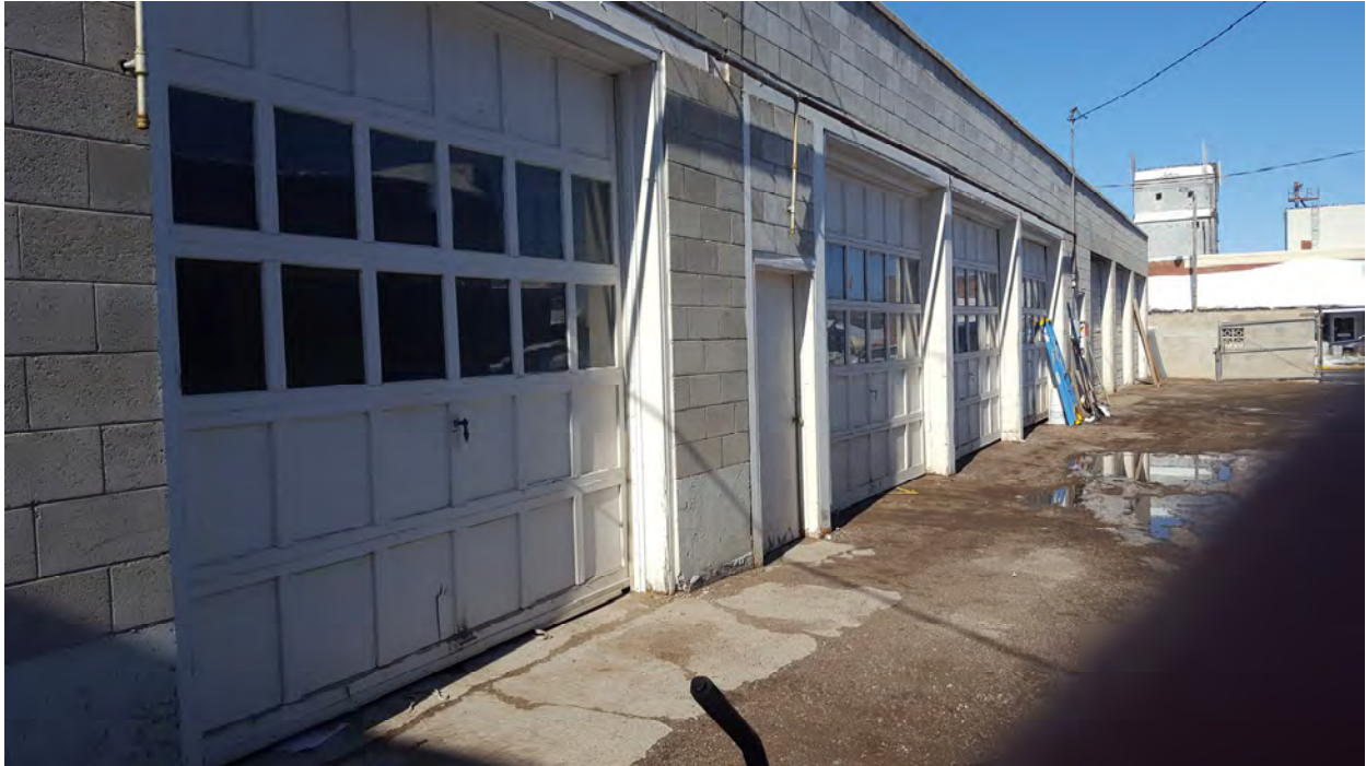
City Shops Building, view to the north, east elevation. MT_BeaverheadCounty_DillonCityHallHistoricDistrict_0014
