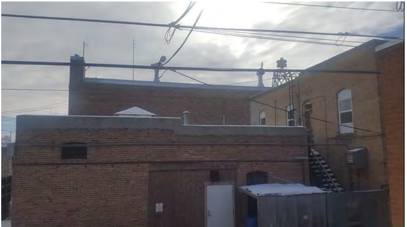
Dillon City Hall, view to the southeast, west elevation. MT_BeaverheadCounty_DillonCityHallHistoricDistrict_0004
