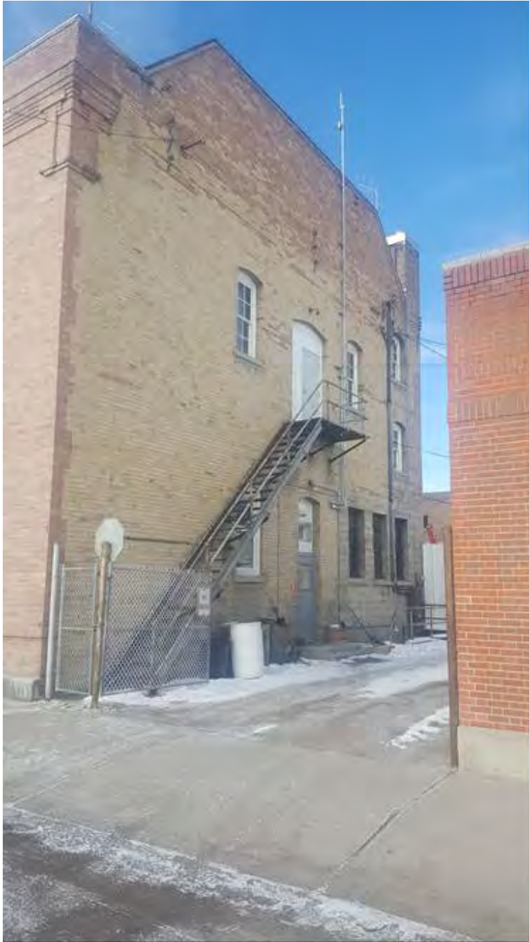
Dillon City Hall, view to the west, north elevation. MT_BeaverheadCounty_DillonCityHallHistoricDistrict_0003
