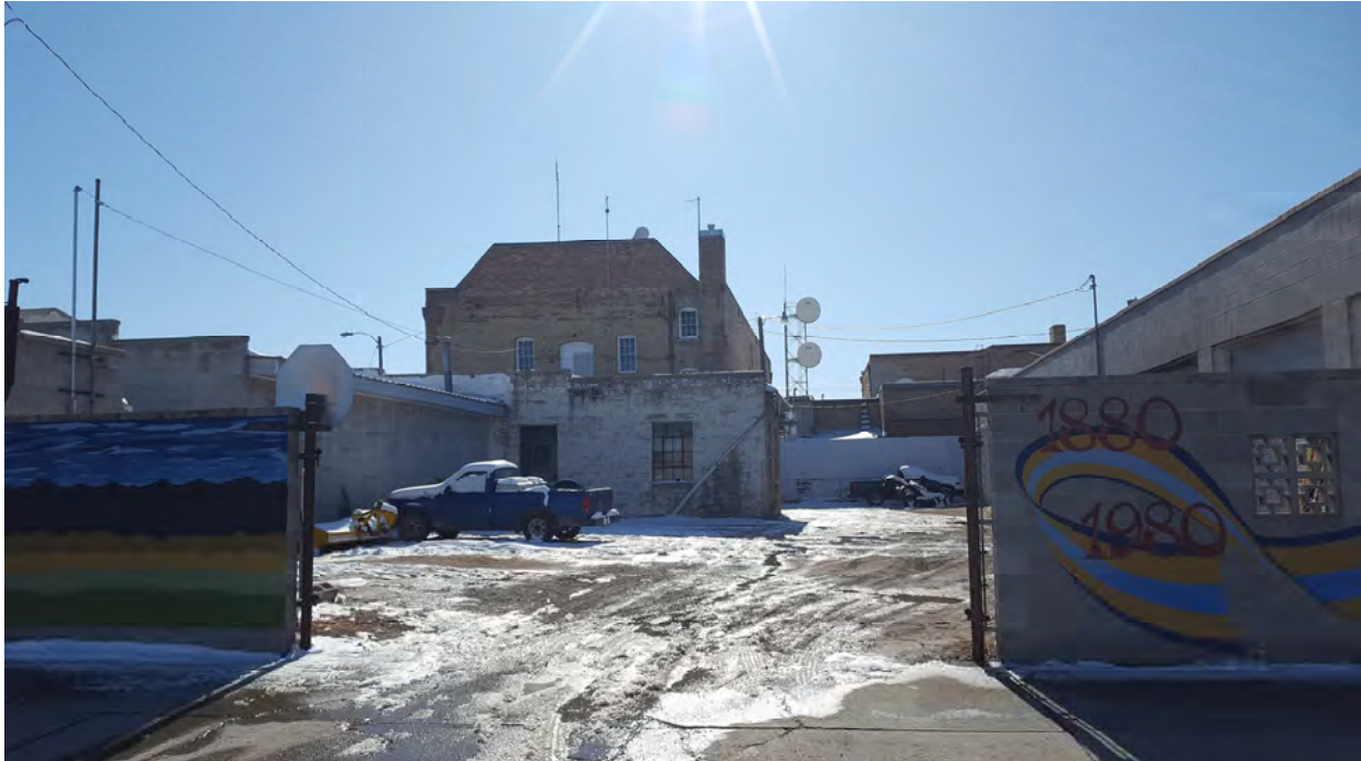
City Well #3 Building and concrete block wall, view to the southwest, north elevation. MT_BeaverheadCounty_DillonCityHallHistoricDistrict_0013
