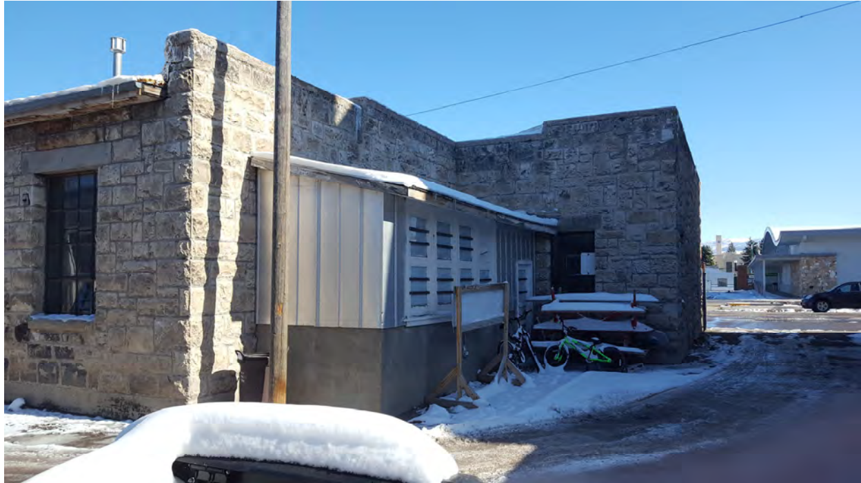
City Shop and Storage Garage, view to the east, west and south elevations. MT_BeaverheadCounty_DillonCityHallHistoricDistrict_0010
