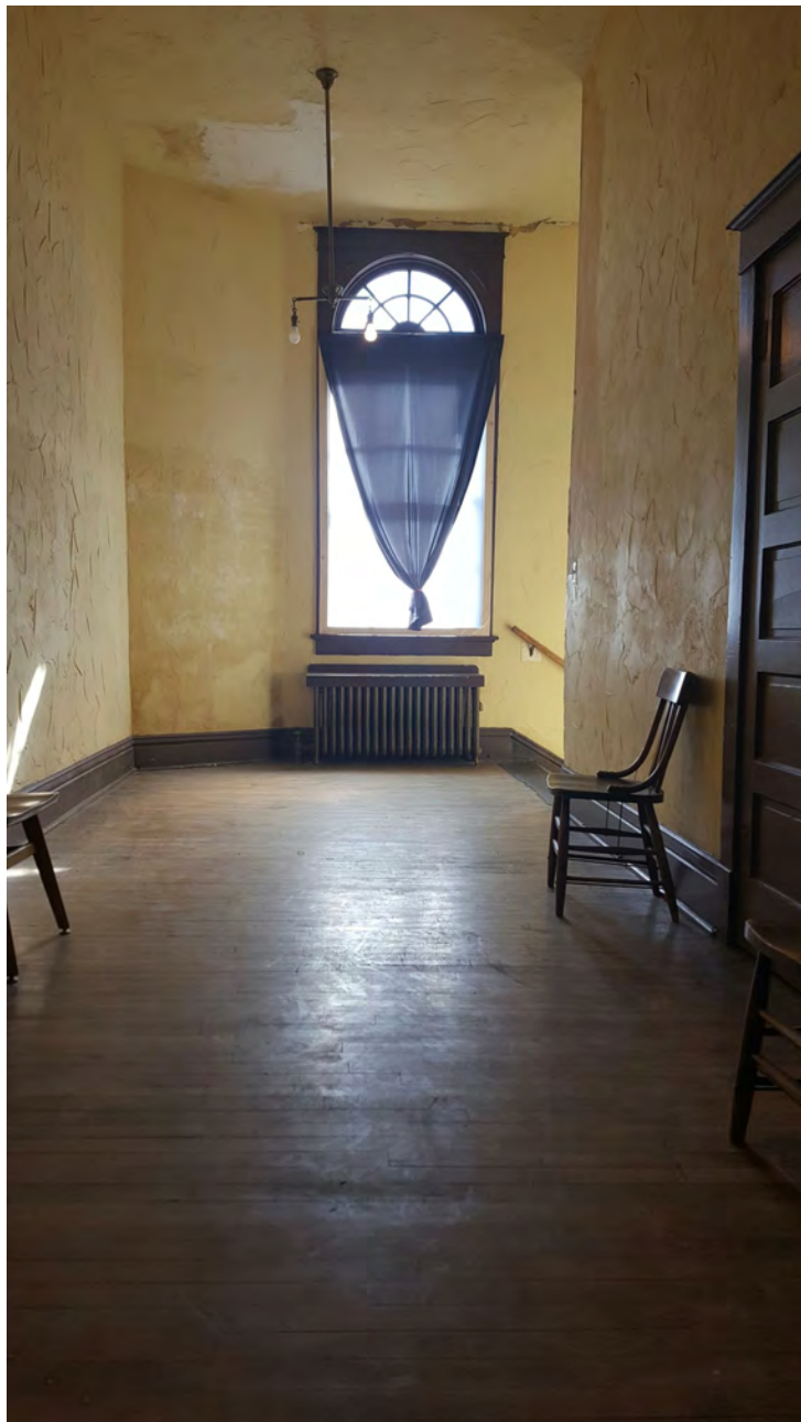
Dillon City Hall, second story landing
