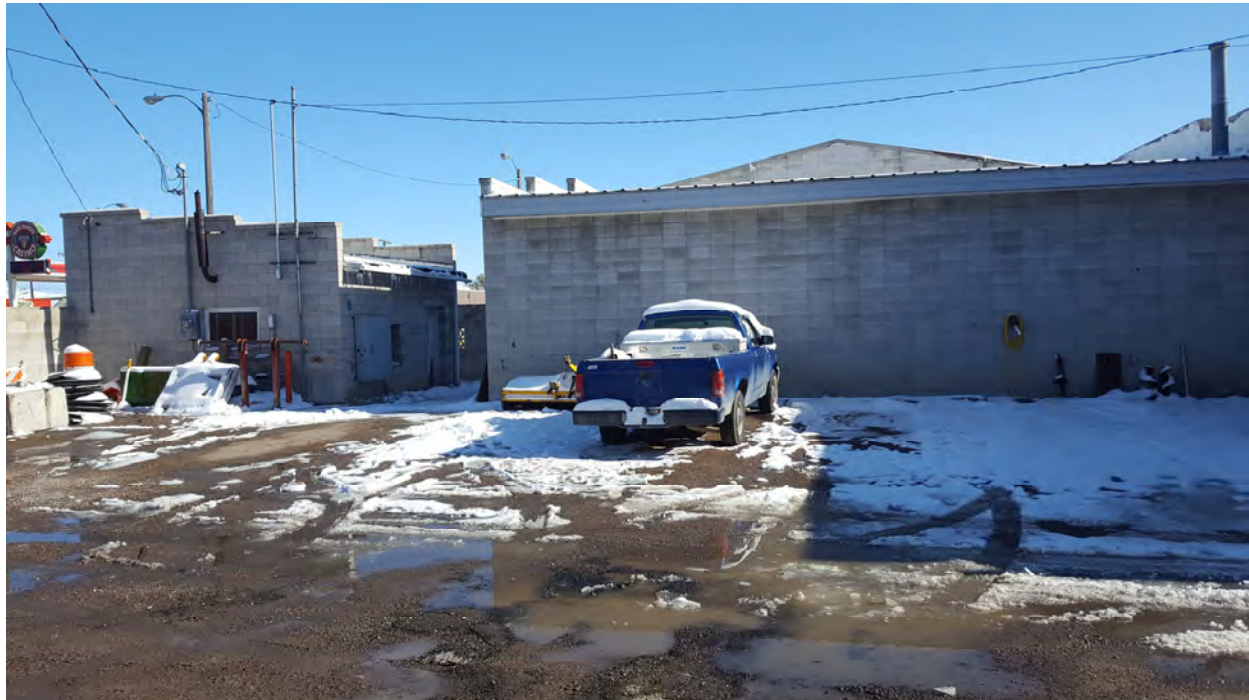
City Shop and Storage Garage (right), view to the southeast, west elevation, and City Well #3 Building (right), south and west elevations.
