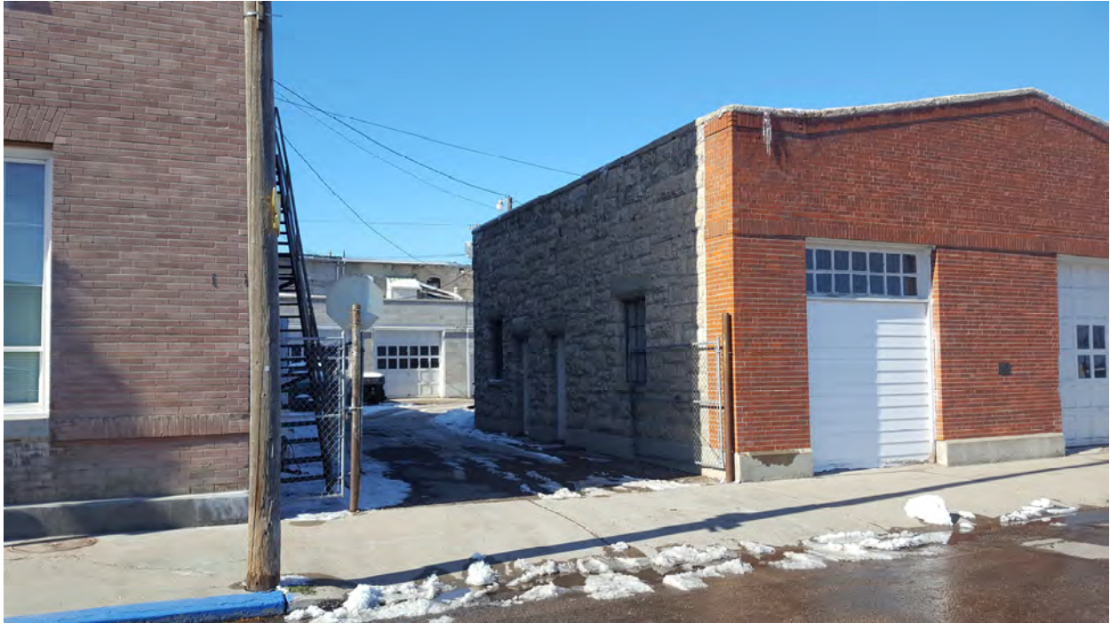
City Shop and Storage Garage, view to the north, south elevation. MT_BeaverheadCounty_DillonCityHallHistoricDistrict_0009
