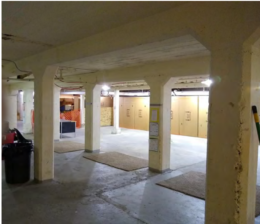
Dillon City Hall, basement, former shooting range.
