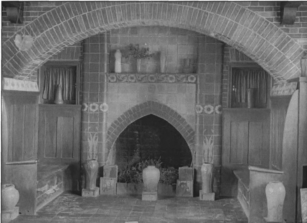
Figure H12. The salesroom wing of the pottery displayed art pottery designs as well as interior architectural products, such as tile fireplaces. SOURCE: Denver Public Library, Western History and Genealogy Department, photograph collection, call number X-14311, c. 1910s.
