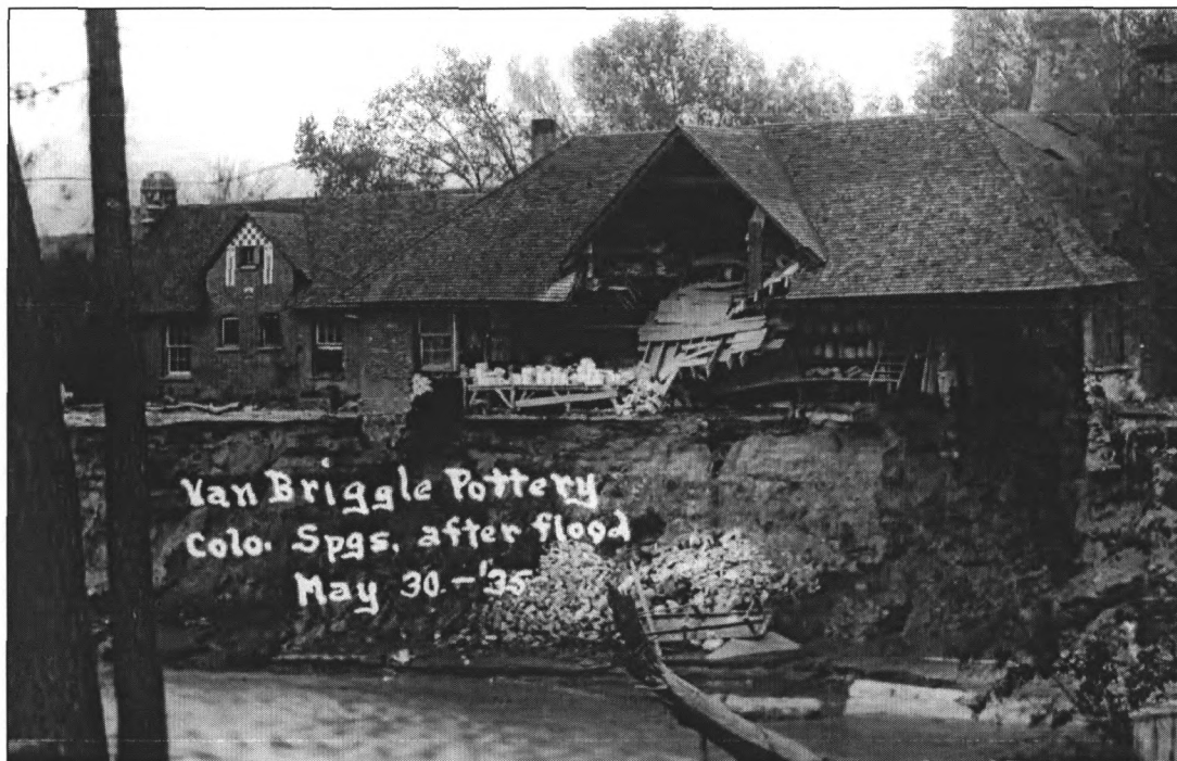
Figure H14. The 1935 Memorial Day flood of Monument Creek severely damaged the pottery's molding/casting wing and left water, sand, and mud throughout the rest of the plant. SOURCE: Colorado Springs Museum, Starsmore Center for Local History, Van Briggle photographic collection, accession number S 2000.0143.0001.
