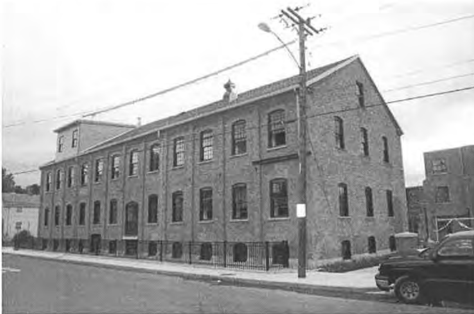
Photo 5 of 20: Exterior view of the Silk Mill Apartments showing the north and west elevations of Building 1 and a portion of Building 4 (camera facing southeast).
