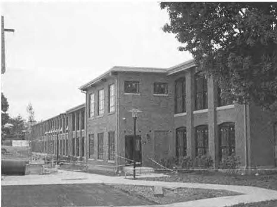
Photo 10 of 20: Exterior view of the Silk Mill Apartments showing the south and east elevations of Building 7 (camera facing northwest).
