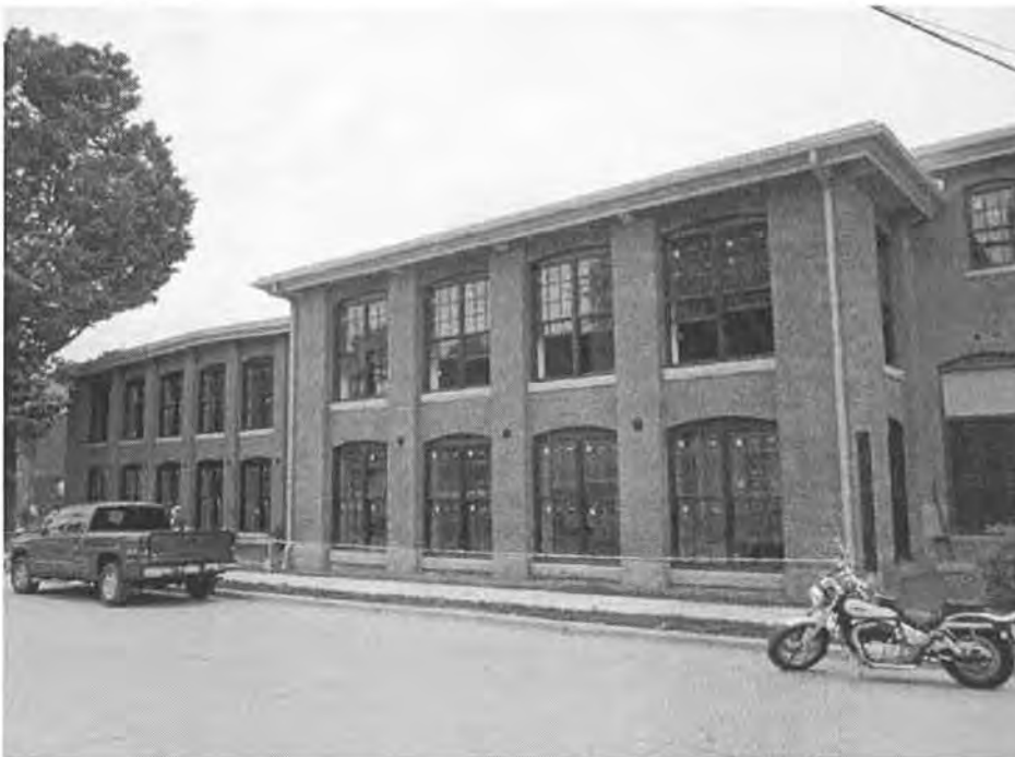
Photo 8 of 20: Exterior view of the Silk Mill Apartments showing the east and north elevations of Buildings 3 & 7 (camera facing southwest).
