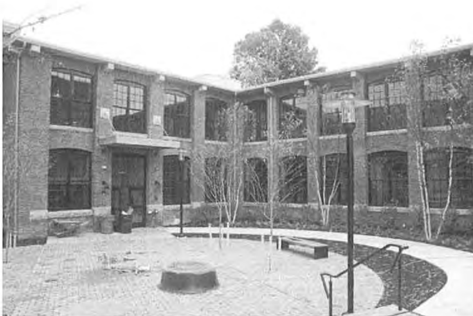
Photo 14 of 20: Courtyard entrance to the Silk Mill Apartments showing the west and north elevations of Buildings 3 & 7 (camera facing southeast).
