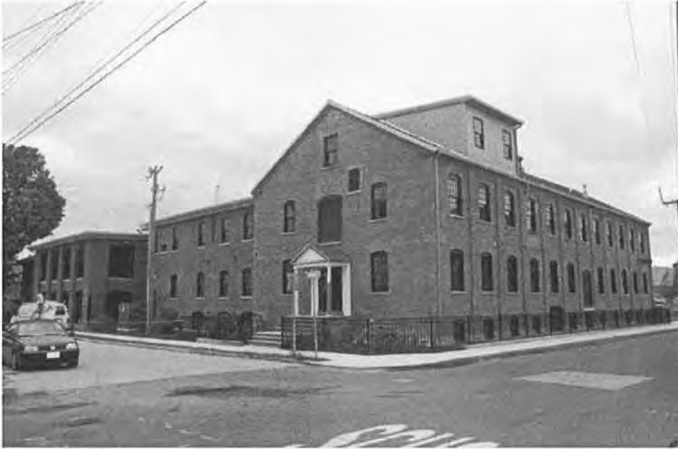
Photo 1 of 20: Exterior view of the Silk Mill Apartments showing the east and north elevations of Buildings 3, 1A, and 1 (camera facing southwest).
