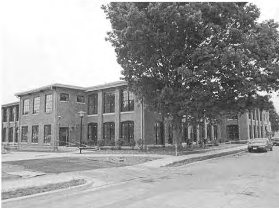
Photo 9 of 20: Exterior view of the Silk Mill Apartments showing the south and east elevations of Buildings 7 & 3 (camera facing northwest).
