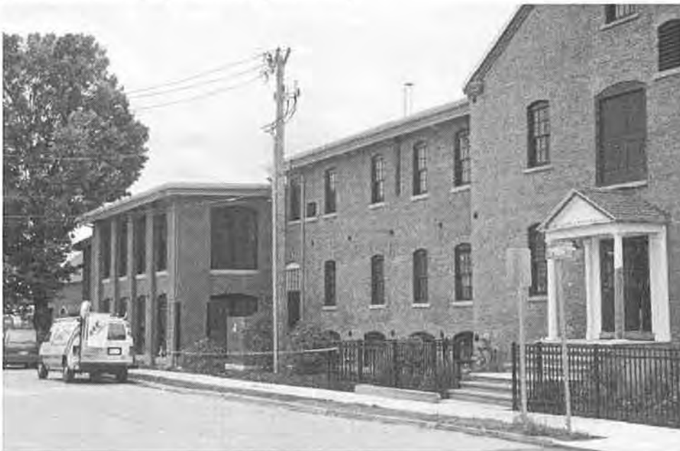
Photo 6 of 20: Exterior view of the Silk Mill Apartments showing the north and east elevations of Building 11 (barn), 3, 1A & 1 (camera facing southwest).
