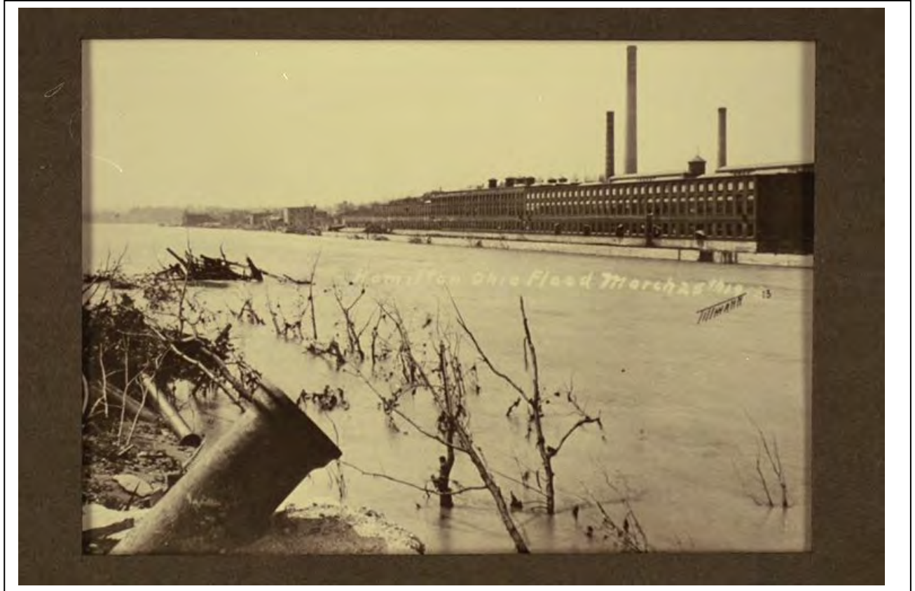
Figure 8: No. 2 Mill from east bank of Great Miami River, 1913, Hamilton Lane Library
