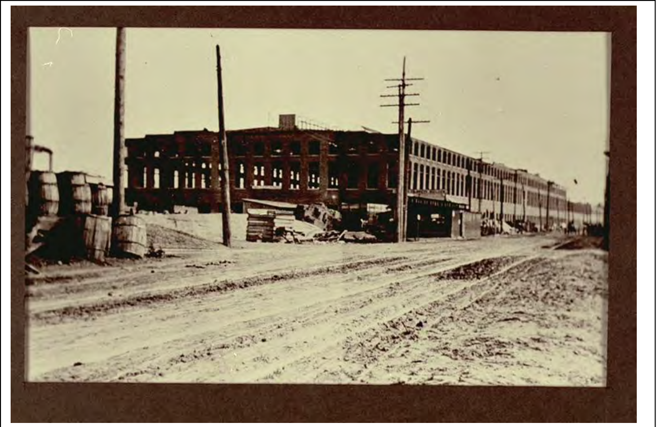
Figure 7: No. 2 Mill under construction, 1906, Hamilton Lane Library
