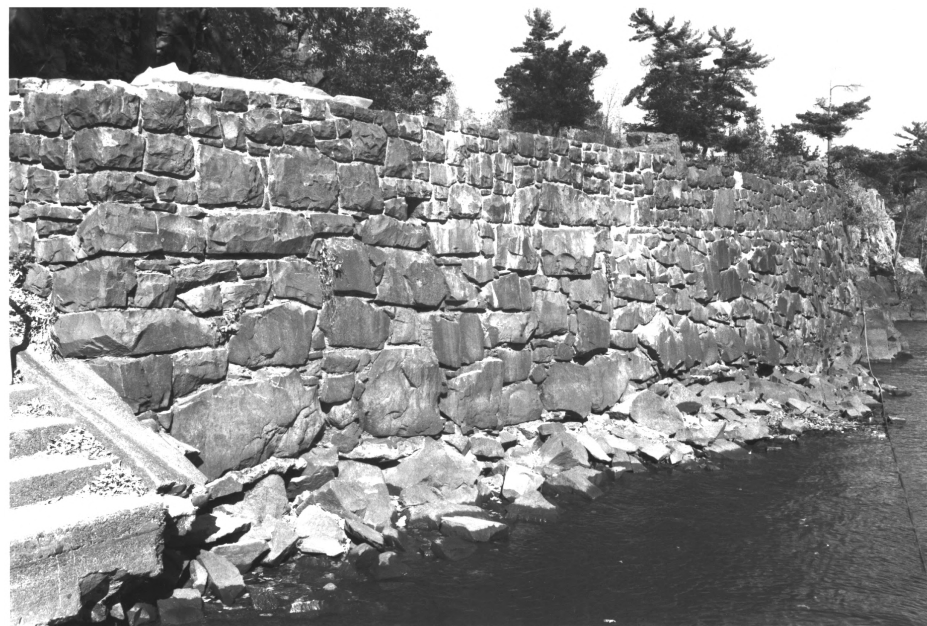
INTERSTATE STATE PARK CHISAGO CO., MN STRUCTURE# 6 PHOTO I.D. 09336#24
