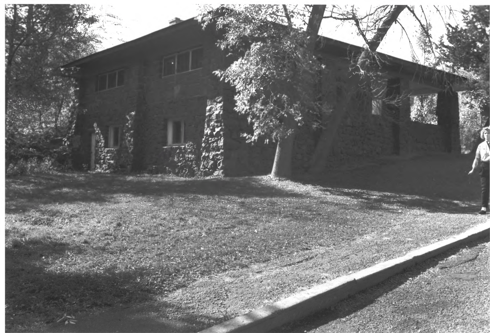
INTERSTATE PARK CHISAGO CO., MN BLDG #1 PHOTO I.D. 09336 #16
