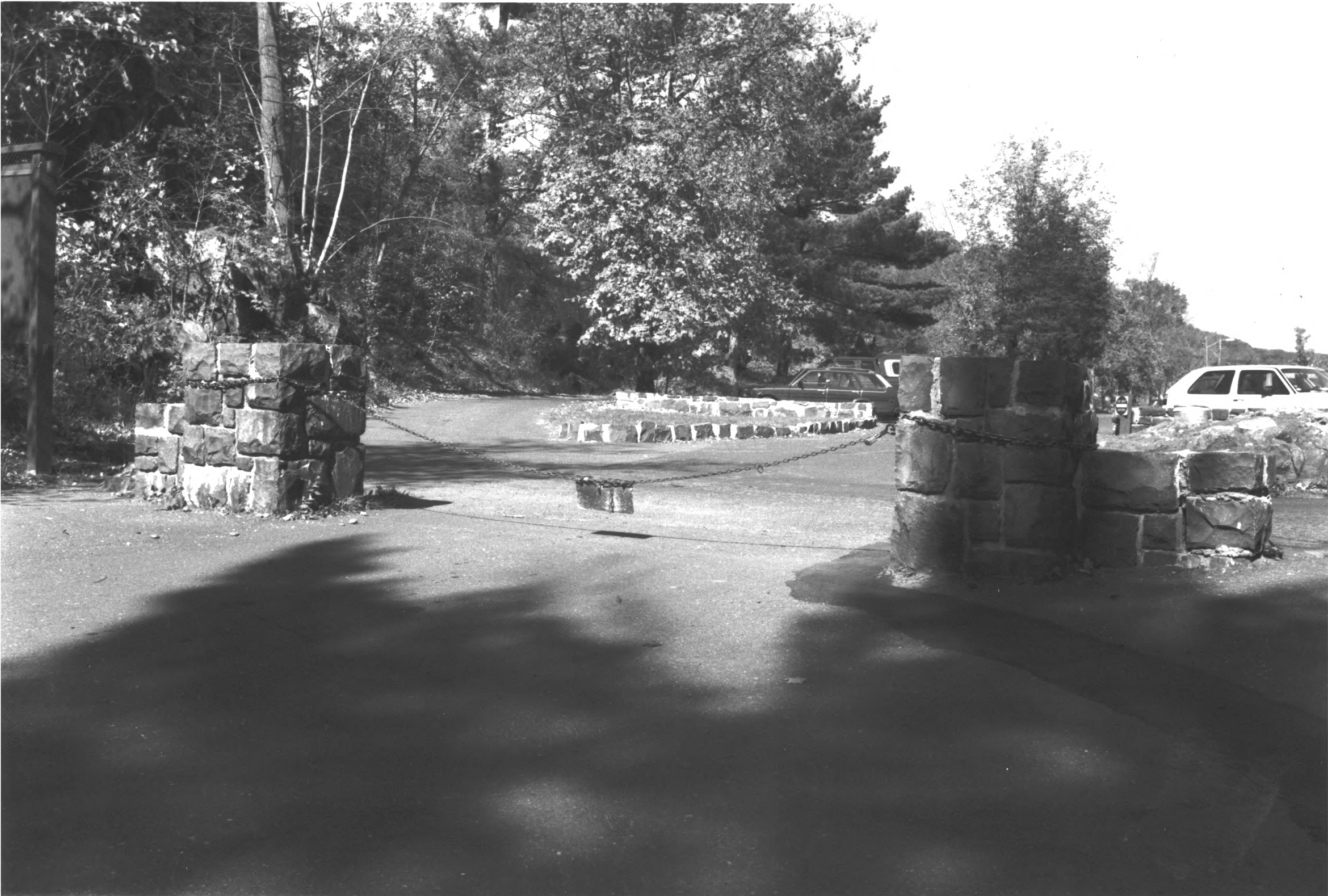
INTERSTATE STATE PARK CHISAGO CO., MN [REDACTED] STRUCTURE # 4 PHOTO I.D. 09336#18
