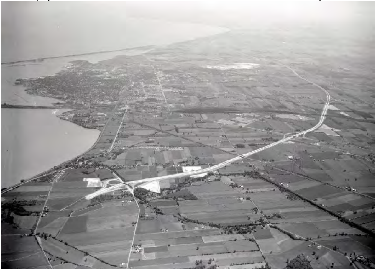
Figure 7: Aerial Photo of Construction of Ohio SR 2 Bypass around Sandusky, September 1963. Source: Tom Root Aerial Photograph collection – Sandusky Library Archives Research Center.
