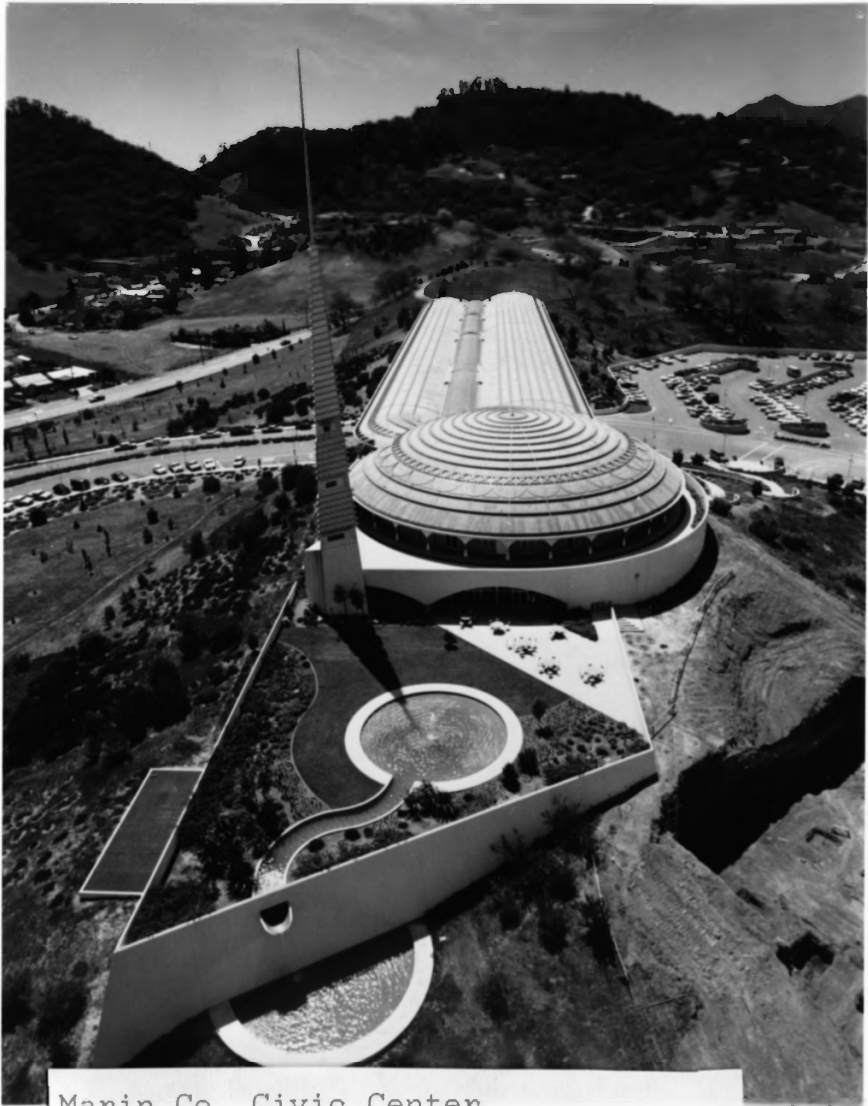
Marin Co. Civic Center San Rafael, Ca. Administration Bldg.c. 1958 from N. Photo: Woodbridge - Aaron Green
