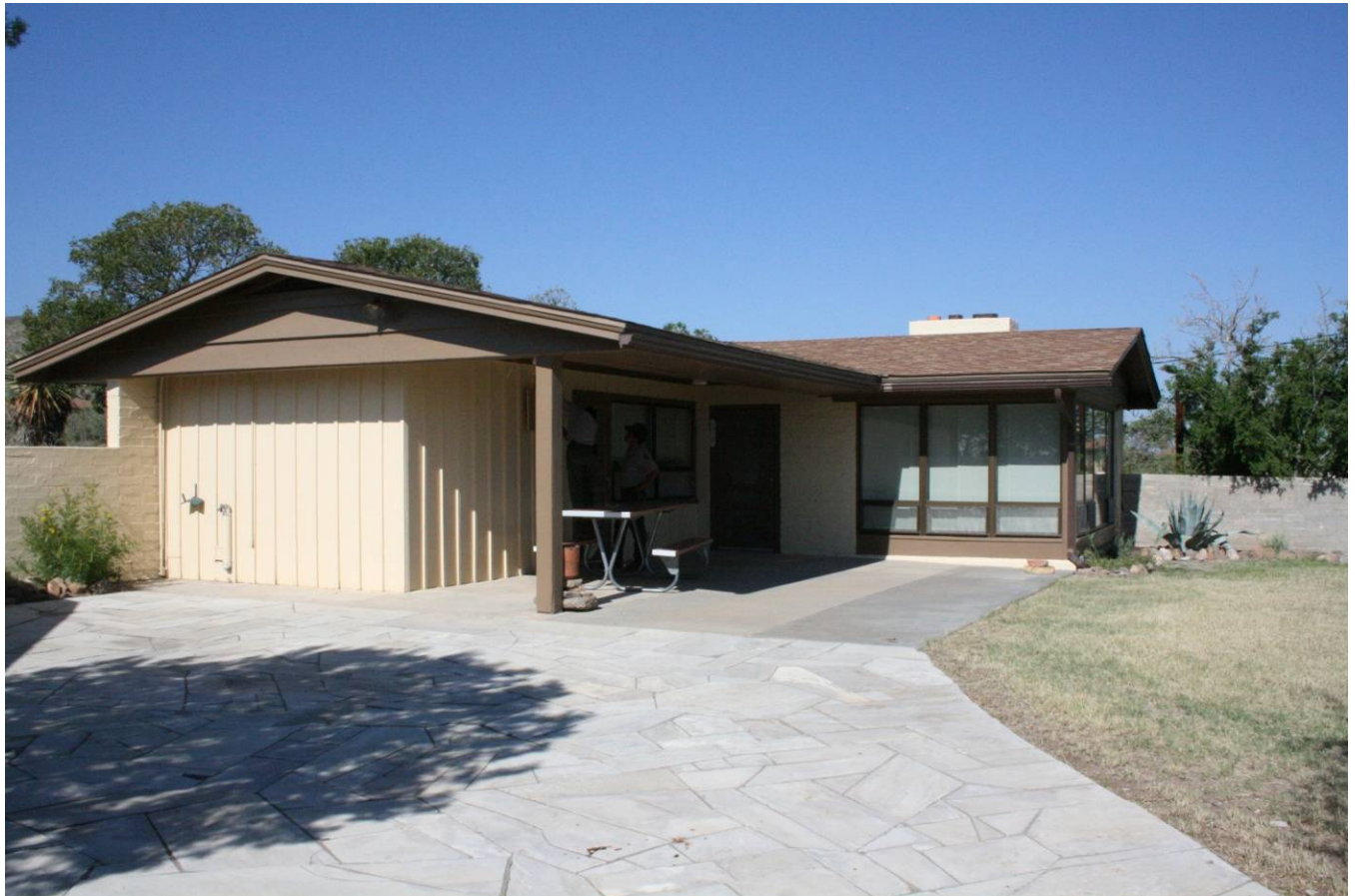
Rear of superintendent's residence (building 203) facing west
