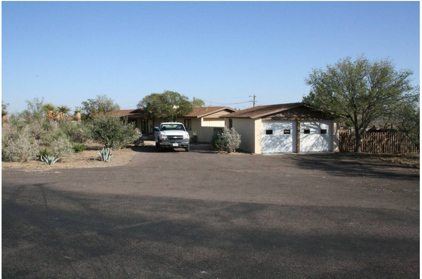
Front of superintendent's residence (building 203) facing north
