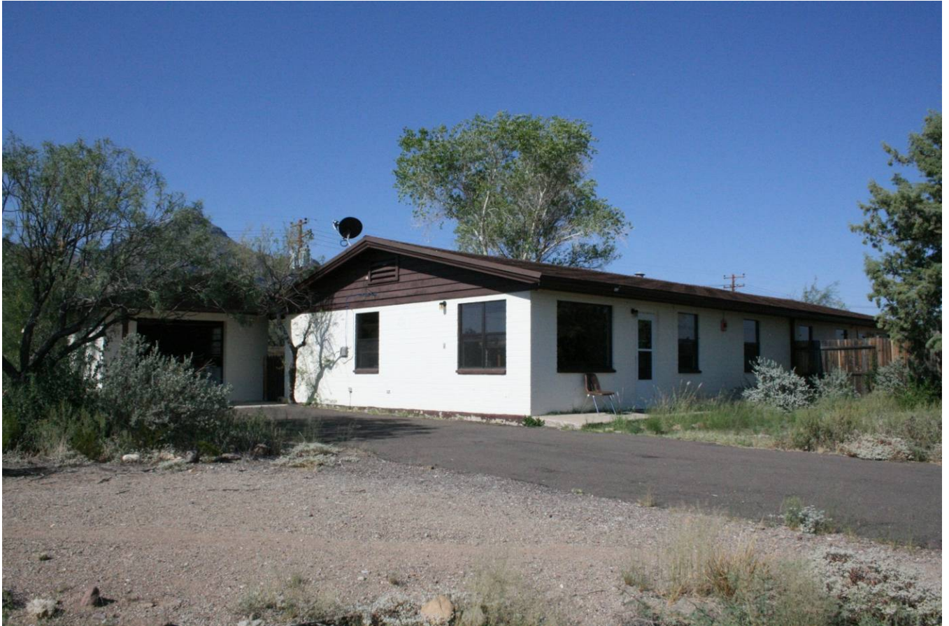
Front of teacherage (residence 236a/236b – duplex with two (2 bedroom, 1 bath units) facing southwest
