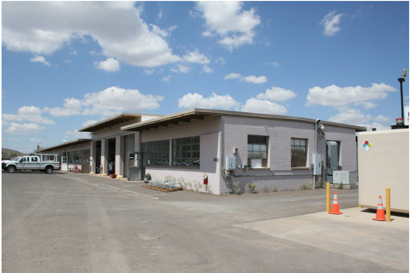
Front and northeast façades of maintenance building facing northwest
