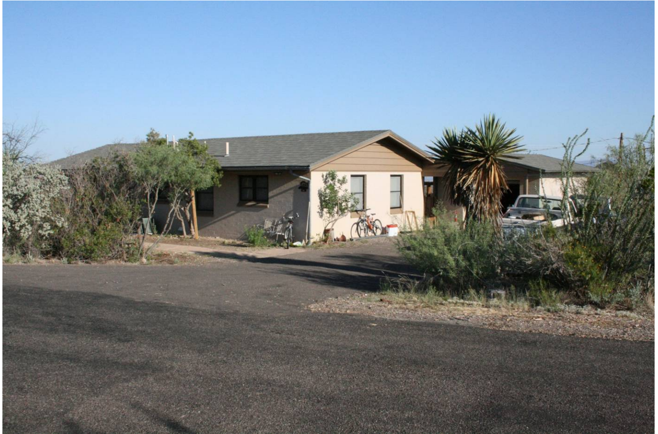
Front of residence 320 (2 bedroom, 1 bath) facing northwest
