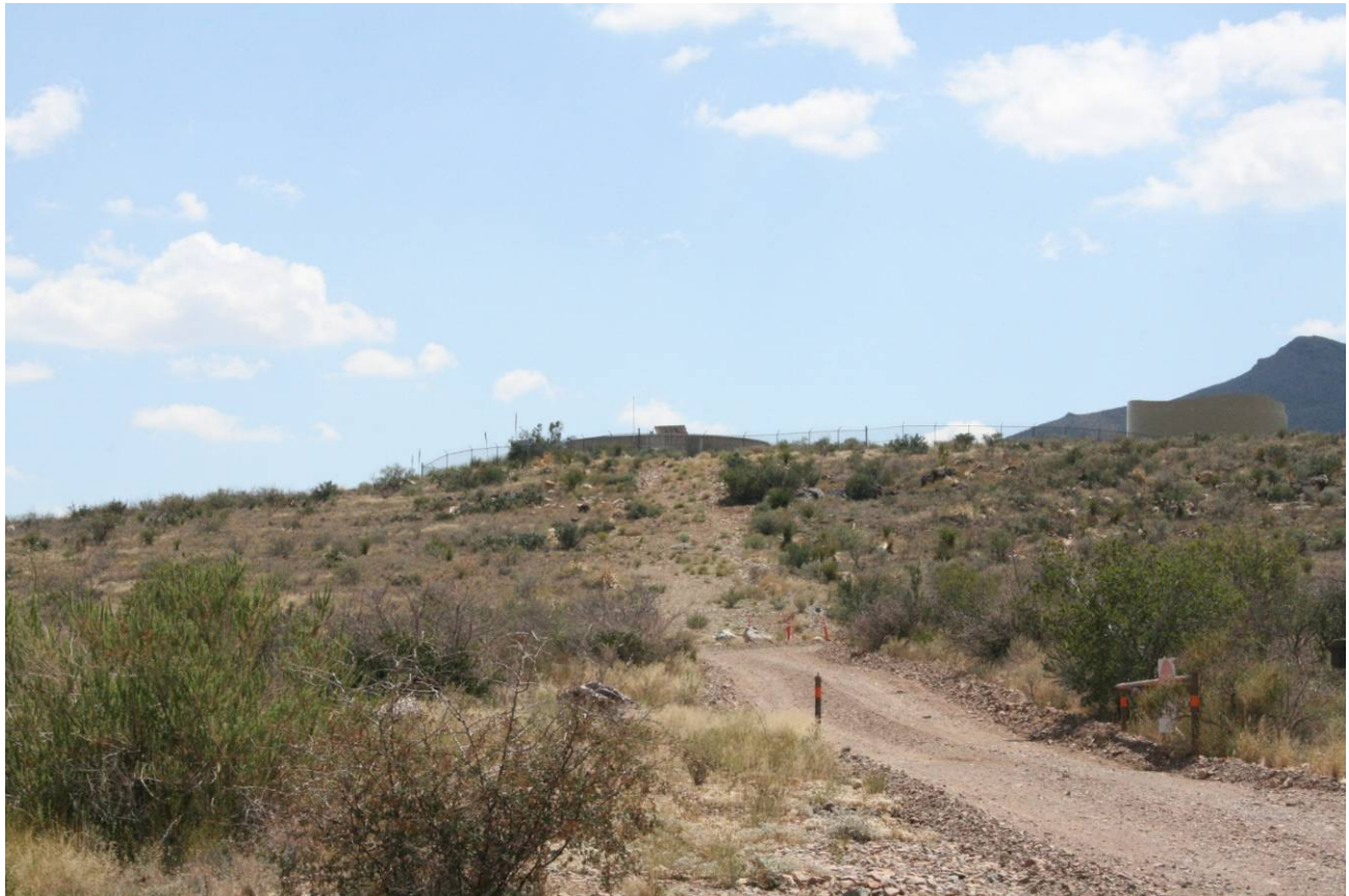
Water tank and pump house facing south
