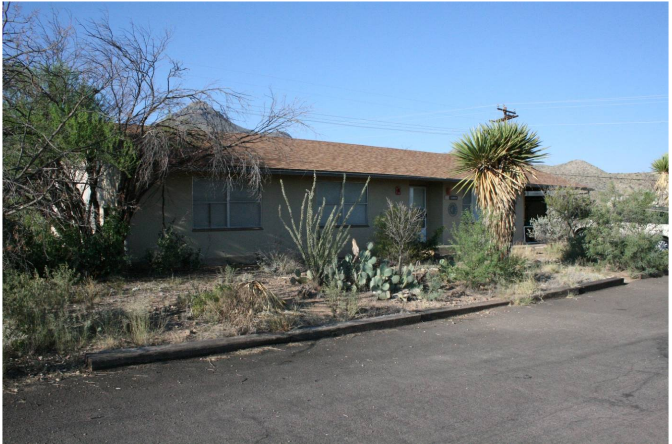
Front of residence 208 (3 bedroom, 1 and 1/2 bath) facing southwest
