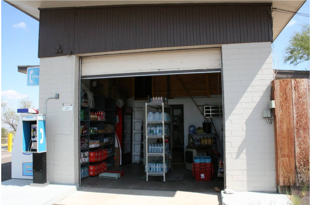
Northwest façade and maintenance bay of gas station facing southeast
