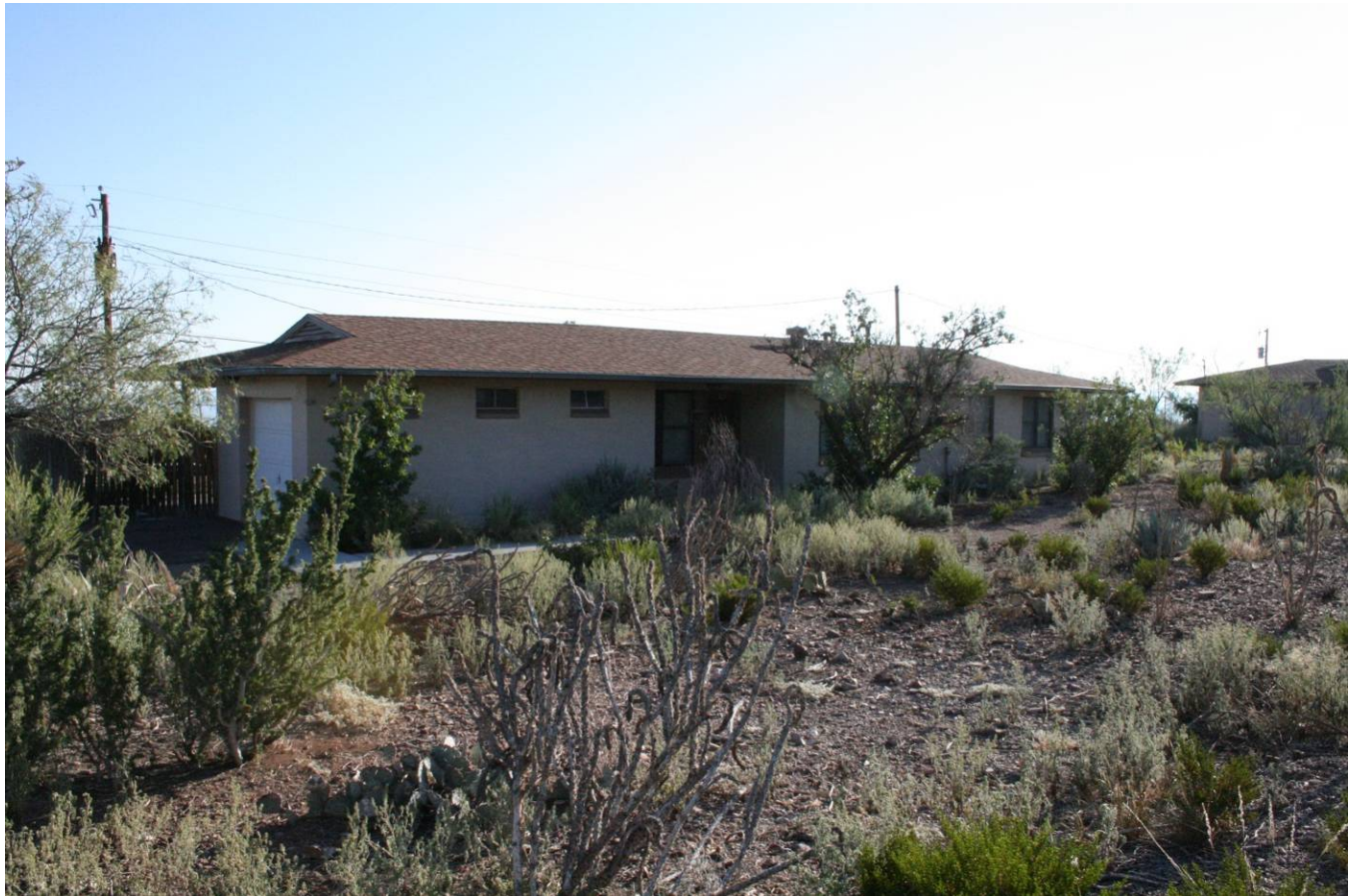
Front of residence 227 (3 bedroom, 1 bath) facing northeast
