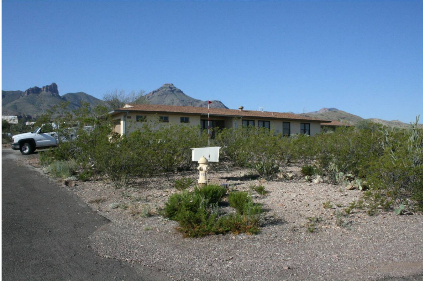
Front of residence 228 (3 bedroom, 1 bath) facing southeast
