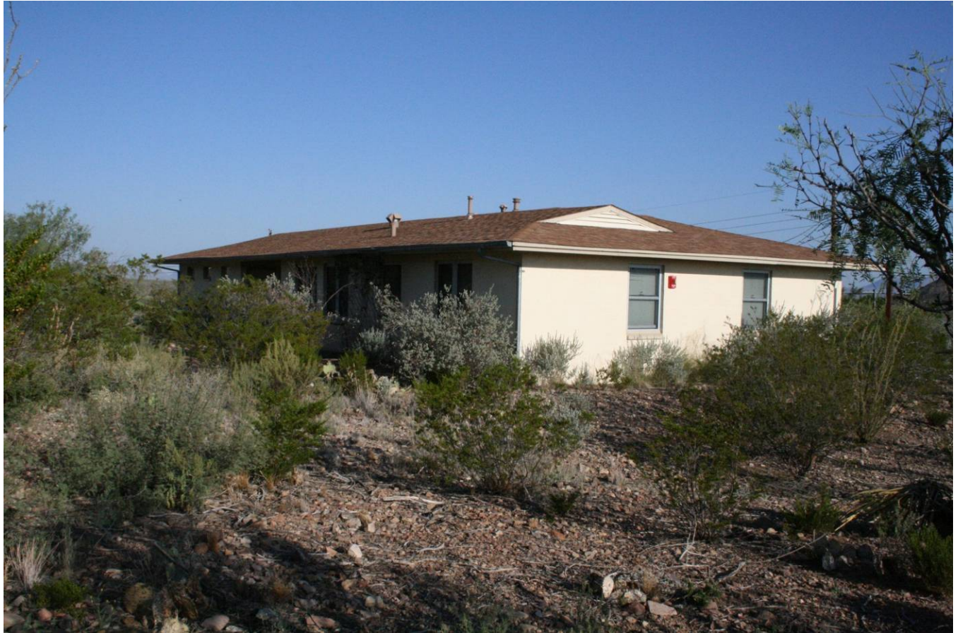
Front of residence 223 (3 bedroom, 1 bath) facing northwest
