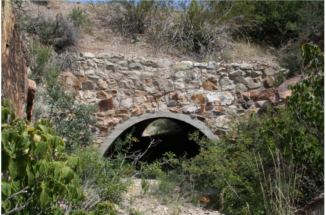
Stone-faced culvert under Alsate Drive facing northeast
