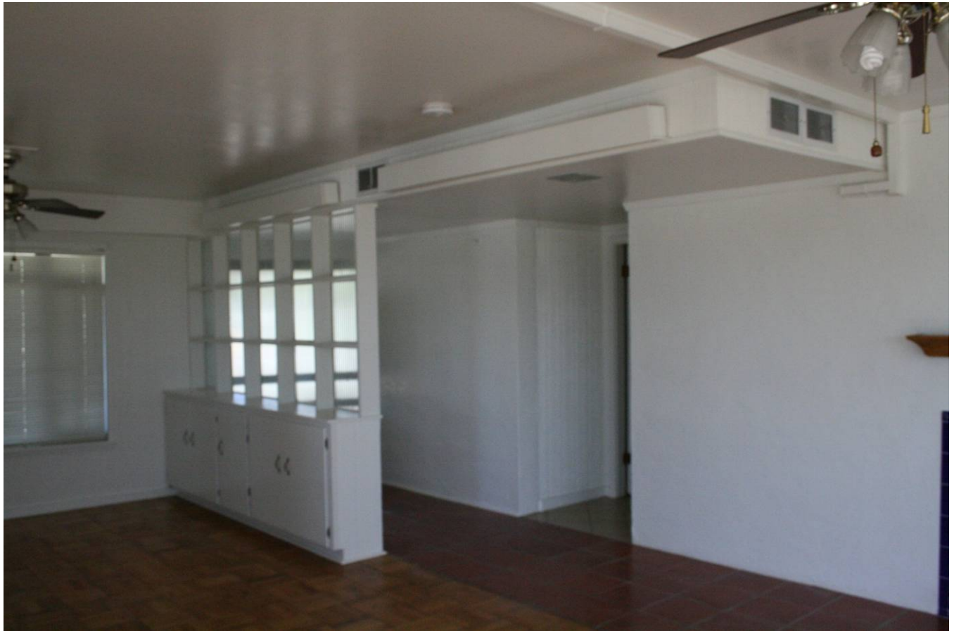
Superintendent's living room facing southwest
