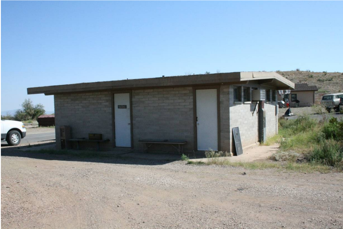
West and south façades of laundry/shower building facing northeast
