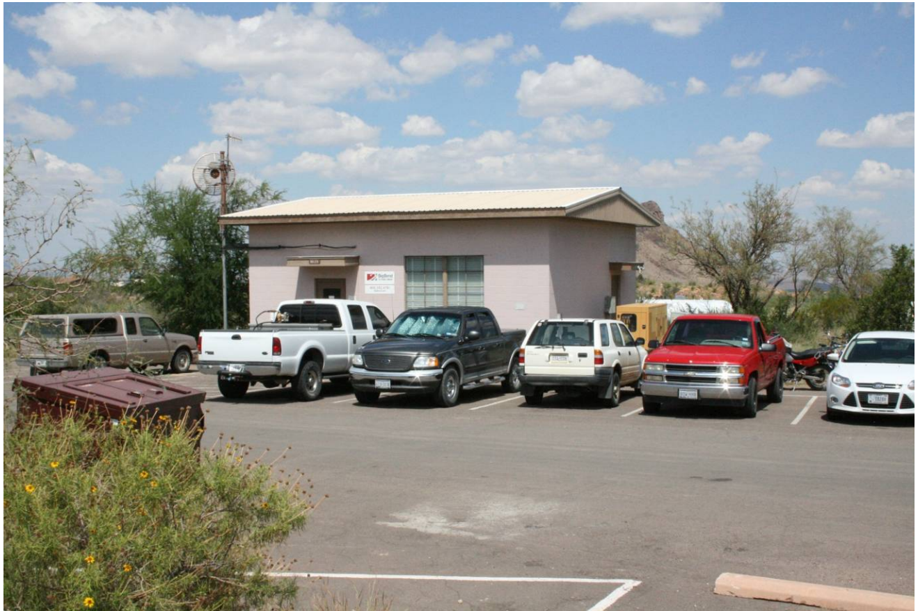
Telephone exchange building (271) facing northeast
