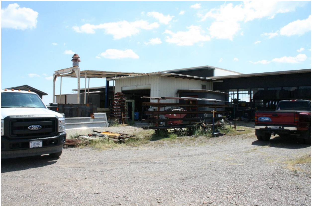
Northeast (back) façade of maintenance building facing southeast
