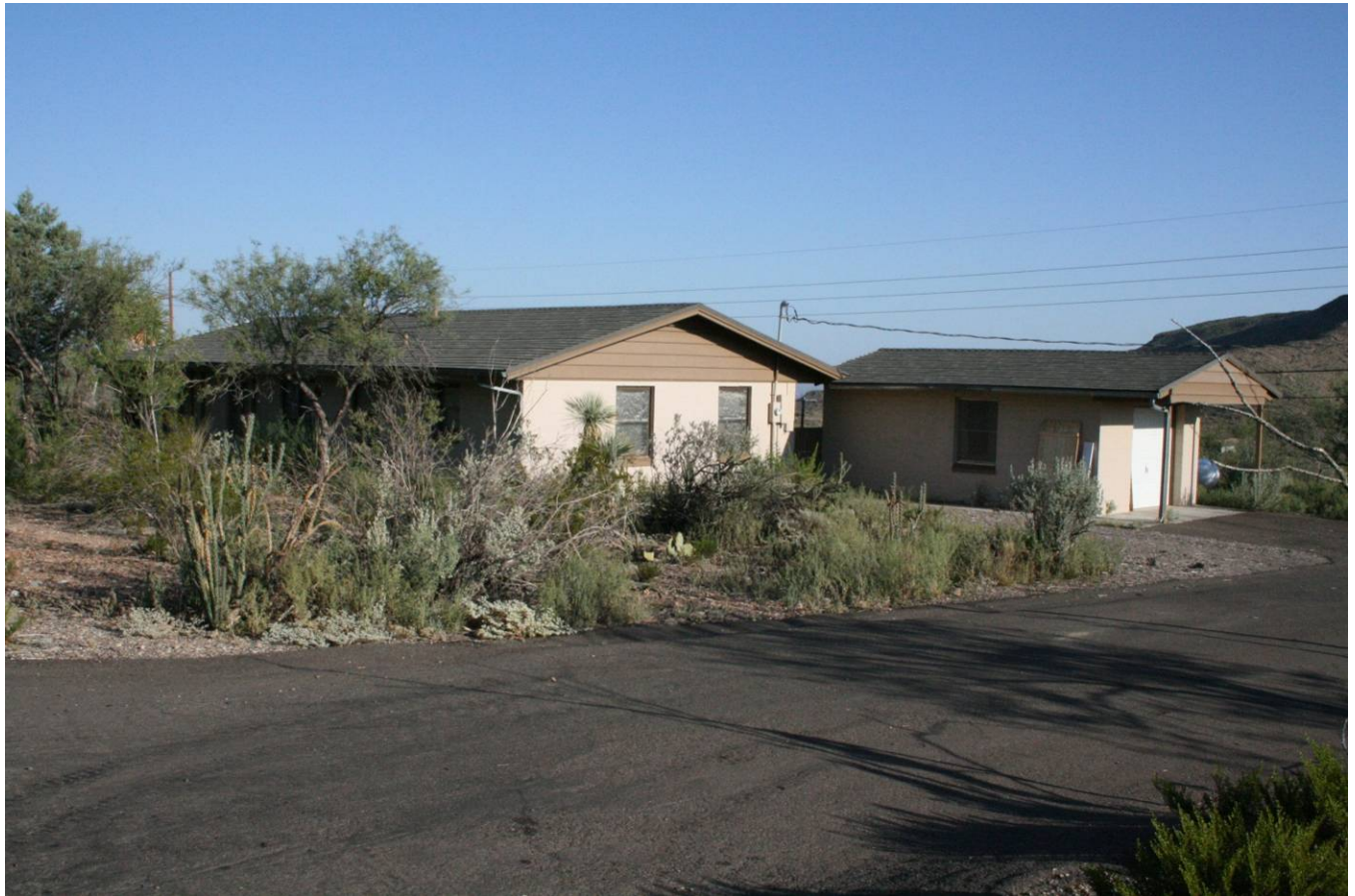
Front of residence 225 (2 bedroom, 1 bath) facing northwest
