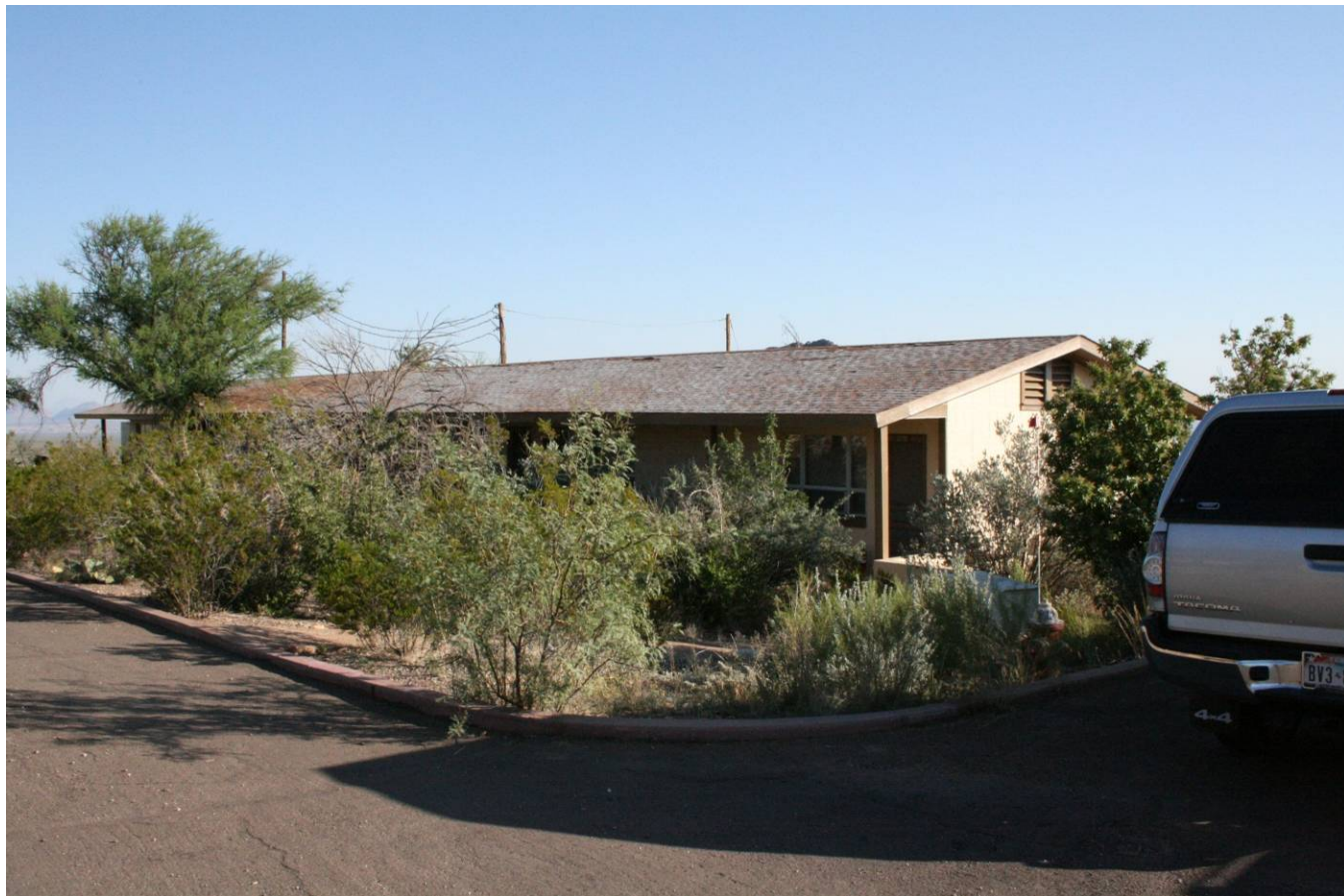
Front of apartment 217 facing north
