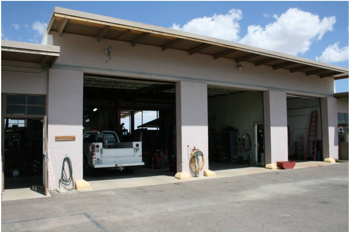
Front façade high bays of maintenance building facing northeast
