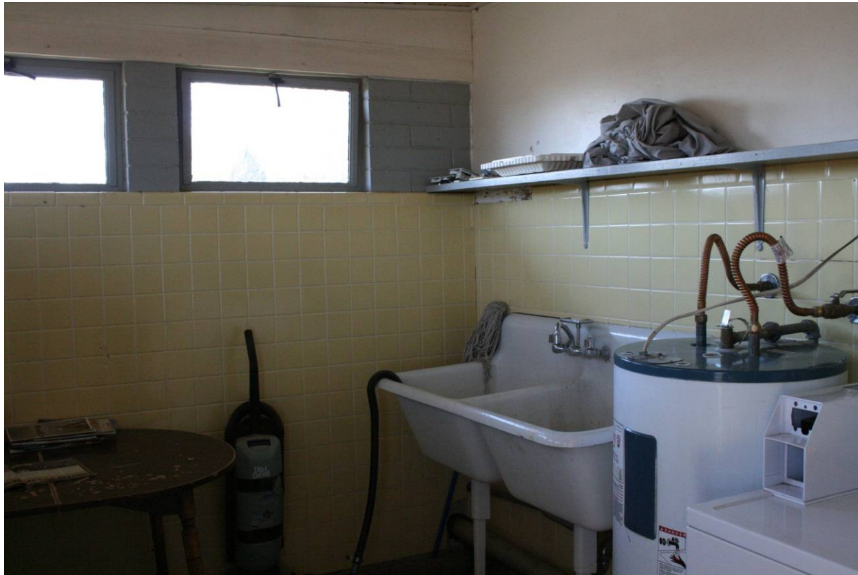
Interior of laundry building facing south
