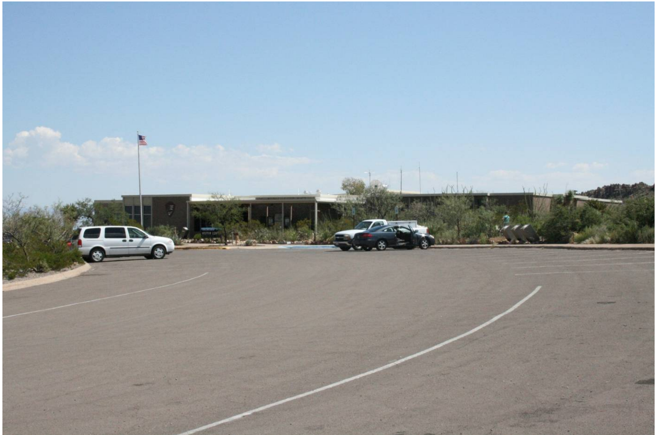
Visitor center parking lot facing southeast
