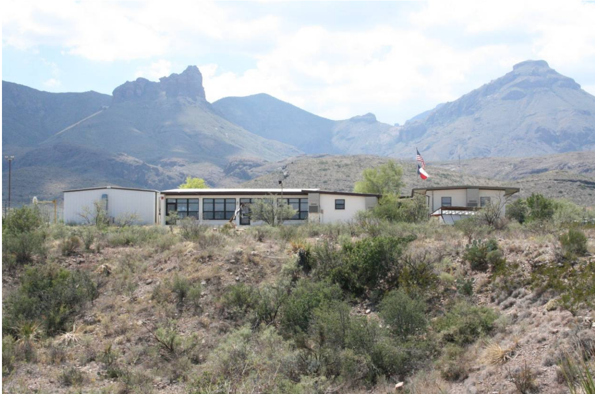
Northeast façade of school facing southwest
