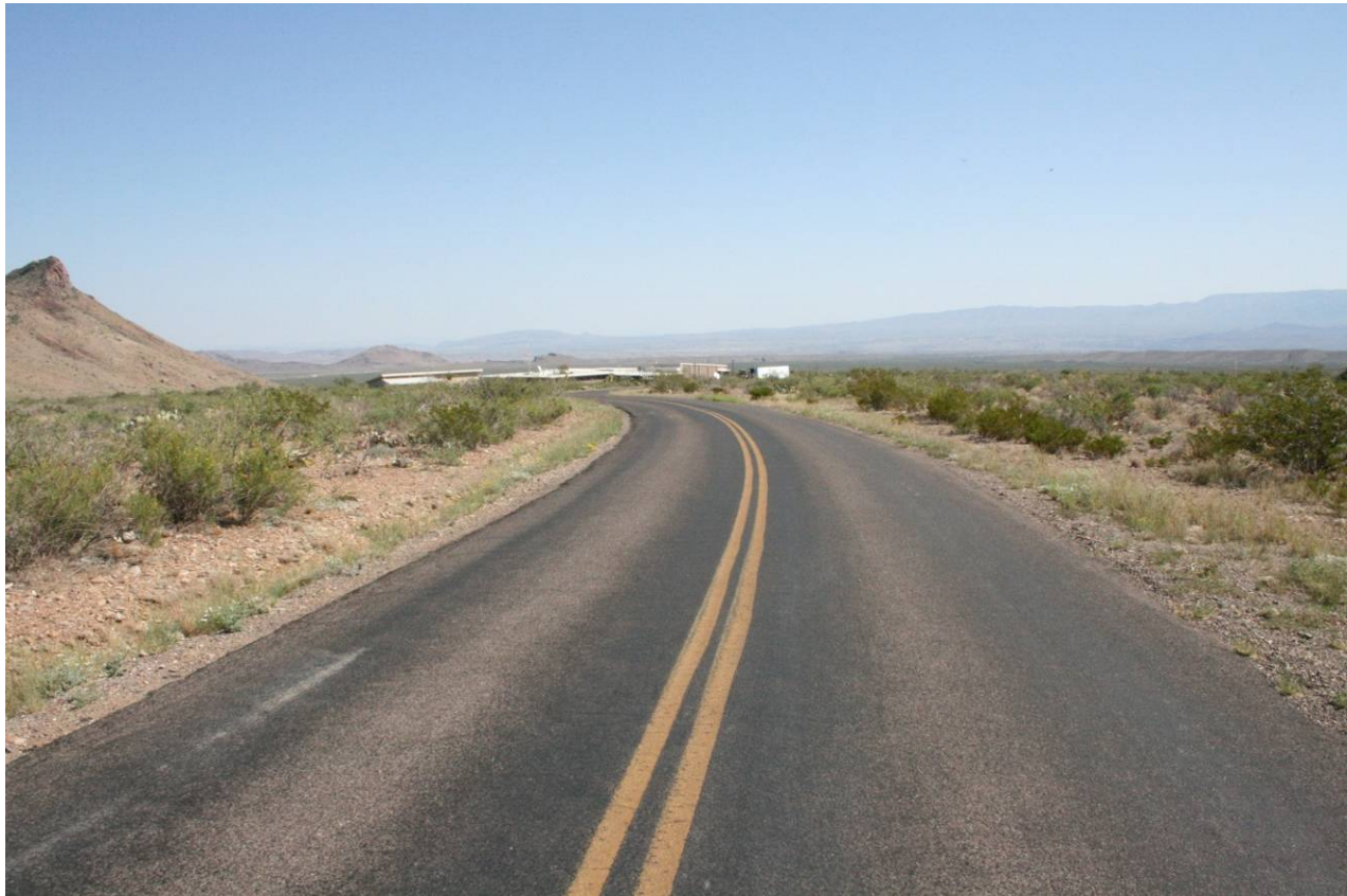
Alsate Road from residential area toward administration building facing northeast
