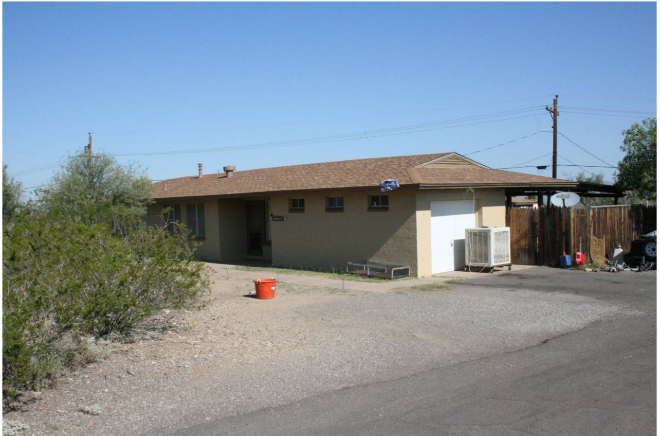
Front of residence 237 (3 bedroom, 1 bath) facing northwest
