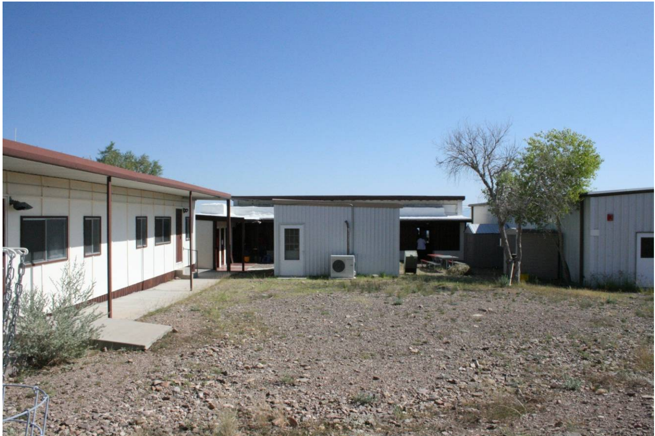
Southwest façade of school (hidden by infill) facing northeast
