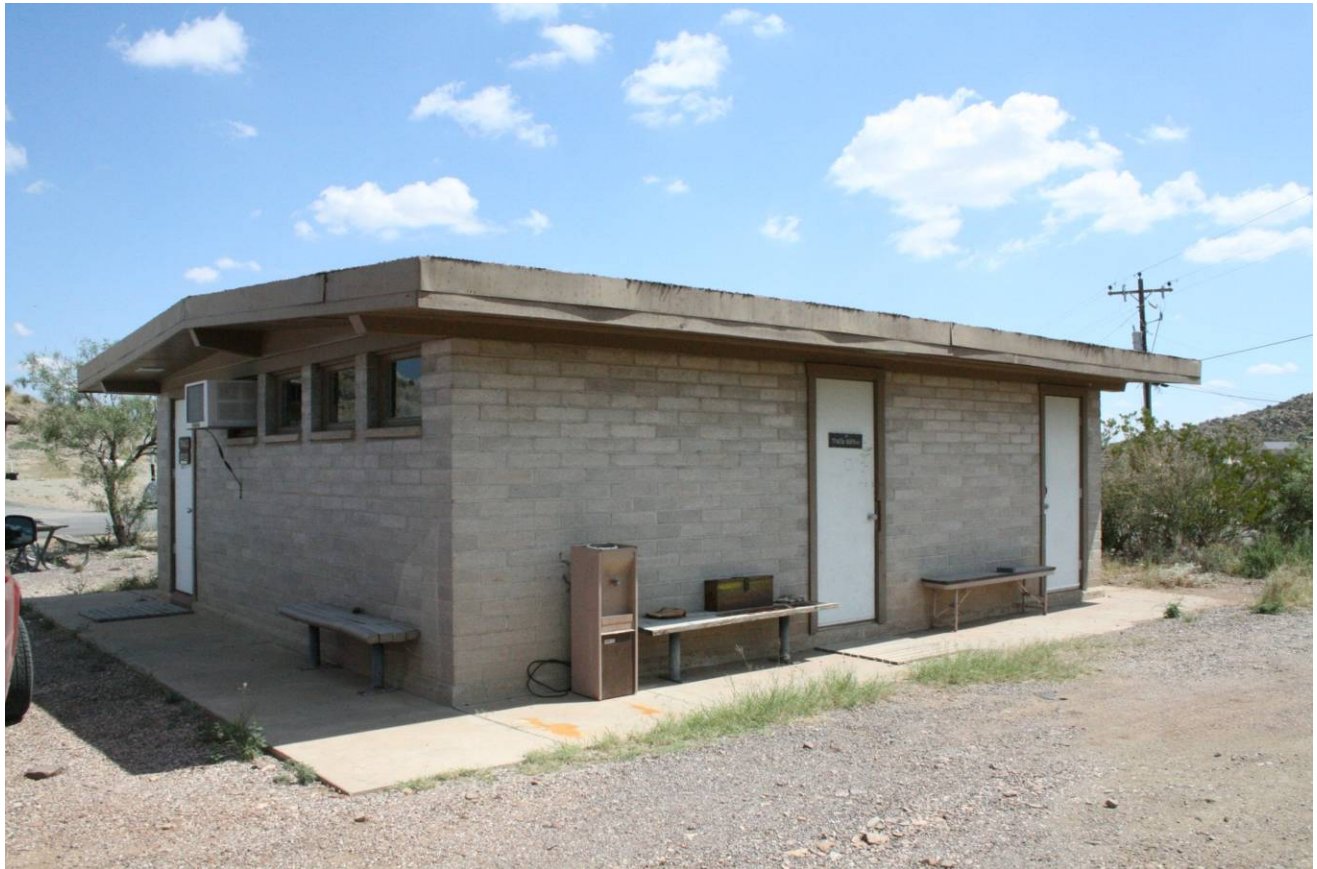
West and north façades of laundry/shower building facing southeast
