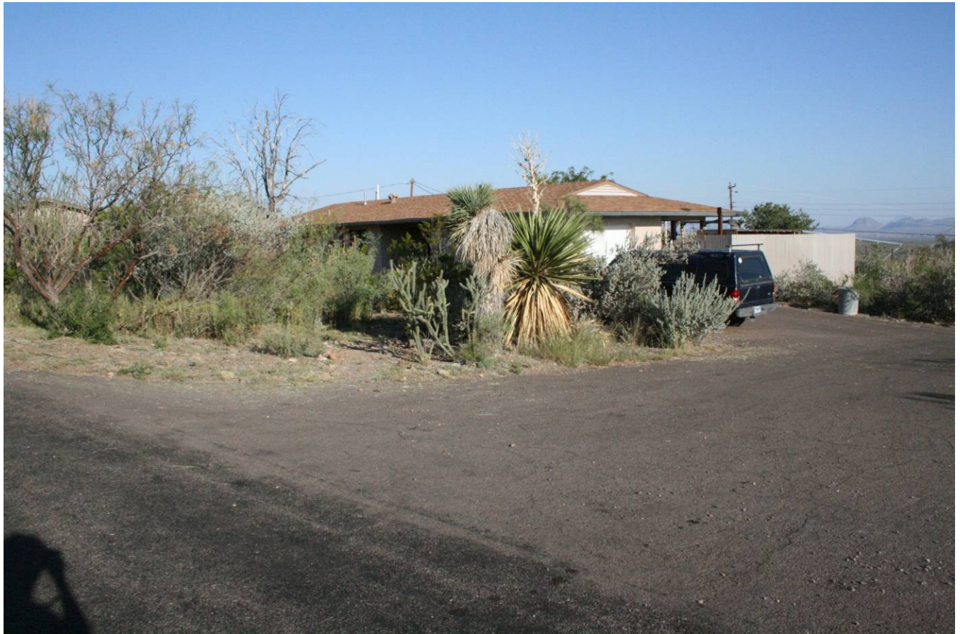
Front of residence 319 (3 bedroom, 1 bath) facing northwest
