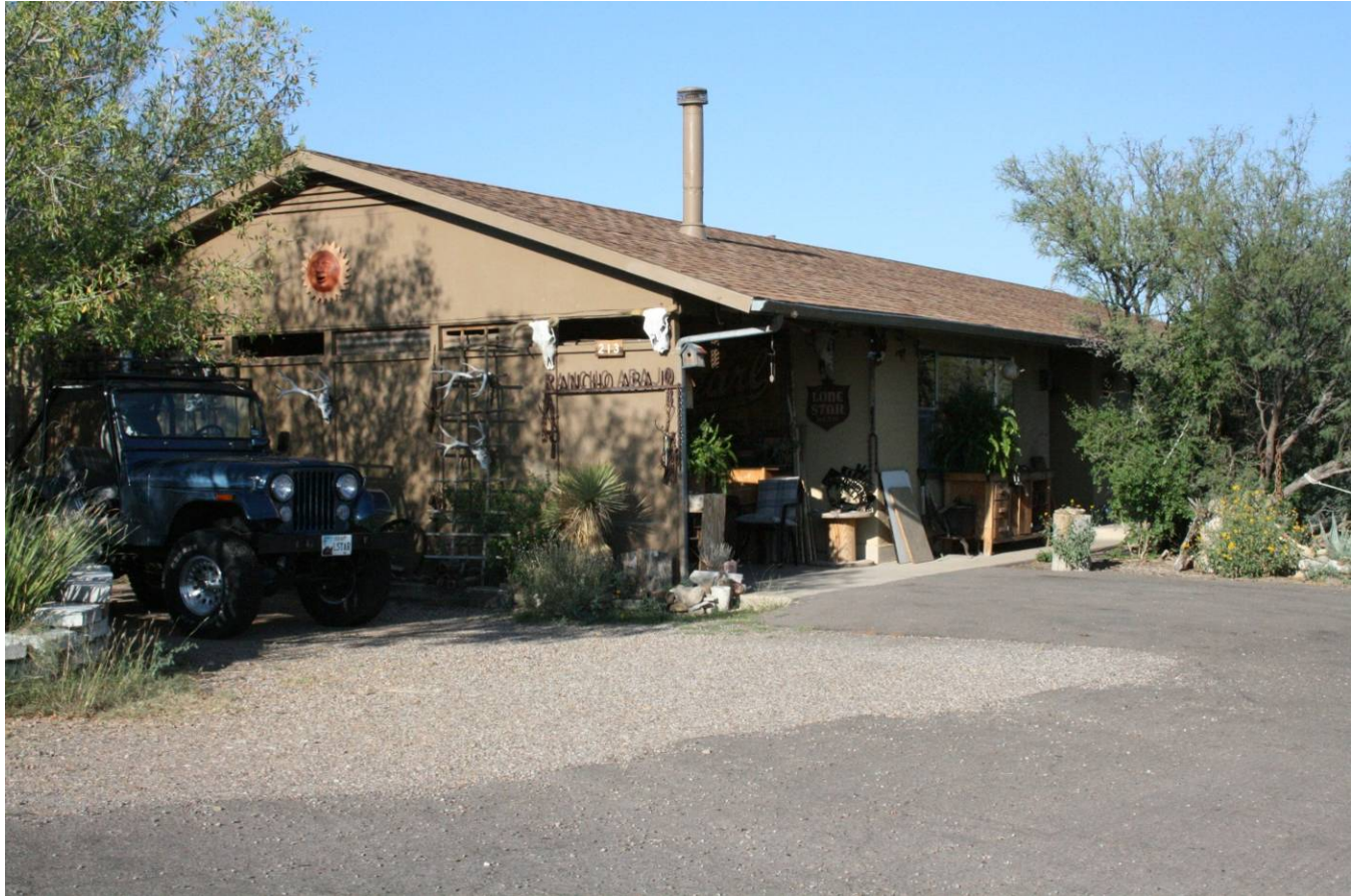
Front of residence 213 (3 bedroom, 1 and 1/2 bath) facing southwest
