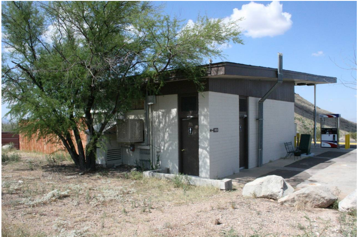
South and east façades of gas station facing north
