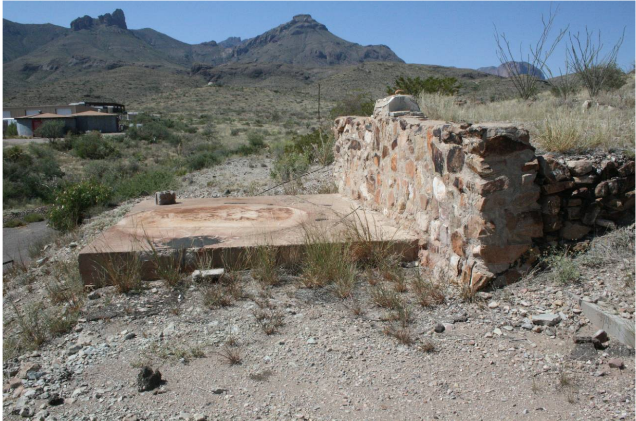
Stone Oil Tank pad in maintenance storage area (contributing landscape feature), looking southwest
