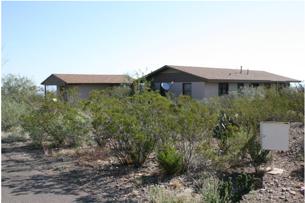
Front of residence 235 (2 bedroom, 1 bath) facing northeast
