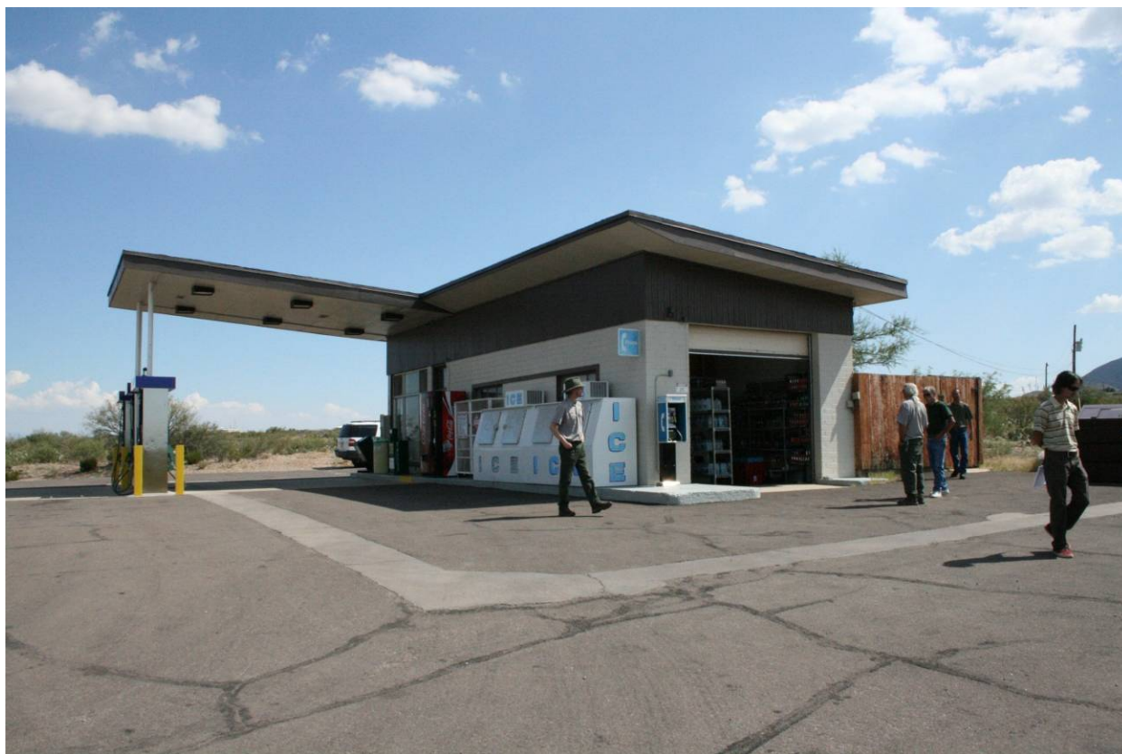
North and west façades of gas station facing southeast
