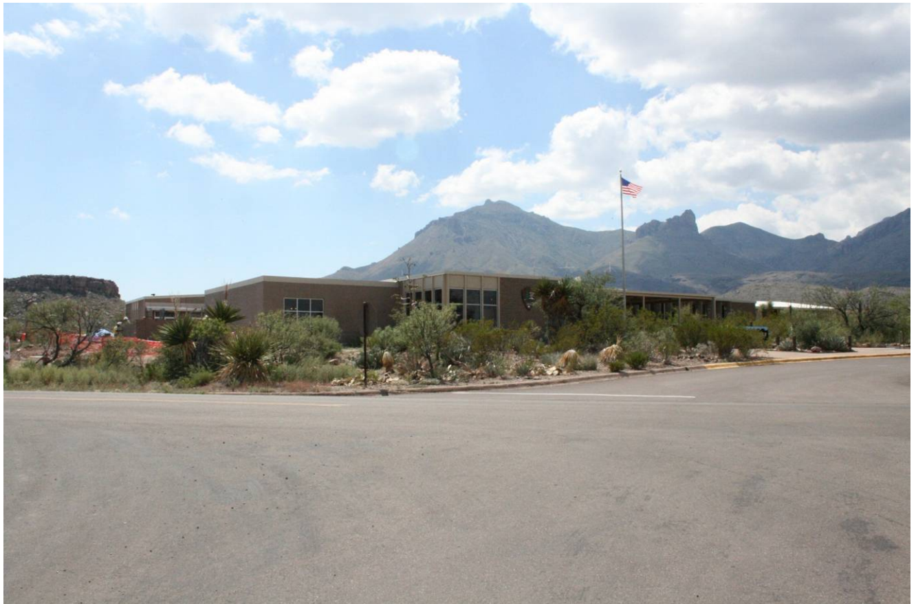
Front and northeast façades of visitor center and administration building facing southwest
