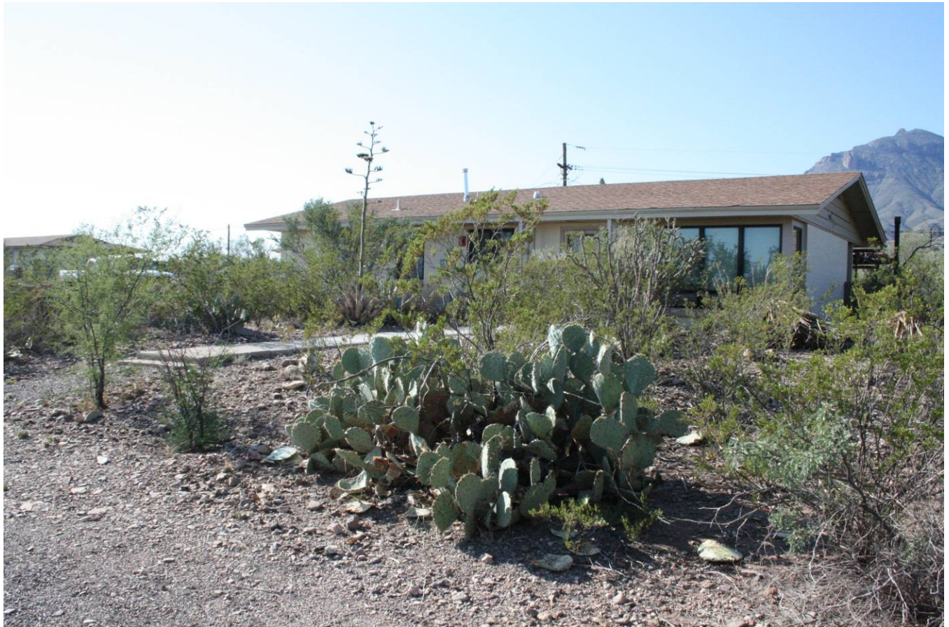
Front of residence 250 (2 bedroom, 1 bath) facing southeast
