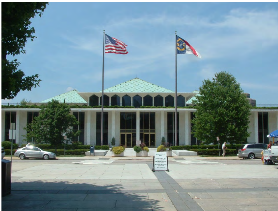
Figure 9: The exterior of the Stuhr Museum borrows heavily from Edward Stone's 1960 North Carolina State Legislature Building, including the use of vertical window bands, concrete columns, and pyramidal domes. (Wikimedia Commons)
