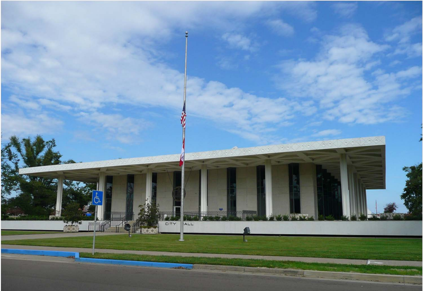
Figure 11: Paducah City Hall. The building shares a very similar plan and details to the Stuhr Museum. Differences include a triangular pattern waffle slab roof, projecting windows, and a larger pyramidal dome (not visible). (Flickr, army.arch, 2009)
