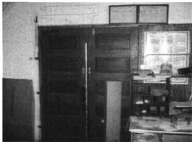
Original Five-Paneled Wood Doors
