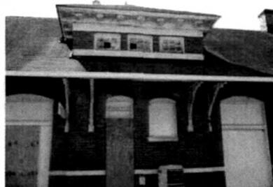
West Façade Detail
