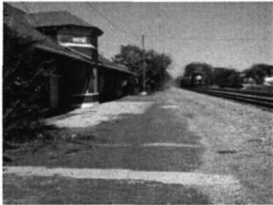
Brick Platform (rear elevation)
