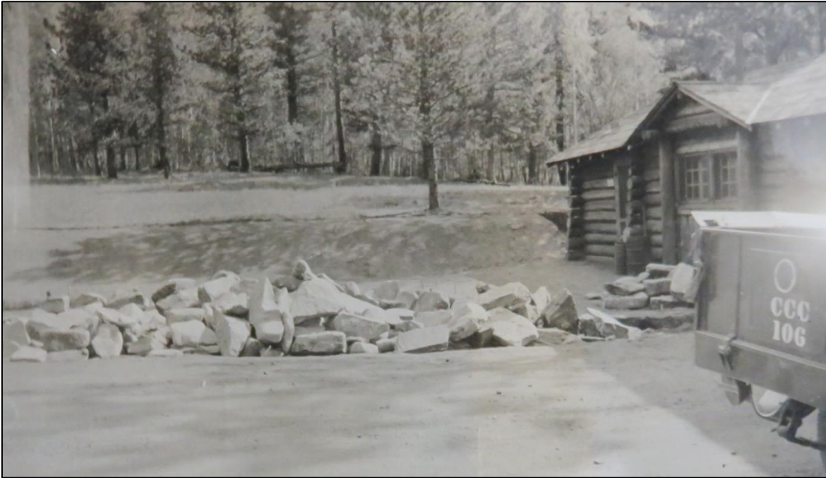
H5. June 1934 view of rocks for masonry curbing at the Fall River Entrance, by Roy Youngs. Located in the files of Rocky Mountain National Park Archives, Estes Park, Colorado, Civilian Conservation Corps Photograph Albums, photograph no. 3575.
