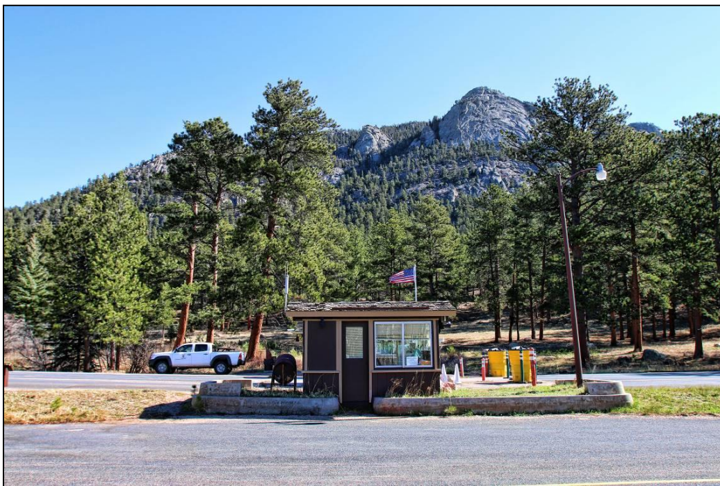
Photograph 6. Overview of the checking station (Building 353) and kiosks (Buildings 669-671) from the outbound lane with McGregor Mountain in the background, facing northeast.
