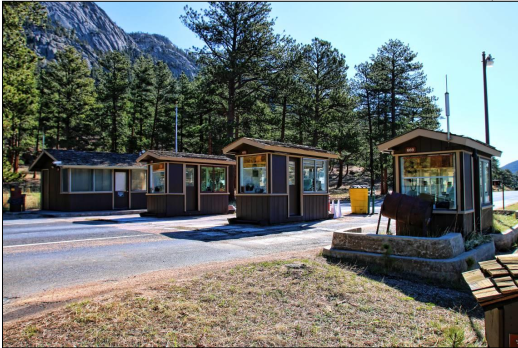
Photograph 5. View of the checking station (Building 353) and kiosks (Buildings 669-671) from the outbound lane, facing east-northeast.
