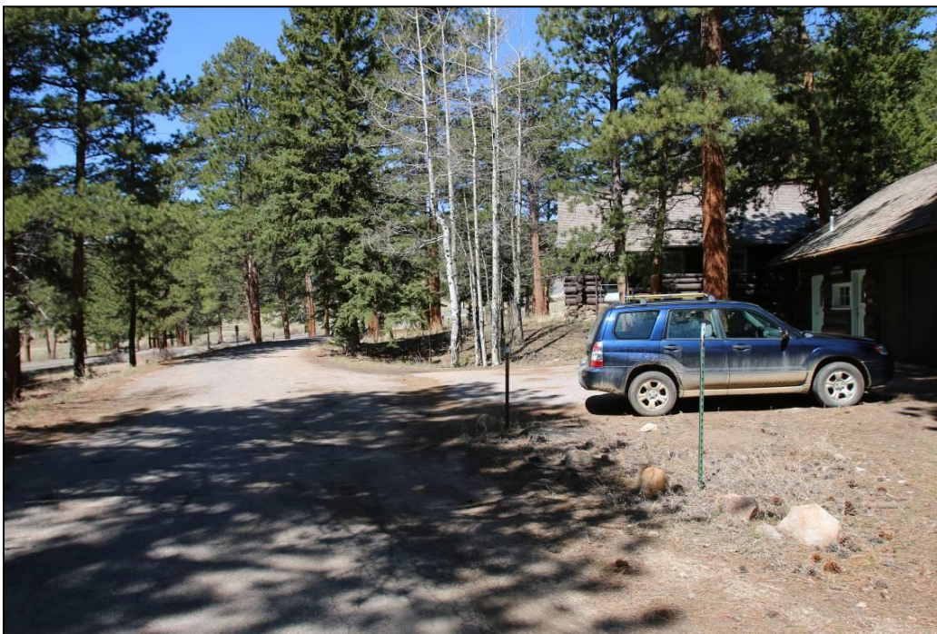
Photograph 14. Overview of the Bighorn Ranger Station Area access road, facing west-northwest.
