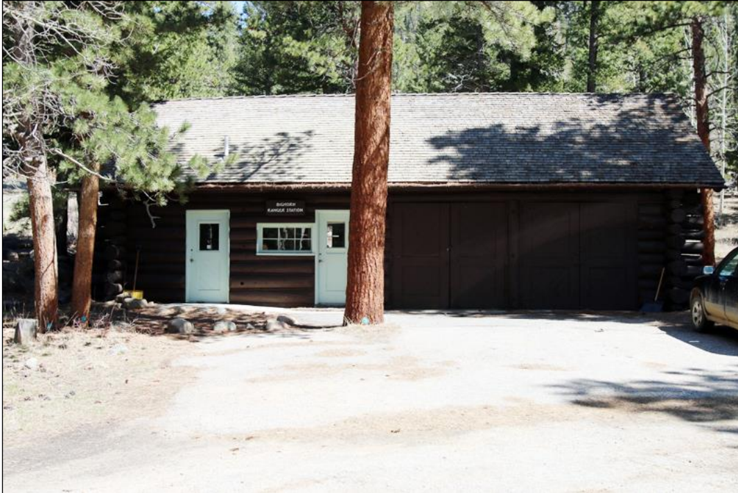
Photograph 21. Façade of the garage and woodshed (Building 169), facing northeast.
