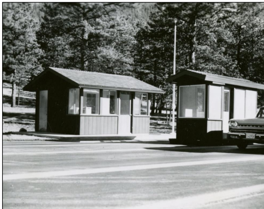
H14. December 1960 view of the checking station and kiosks at the redeveloped Fall River Entrance, by R.H. Boyer. Located in the files of Rocky Mountain National Park Archives, Estes Park, Colorado, Photograph Collection (11-Q-7), album no. 1, photograph no. 1374.
