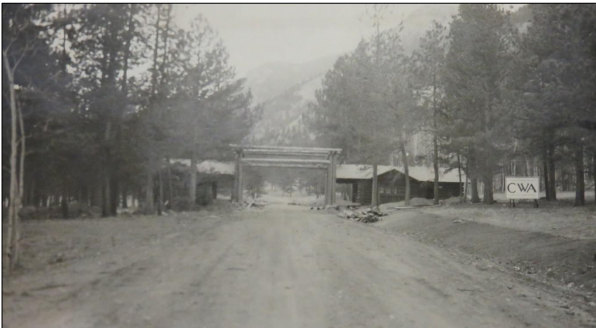
H6. March 1934 view of the relocation of the Fall River Entrance, by Dorr G. Yeager. Located in the files of Rocky Mountain National Park Archives, Estes Park, Colorado, Civilian Conservation Corps Photograph Albums, photograph no. 3279.
