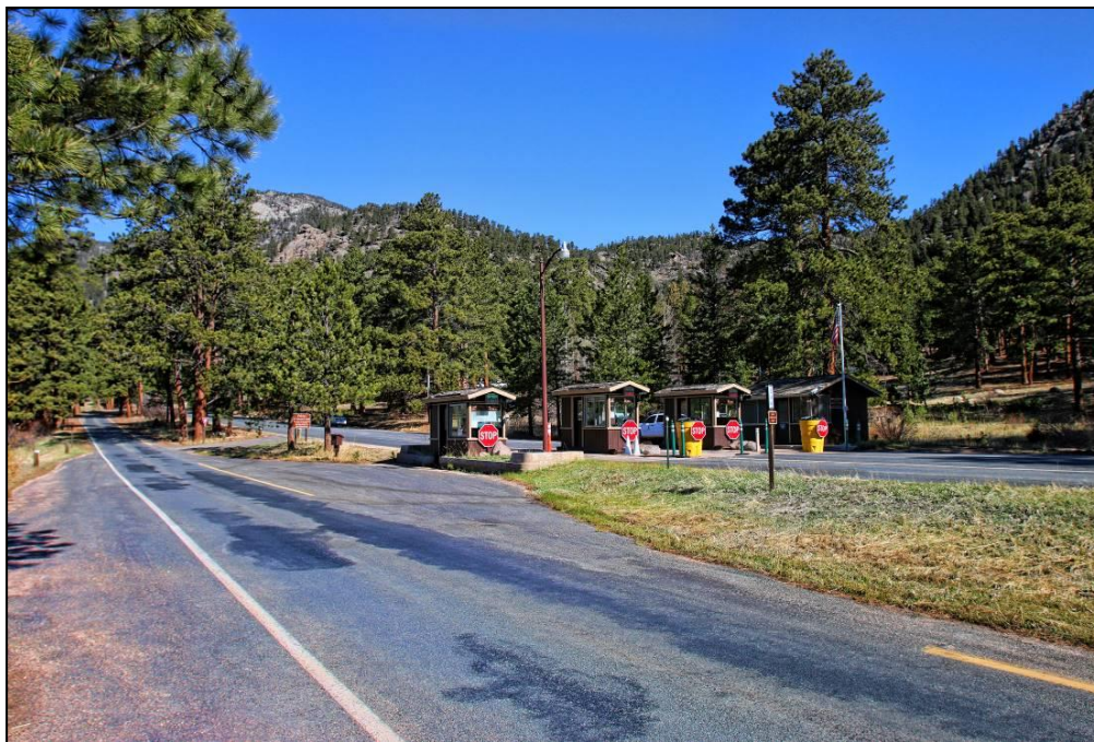
Photograph 4. View of the checking station (Building 353) and kiosks (Buildings 669-671) from the outbound lane, facing north-northwest.
