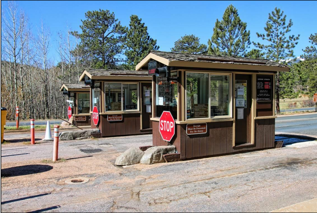
Photograph 7. Close-up of the entrance kiosks (Buildings 669-671), facing southwest.
