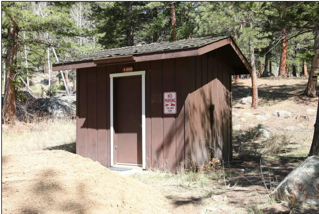
Photograph 22. Oblique view of the pump house (Building 869), facing northwest.
