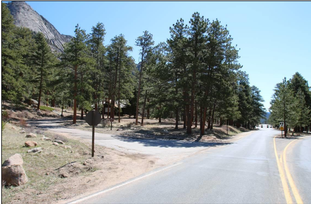
Photograph 13. Overview of the intersection of U.S. 34/Fall River Road and the Bighorn Ranger Station Area access road, facing northeast.
