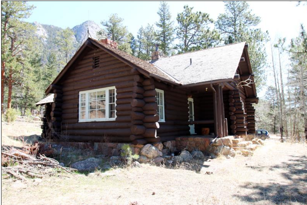
Photograph 15. Oblique view of the Bighorn Ranger Station (Building 44), facing northeast.
