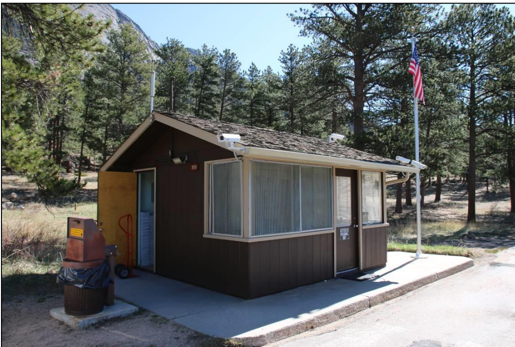
Photograph 8. Oblique view of the checking station (Building 353), facing east-northeast.
