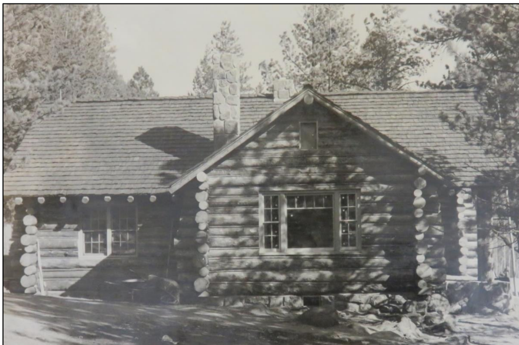
H8. March 1935 view of the Bighorn Ranger Station (Building 44). Located in the files of Rocky Mountain National Park Archives, Estes Park, Colorado, Civilian Conservation Corps Photograph Albums, photograph no. 3376.
