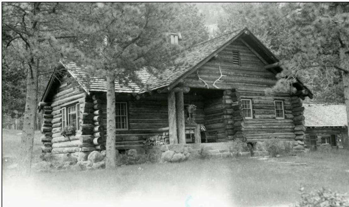
H16. Undated, c. 1960, view of the Bighorn Ranger Station (Building 44), by Ferrel Atkins. Located in the files of Rocky Mountain National Park Archives, Estes Park, Colorado, Ferrel Atkins Collection, Building Folder No. 44.
