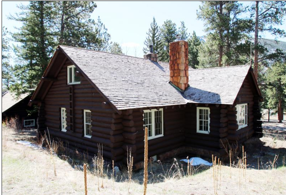
Photograph 17. Oblique view of the Bighorn Ranger Station (Building 44), facing south-southeast.
