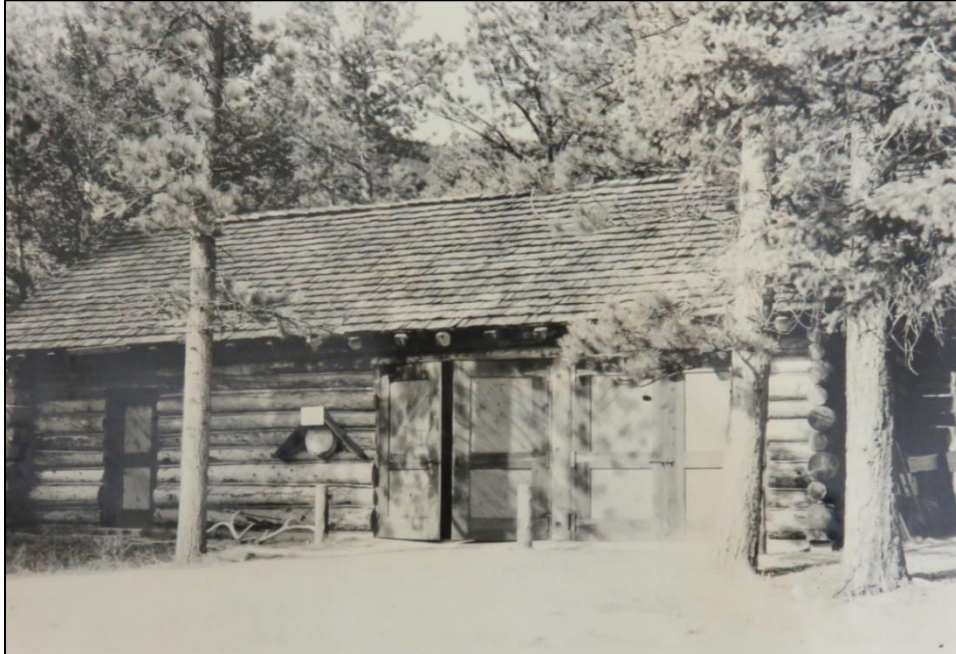
H9. March 1935 view of the garage and wood shed (Building 169). Located in the files of Rocky Mountain National Park Archives, Estes Park, Colorado, Civilian Conservation Corps Photograph Albums, photograph no. 4715.
