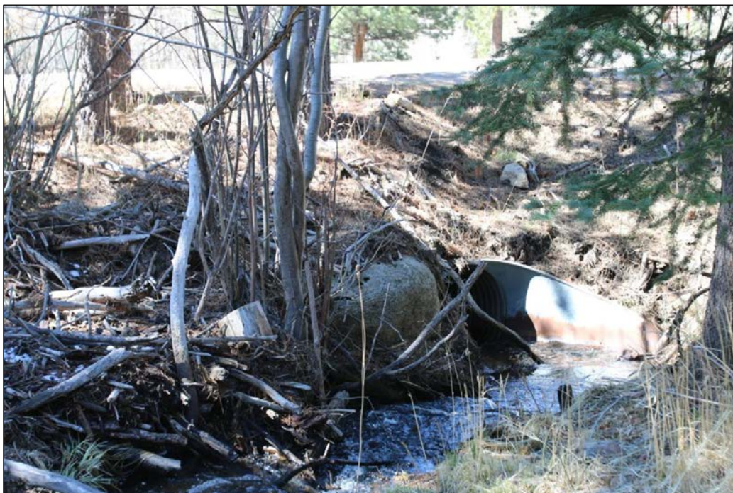
Photograph 10. Pipe culvert at Bighorn Creek north of U.S. 34, facing south.
