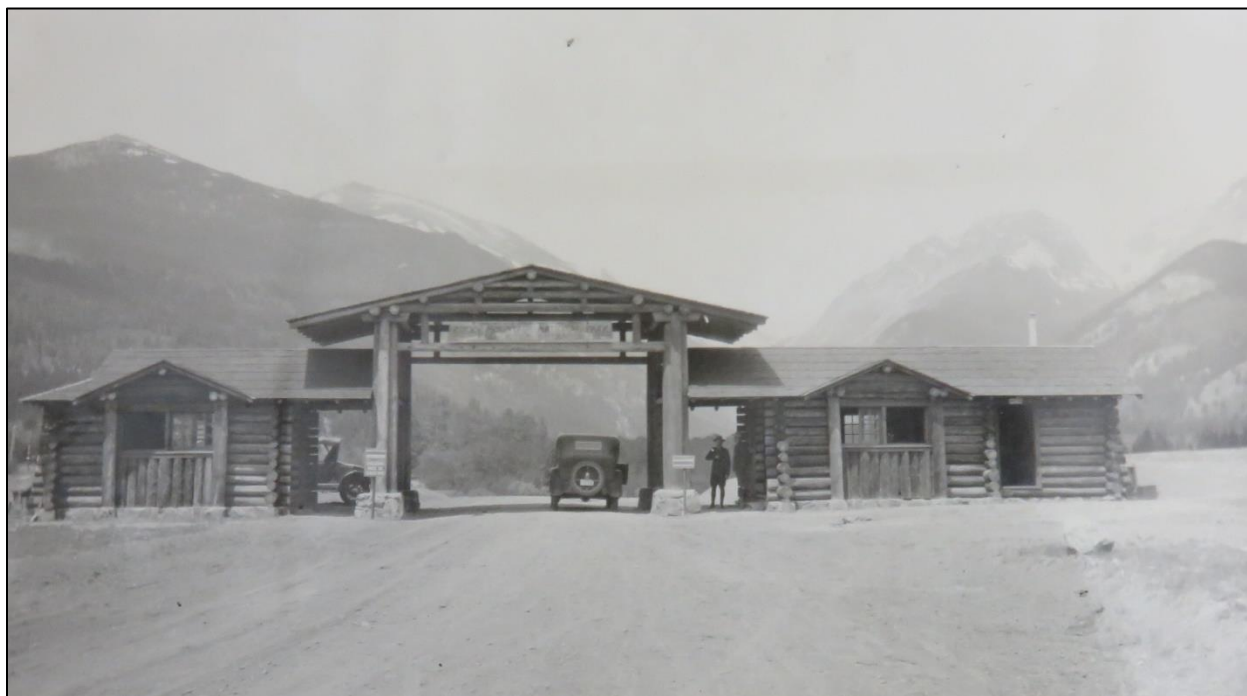
H2. 1927 view of the Fall River Entrance at Horseshoe Park, by Roger W. Toll. Located in the files of Rocky Mountain National Park Archives, Estes Park, Colorado, Civilian Conservation Corps Photograph Albums, photograph no. 879.
