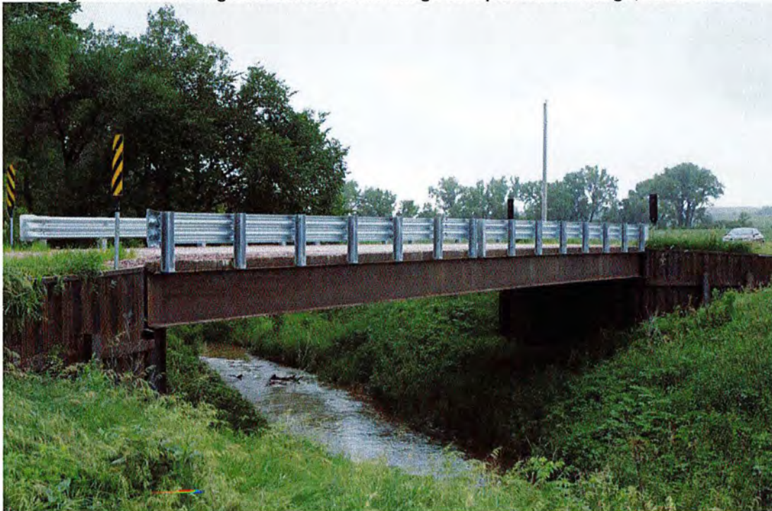
Image 2: View of metal I-beam trusses and metal railings of replacement bridge; view northwest.
