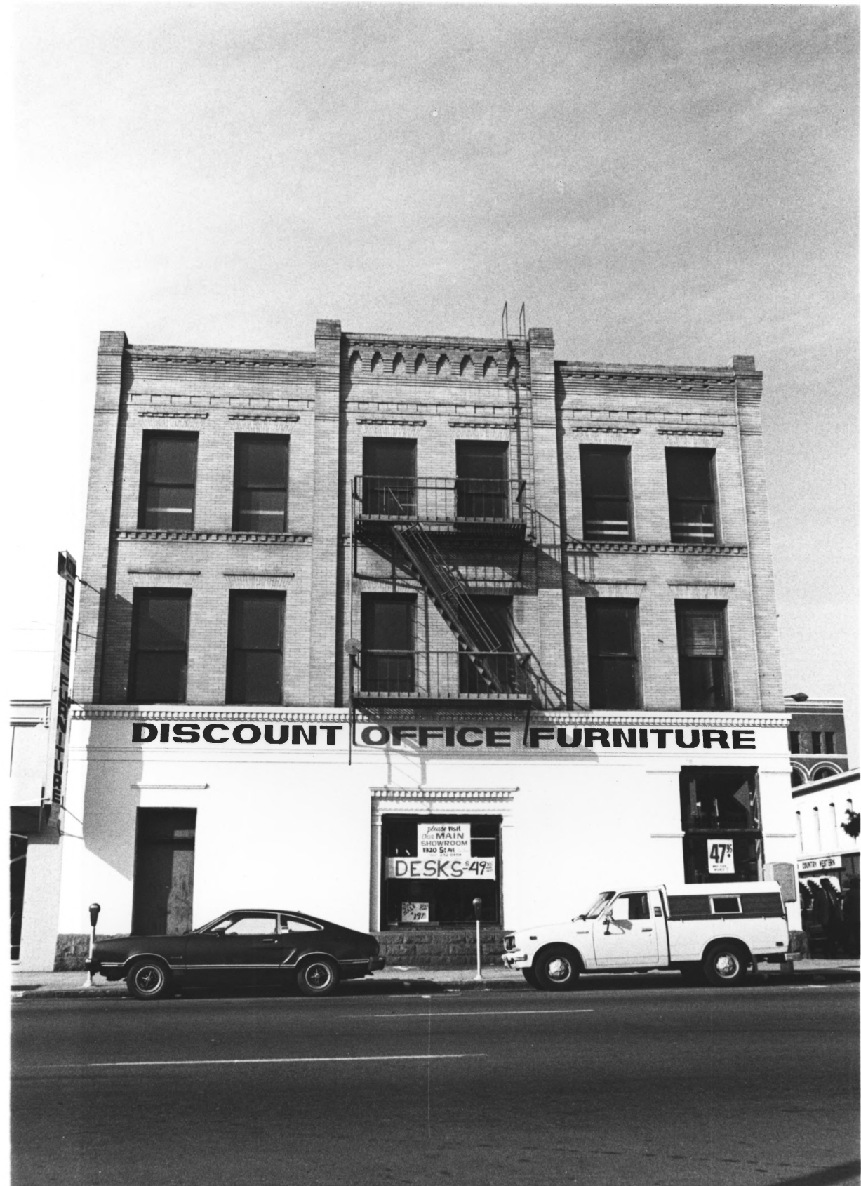
1-13. GEORGE HILL BUILDING. S.W. corner, Sixth & F.
