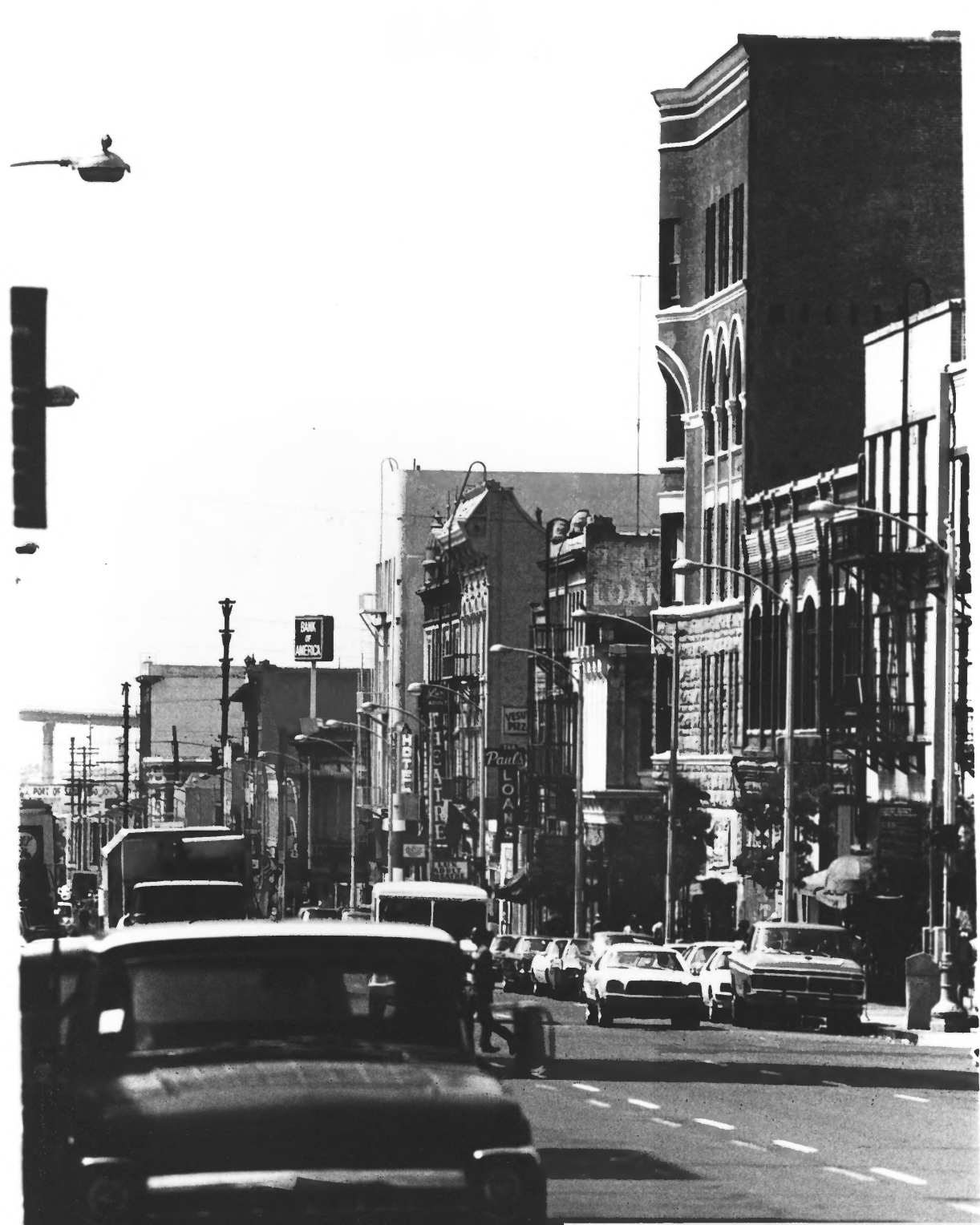
Telephoto view looking south on Fifth Avenue
