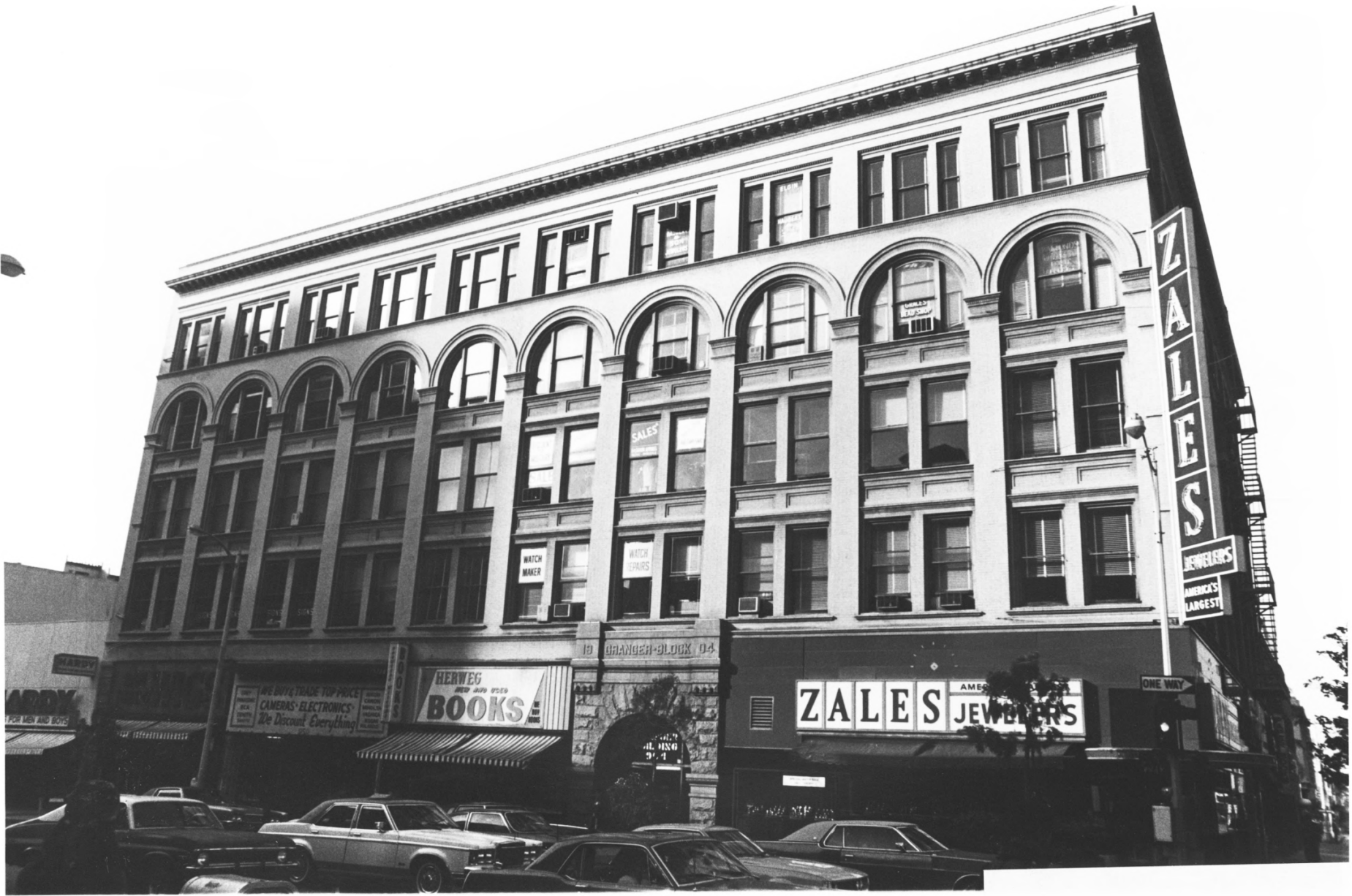
1-1. GRANGER BUILDING, SW corner Fifth Broadway.
