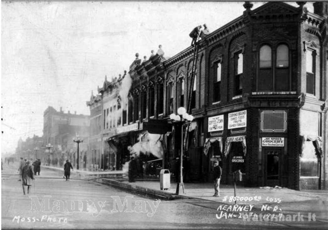
Fig 3: Central Avenue fire, 1927. Note the masonry storefront on the Low Building, which replaced the original cast iron. Maurice May Private Collection.
