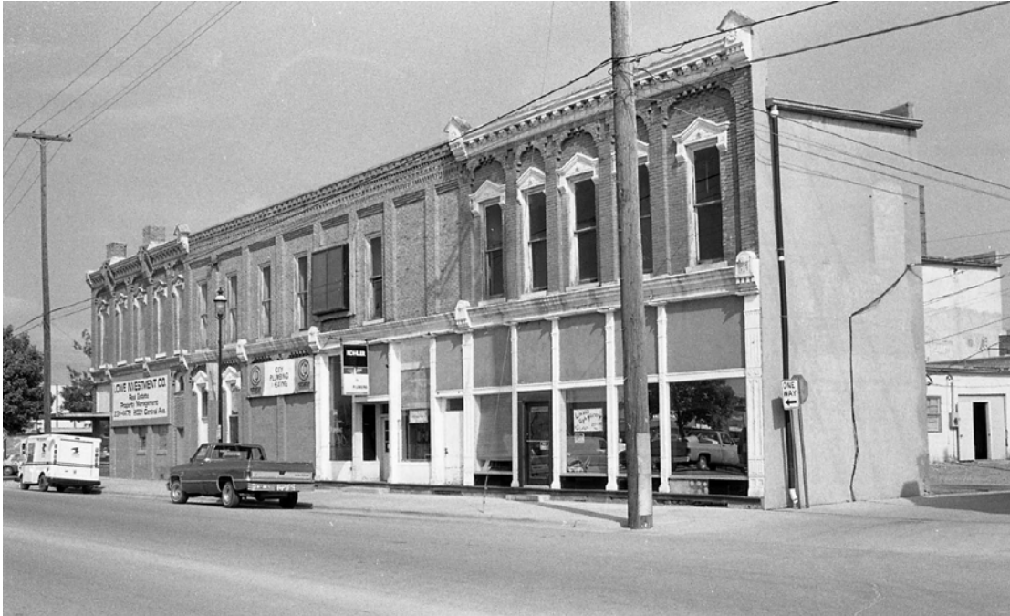
Fig. 5: City Plumbing, 1993. Robert Kay, NE Historic Building Survey.
