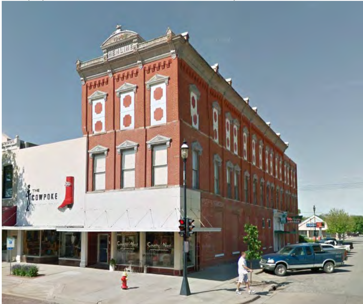
Figure 7: 1888 Henline Building, 2122 Central Ave. Google Street View, 2012.
