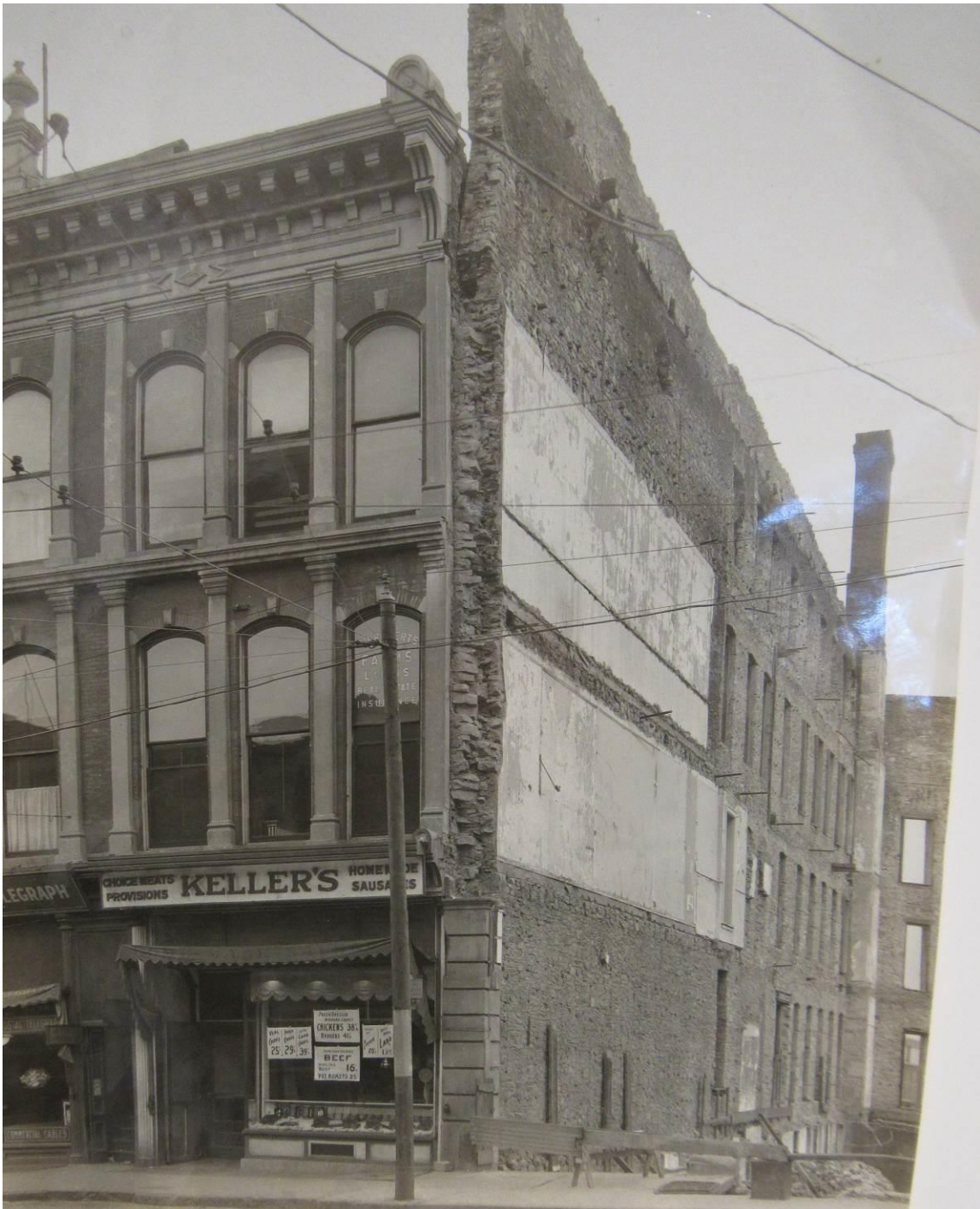
1882 Hodge Opera House (to right of photo), burned in 1928. Shows portion of exterior stone walls salvaged for re-use in the Bewley Building's construction.
