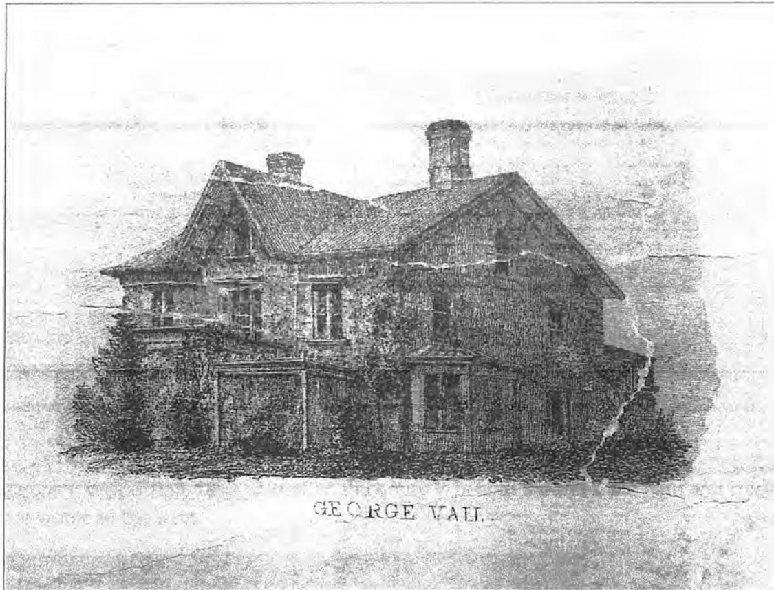
Figure 1: Willow Hall, 1850 with original three-part piazza across the front and bay window on the side elevation.
