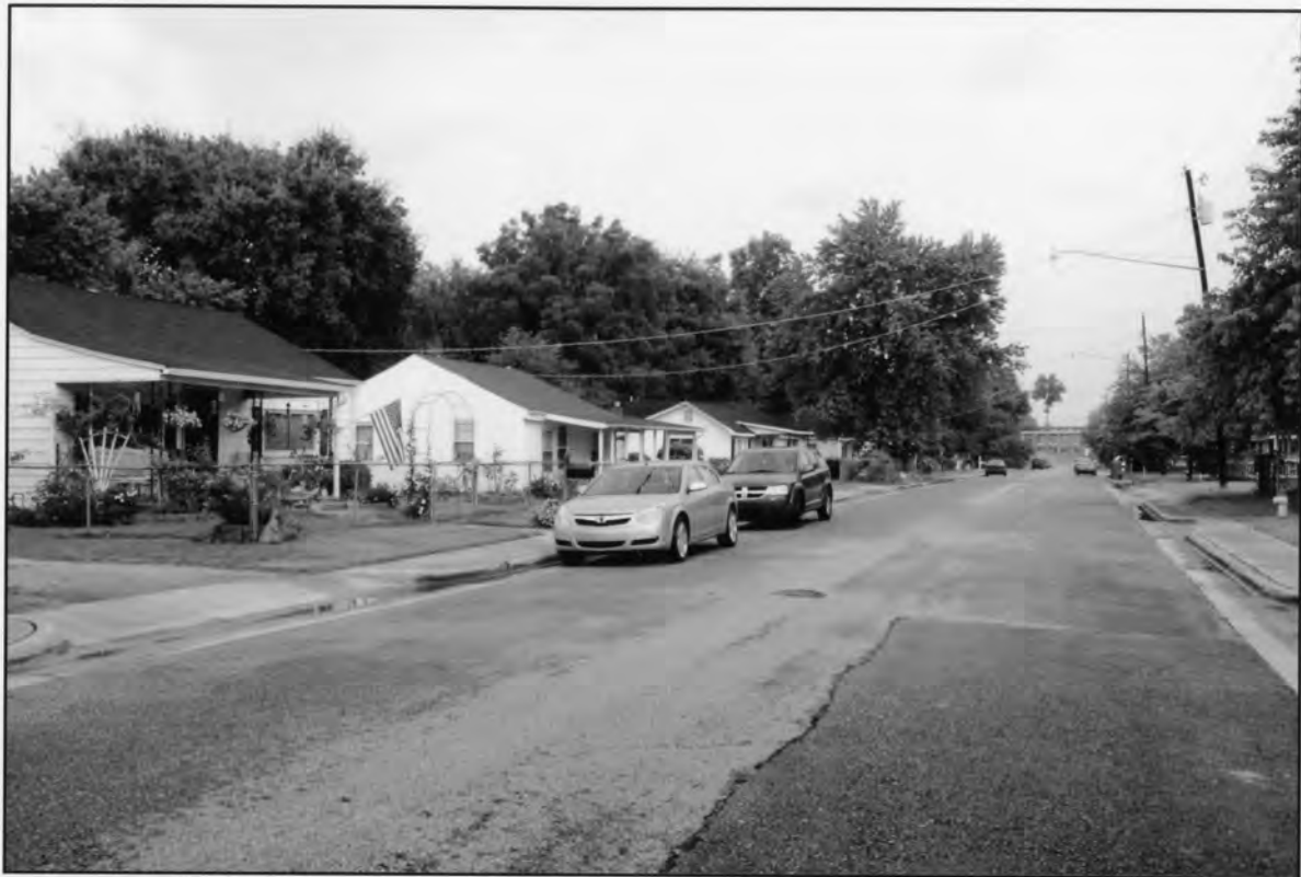
Lowe Mill and Mill Village Historic District Huntsville, Madison County, AL David B. Schneider December 2010 411 E. 6th St., Anniston AL 36207
