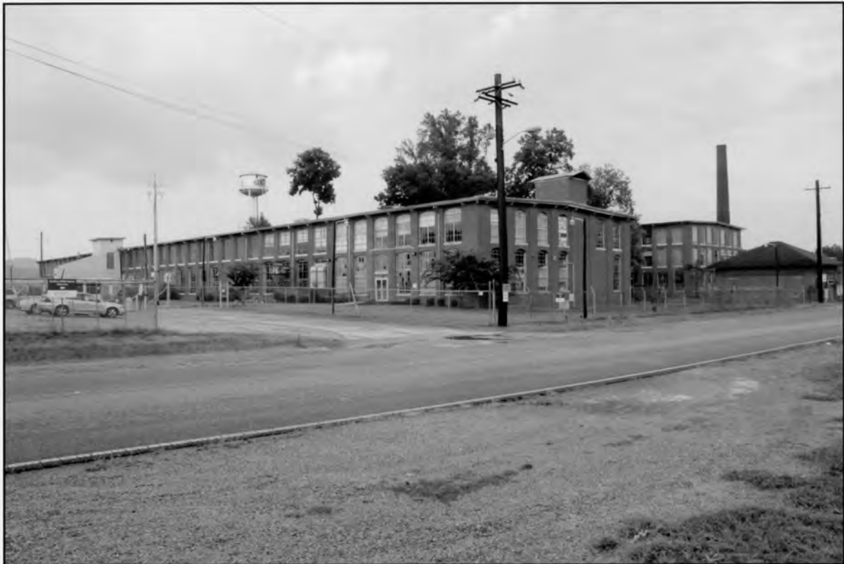
Lowe Mill and Mill Village Historic District Huntsville, Madison County, AL David B. Schneider December 2010 411 E. 6th St., Anniston AL 36207
