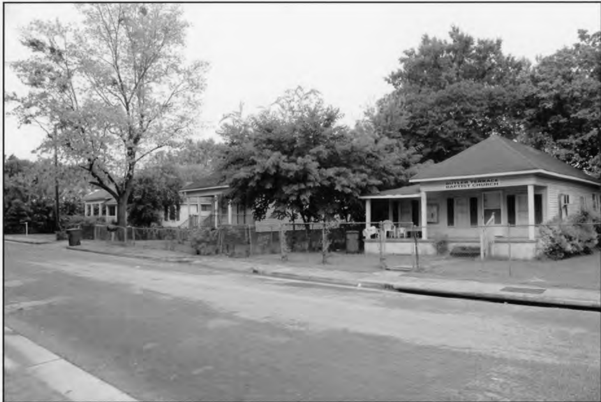
Lowe Mill and Mill Village Historic District Huntsville, Madison County, AL David B. Schneider December 2010 411 E. 6th St., Anniston AL 36207
