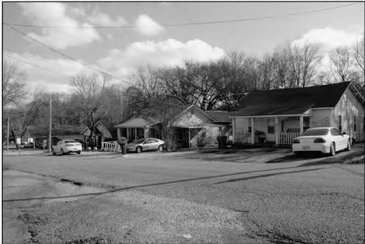
Lowe Mill and Mill Village Historic District Huntsville, Madison County, AL David B. Schneider December 2010 411 E. 6th St., Anniston AL 36207
