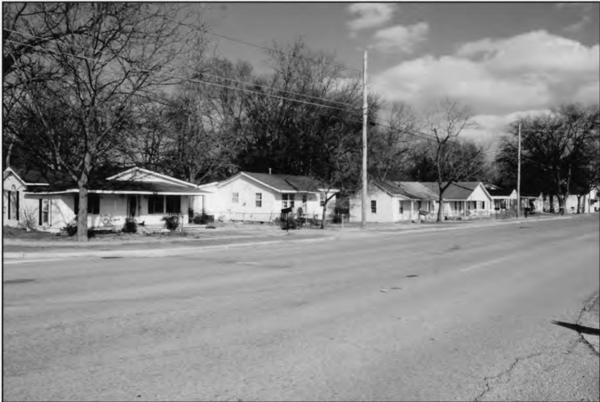
Lowe Mill and Mill Village Historic District Huntsville, Madison County, AL David B. Schneider December 2010 411 E. 6th St., Anniston AL 36207
