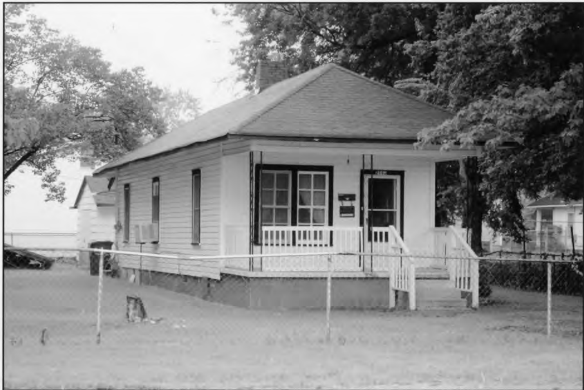
Lowe Mill and Mill Village Historic District Huntsville, Madison County, AL David B. Schneider December 2010 411 E. 6th St., Anniston AL 36207
