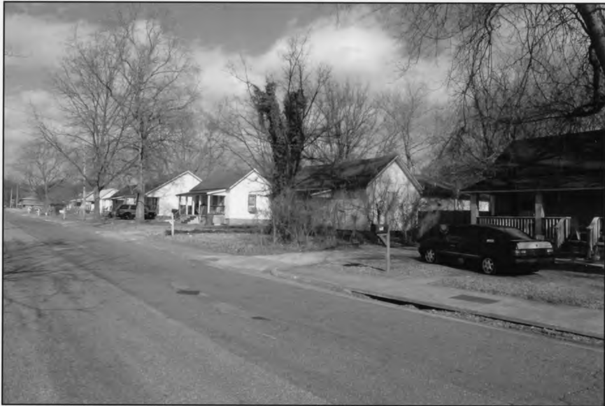
Lowe Mill and Mill Village Historic District Huntsville, Madison County, AL David B. Schneider December 2010 411 E. 6th St., Anniston AL 36207
