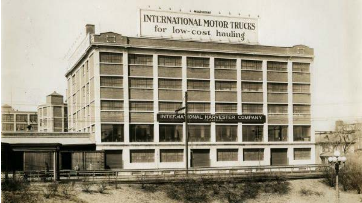
Figure 1 – International Harvester Company Building – Philadelphia Branch House, 1924. Courtesy of the Wisconsin Historical Society. https://www.wisconsinhistory.org/Records/Image/IM85789 . Accessed on July 25, 2017.
