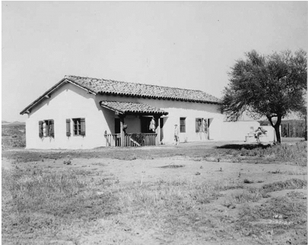
Figure 10. Juan María Osuna Adobe looking northeast, circa 1925. The photo shows the completed Lilian Rice rehabilitation. New tile roofing, plaster, windows, wood shutters, doors, railing, and front porch have been added. Source: Rancho Santa Fe Historical Society.
