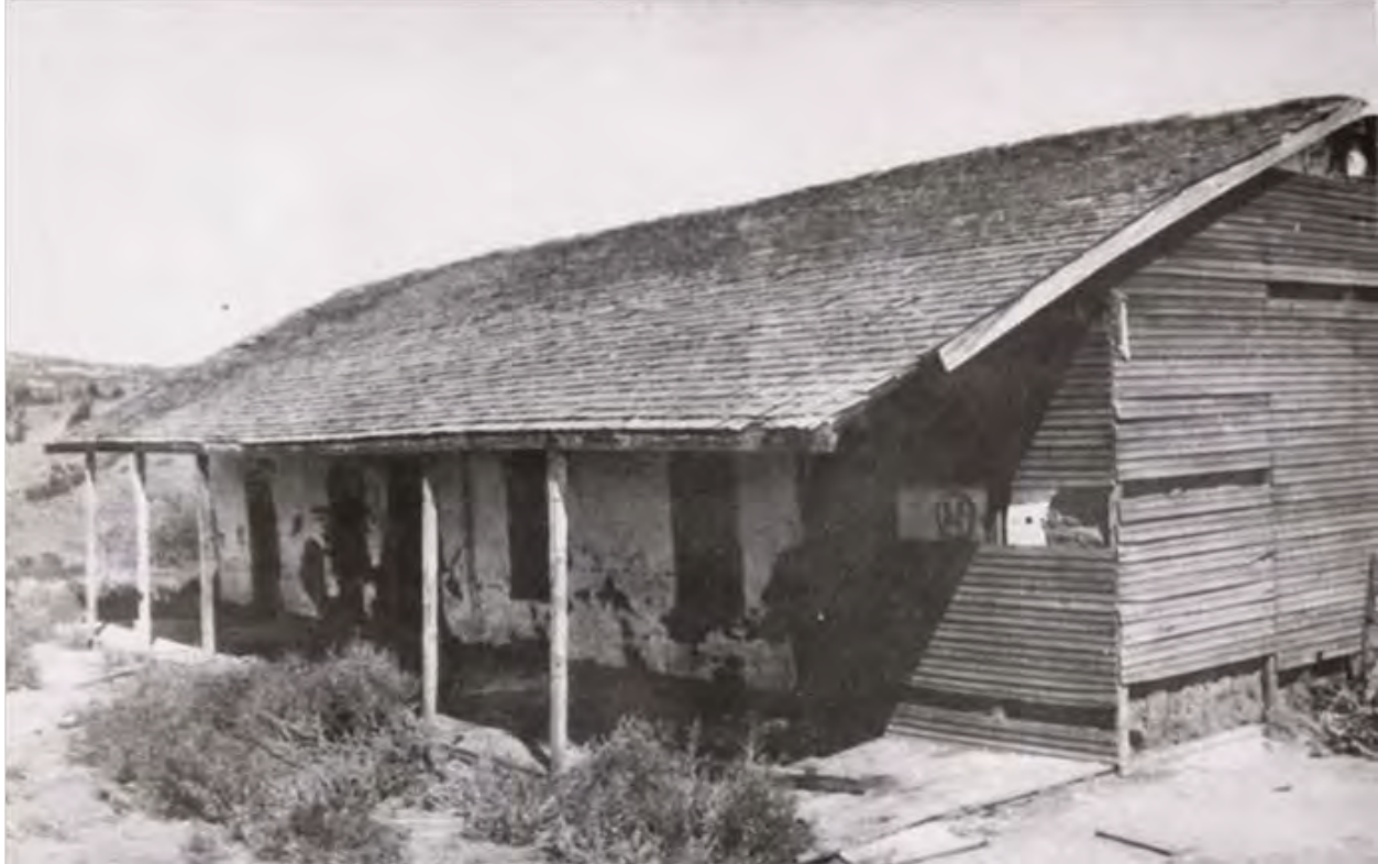
Figure 7. South elevation showing the original porch that extended along the entire south elevation with a raised wood porch deck. Source: Southwest Museum.
