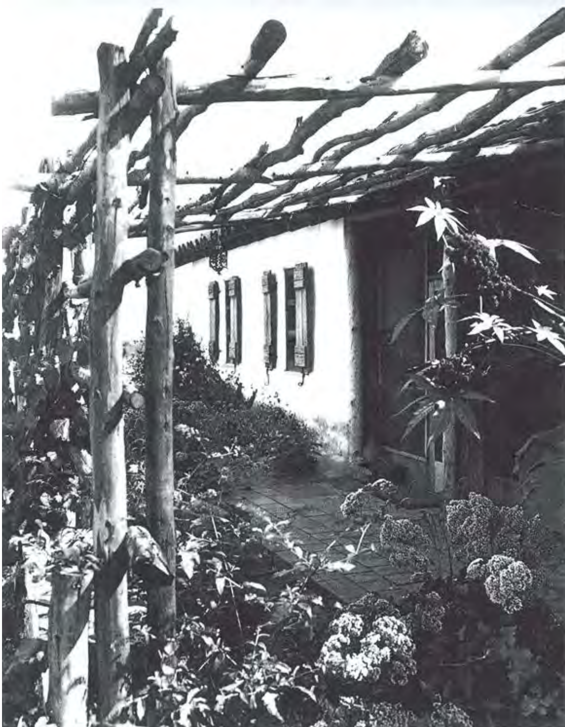
Figure 15. The rear porch shows the historic porch with a rustic wood trellis. The historic porch flooring is scored concrete matching the sleeping porch, circa 1925. Source: Rancho Santa Fe Historical Society.
