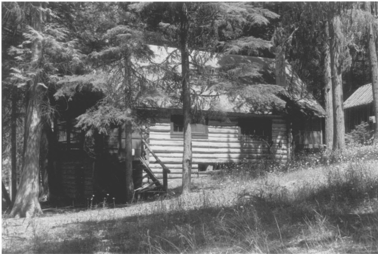
Dora Crump Cabin, Grevels Tourist Cabins Glacier National Park, Flathead County, Montana Photograph No. 1
