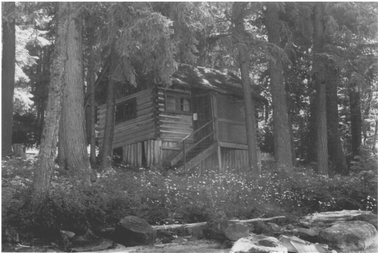
Cabin 4, Grevel's Tourist Cabins Glacier National Park, Flathead County, Montana Photograph No. 4
