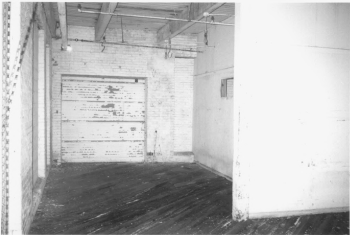
Fly Manufacturing Company Building Bedford Co. TN
