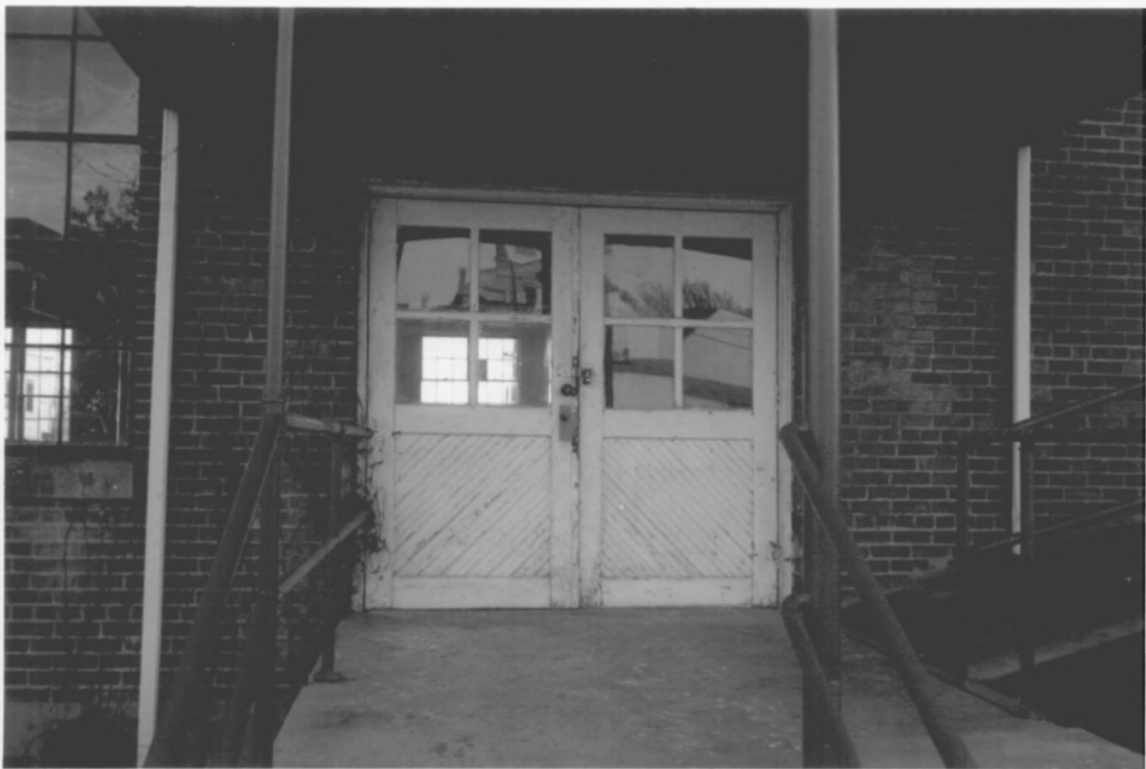
Fly Manufacturing Company Building Bedford Co. TN
