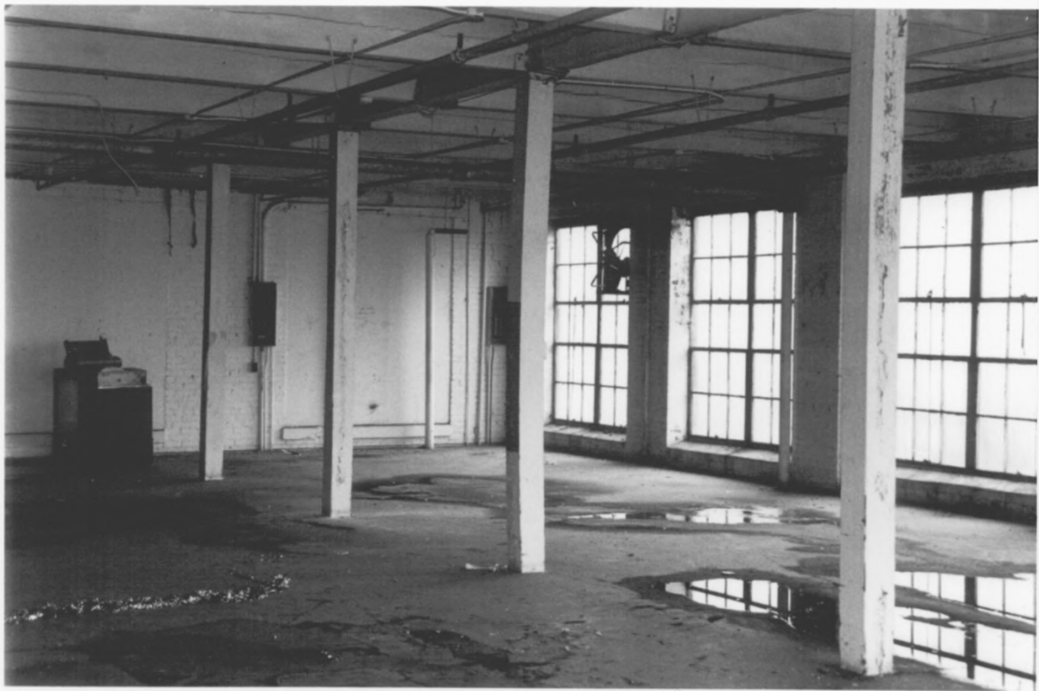
Fly Manufacturing Company Building Bedford Co. TN
