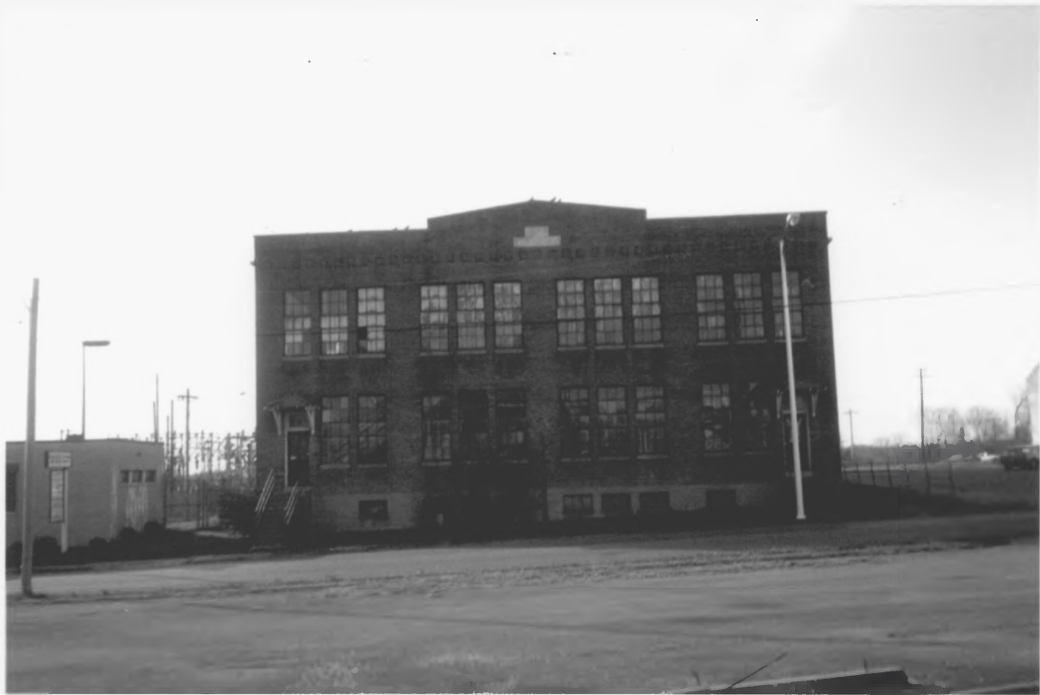
Fly Manufacturing Company Building Bedford Co. TN
