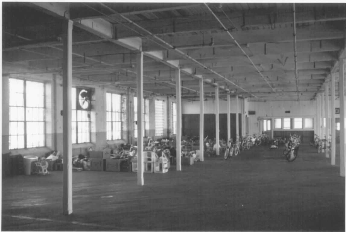
Fly Manufacturing Company Building Bedford Co. TN
