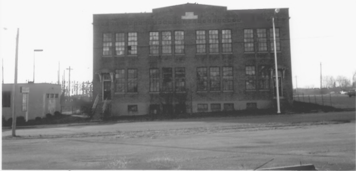
Fly Manufacturing Company Building Bedford Co. TN
