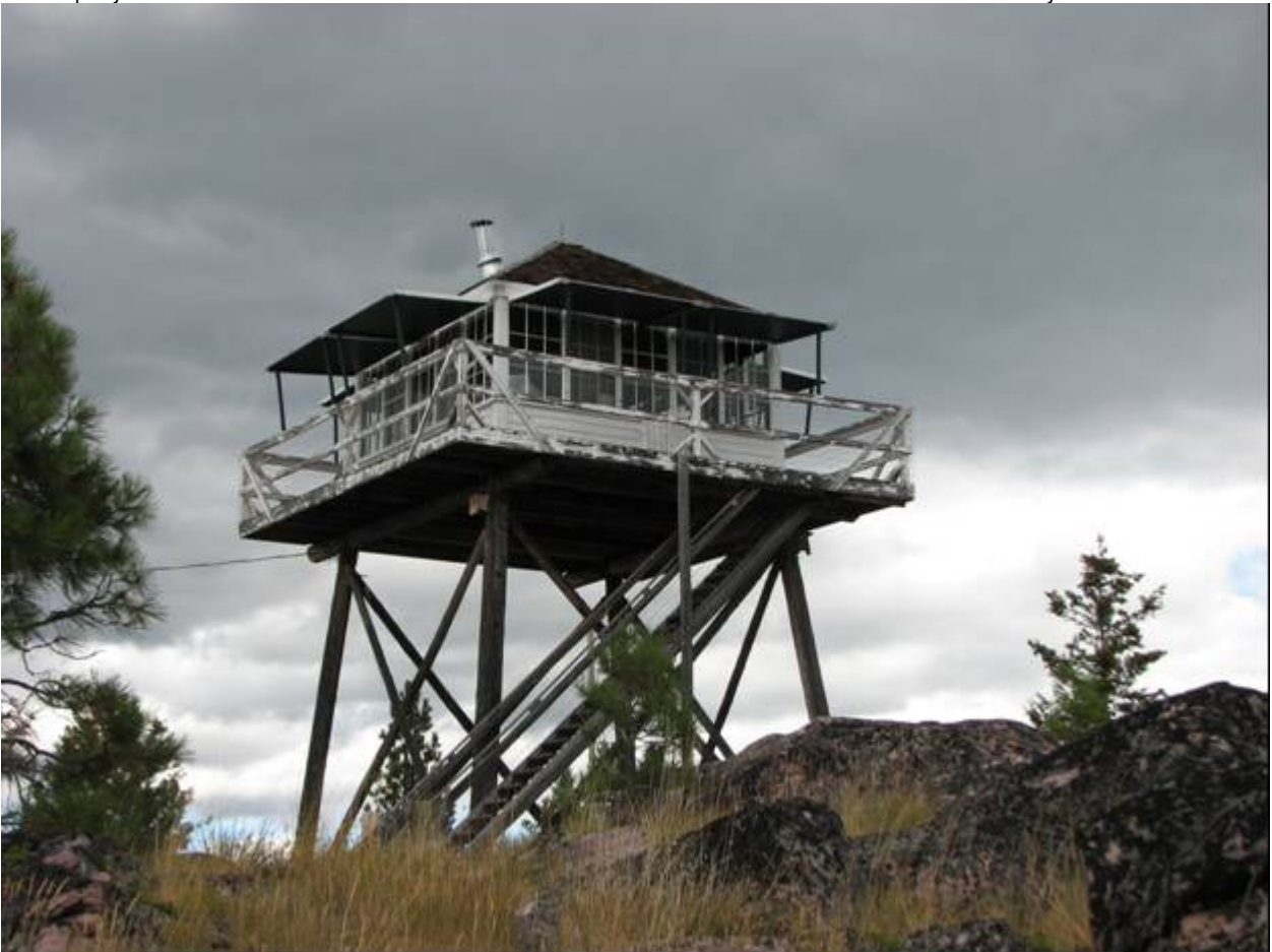
MT_MissoulaCounty_DoubleArrowLookout_0001. Looking northeast to the west and south walls of the Double Arrow Lookout.
