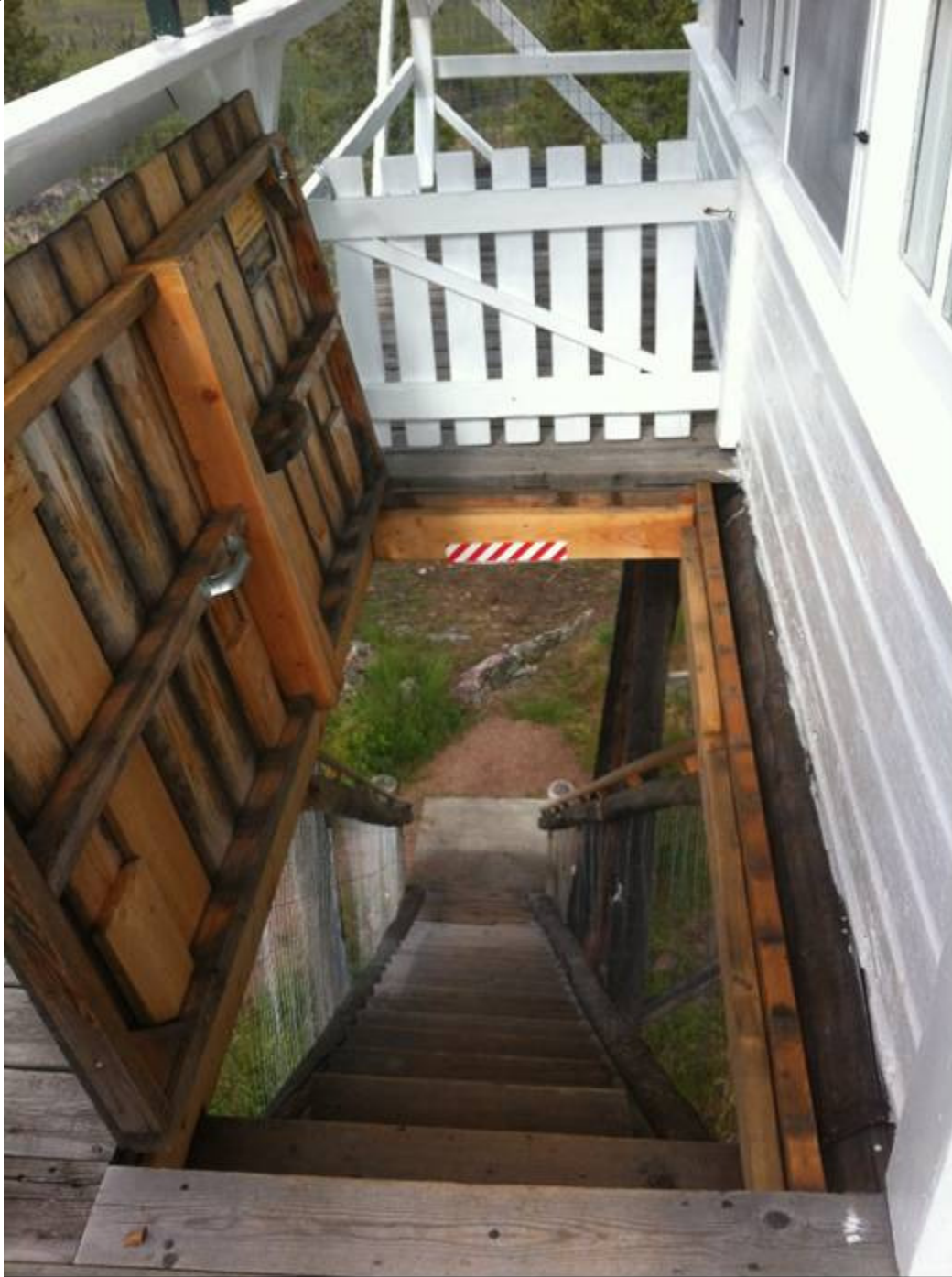
MT_MissoulaCounty_DoubleArrowLookout_0004. Looking down the stair through the open trapdoor.
