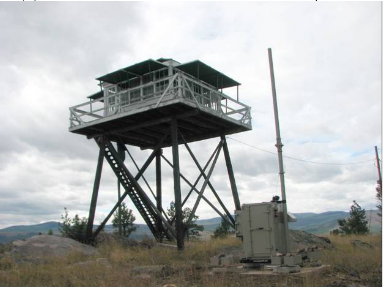
MT_MissoulaCounty_DoubleArrowLookout_0002. Looking south-southwest to the east (front) and north walls of the Double Arrow Lookout. Radio relay equipment in foreground.
