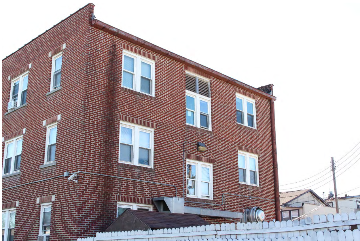
Photo 7 of 18: Upper back (north) wall, looking southwest.
