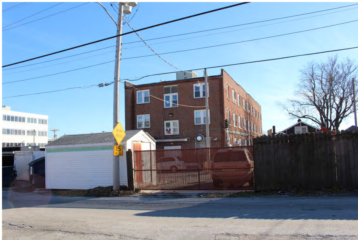
Photo 8 of 18: Back wall, looking south.
