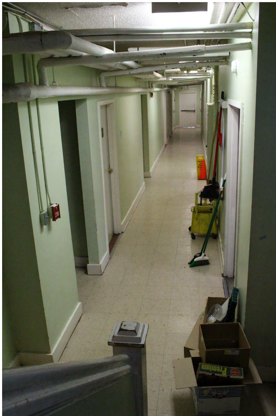
Photo 14 of 18: First floor, hall, looking south.
