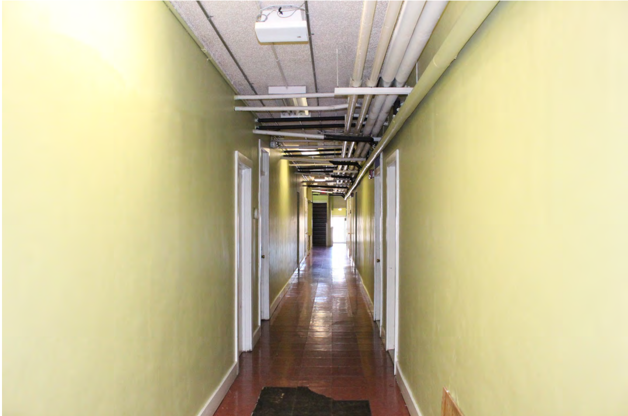
Photo 16 of 18: Second floor, hall, looking north.
