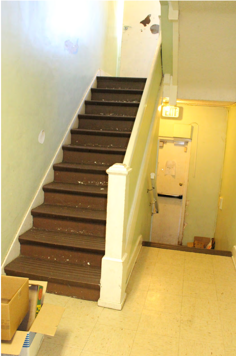
Photo 13 of 18: First floor, back (north) stair, looking north.
