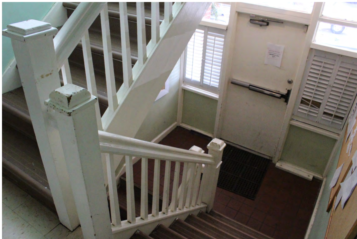
Photo 11 of 18: First floor, front stair, looking south.
