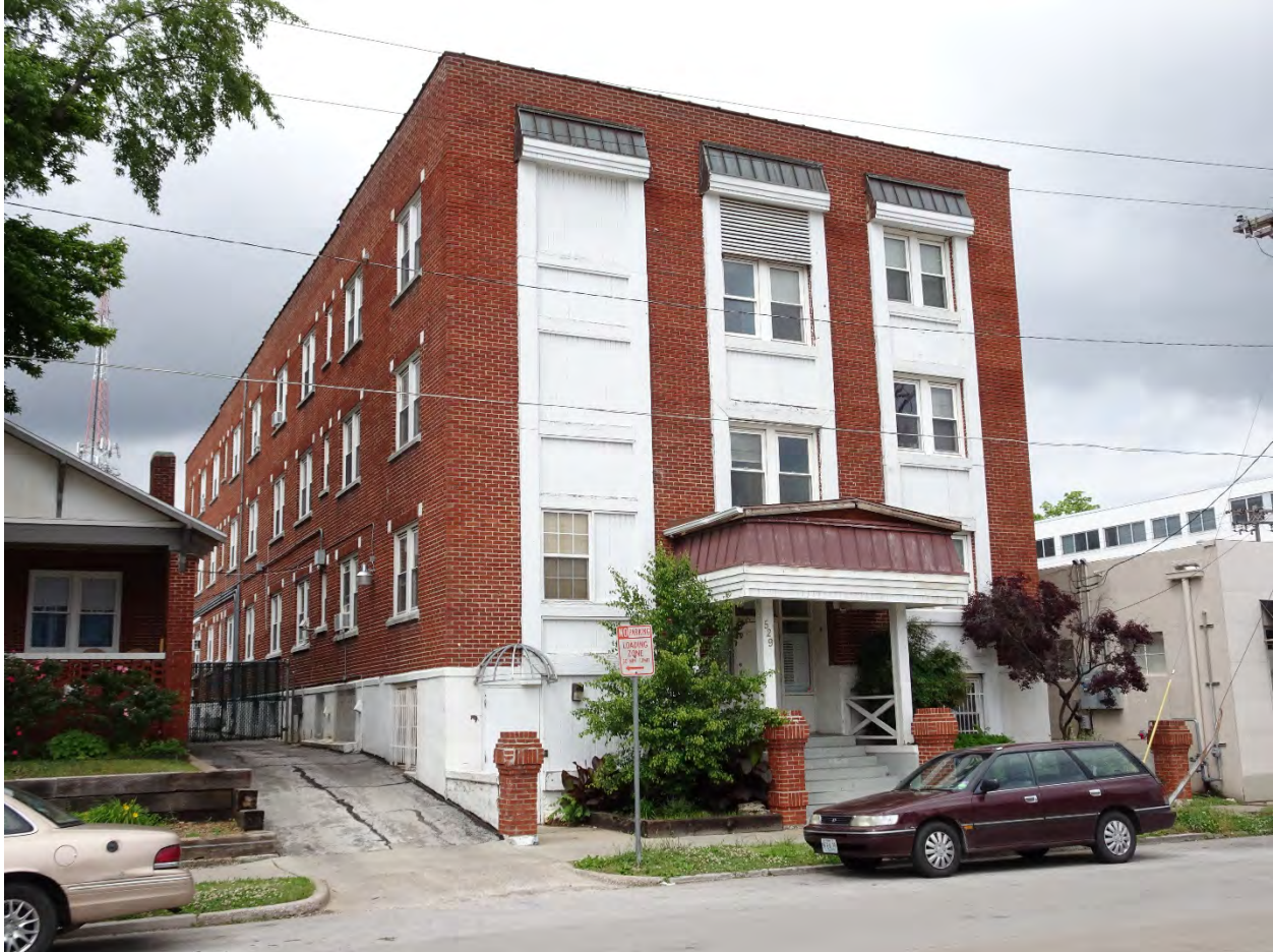
Figure 9. Beverly Apartments, summer 2016, before the removal of modern elements from the façade. Photo taken by Deb Sheals.
