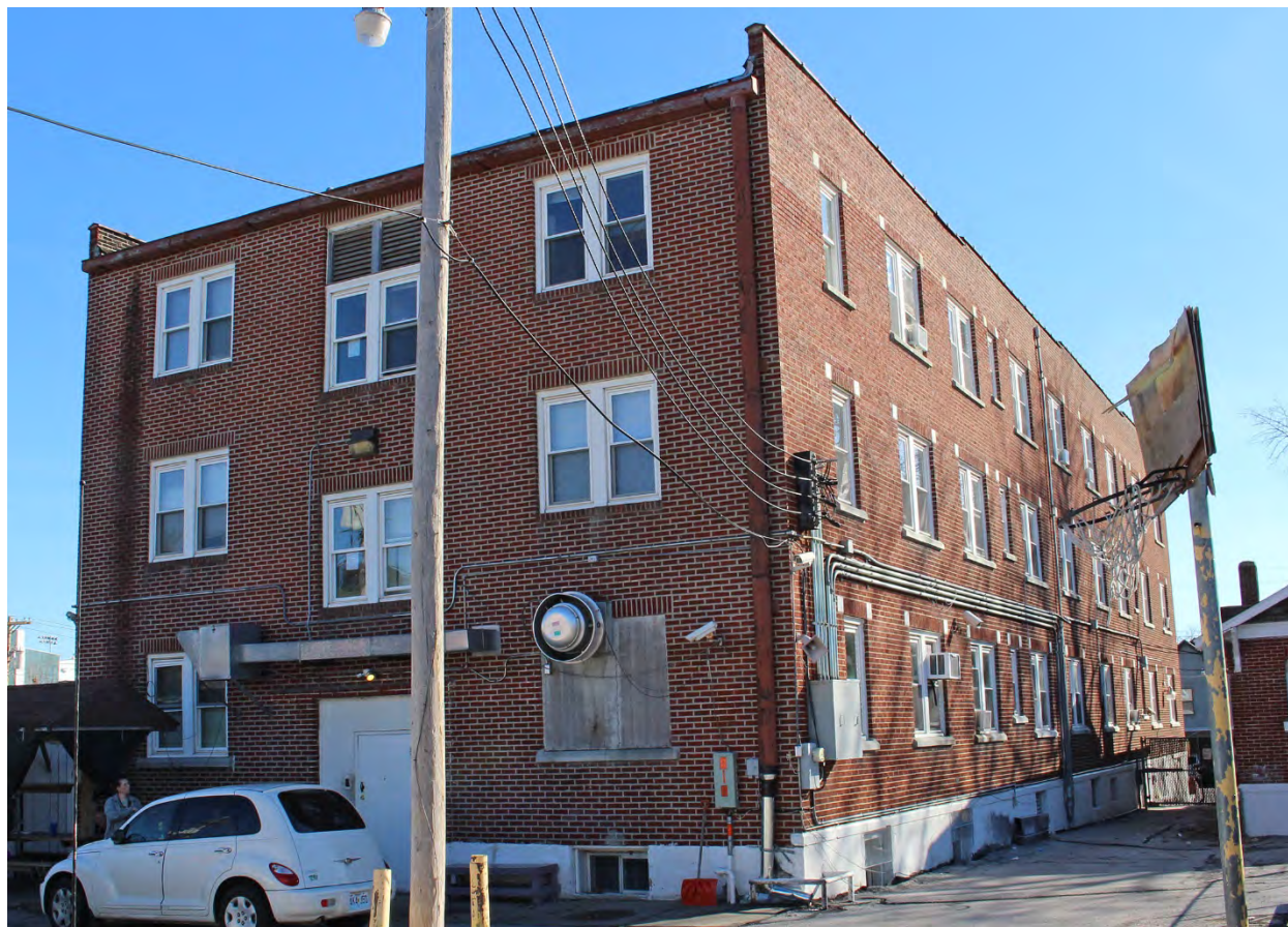
Photo 9 of 18: Northwest corner, looking southeast.
