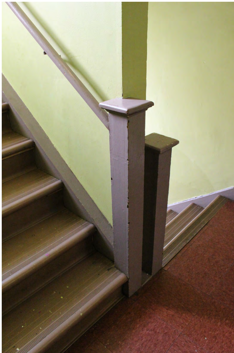
Photo 15 of 18: Second floor, front stair, looking south.
