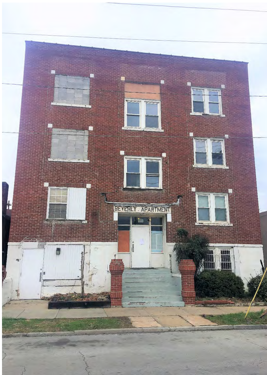
Photo 3 of 18: Façade (South wall), looking north.
