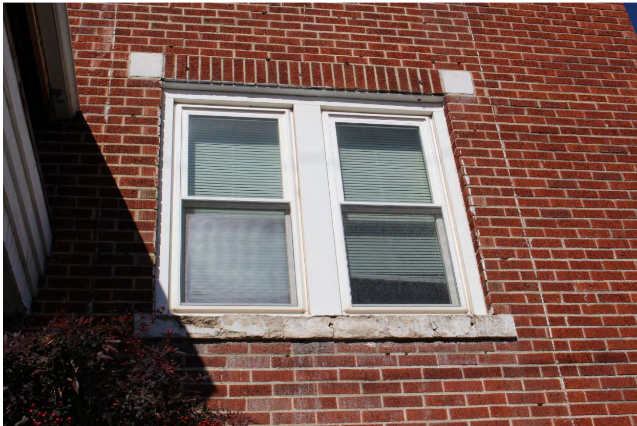
Photo 4 of 18: Window detail: façade, looking north.
