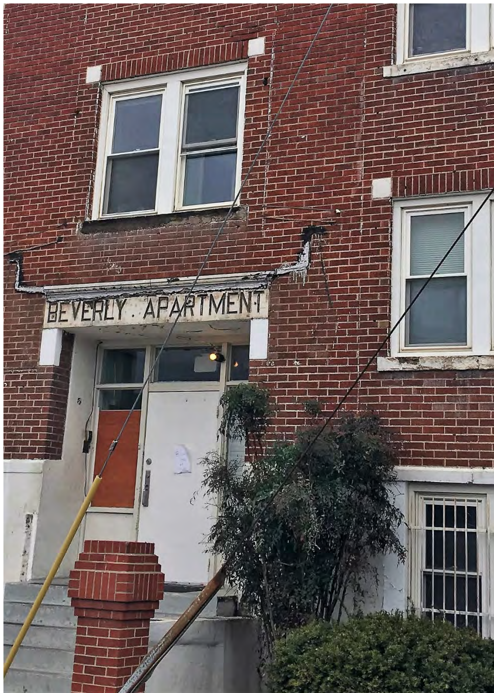
Photo 10 of 18: Front door, façade, looking northwest.
