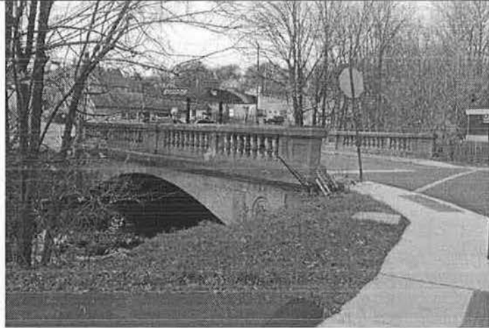
Photo 22. Pennsylvania Avenue Bridge, carrying Pennsylvania Avenue over Martin's Creek, facing west.
