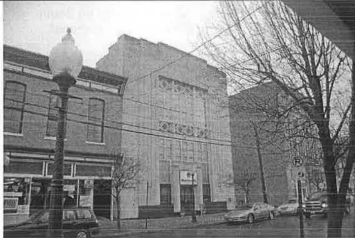
Photo 10. Merchants National Bank, 25 Broadway, facing NE.
