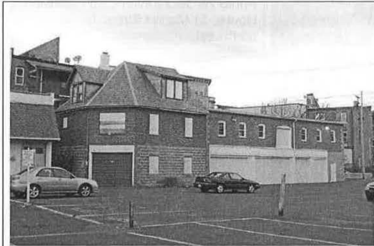
Photo 25. Outbuilding on Bracad Court (rear of 36 Market Street), facing north.
