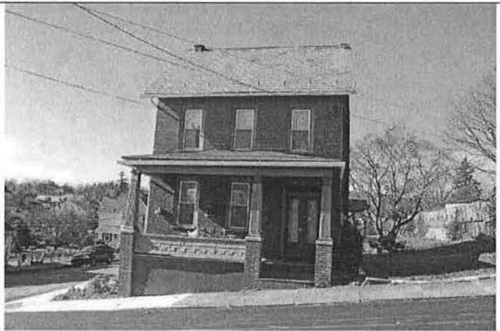
Photo 21. 204 North Fifth Street, facing west.
