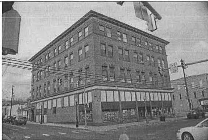
Photo 11. Bowers Building, 55 Broadway, facing NE
