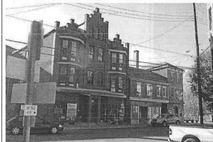
Photo 30. 3-part block located 28-34 South Main Street, facing southwest.
