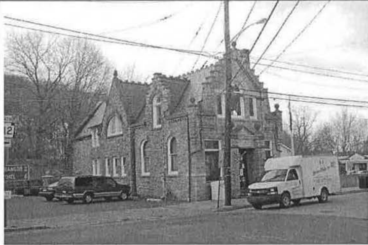
Photo 13. Bangor Public Library (built as the Merchants National Bank), 39 South Main Street, facing SW.
