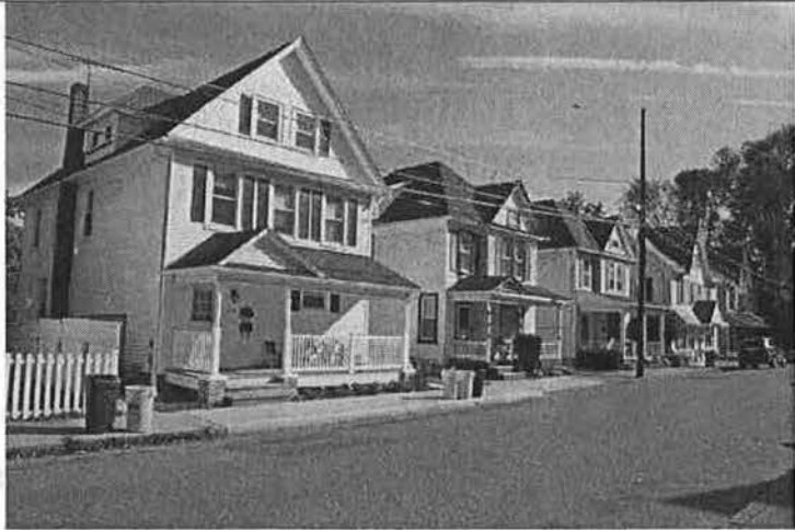
Photo 7. View of houses on South Second Street, facing southeast.
