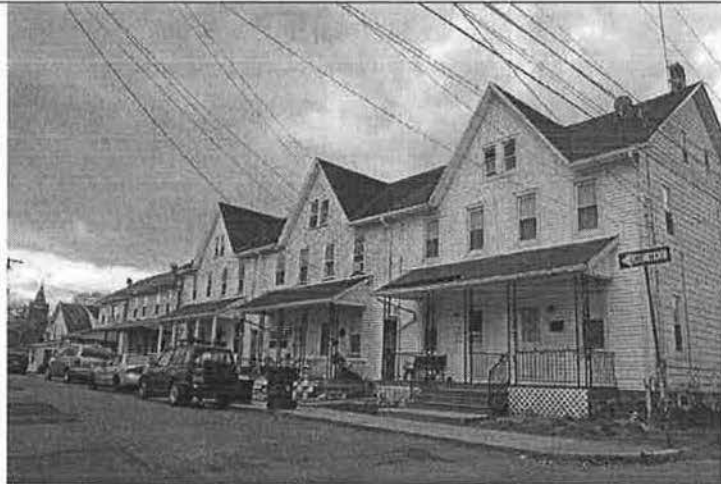
Photo 17. Worker's housing along North Second Street (24-48 North 2 nd Street), facing southwest.
