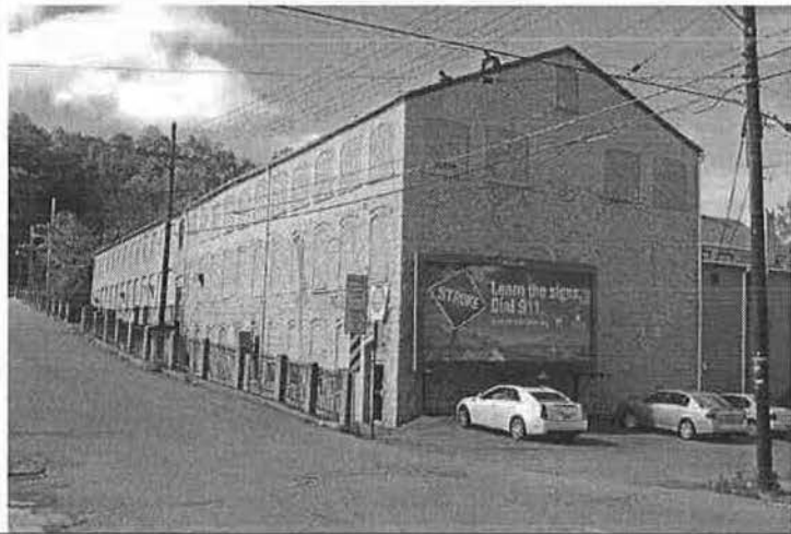
Photo 23. Sterling Silk Mill, 25 West Messinger Street, facing northwest.
