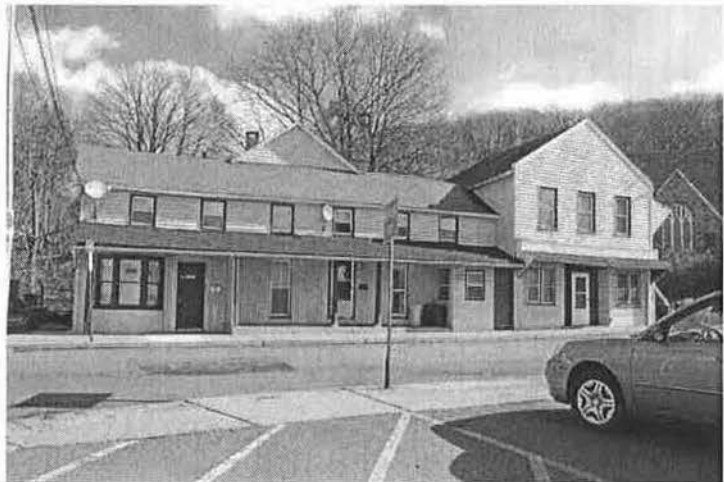
Photo 32. Slater's Row, 112 South Main Street, facing west.
