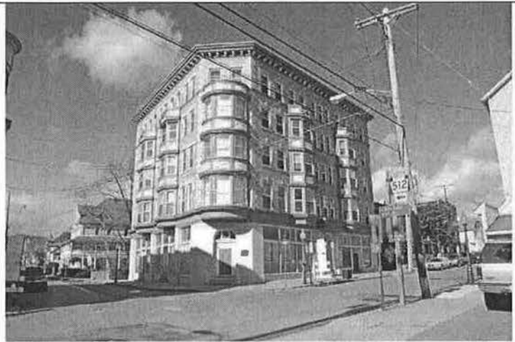
Photo 14. Real Estate Building, 17 Market Street, facing northwest.
