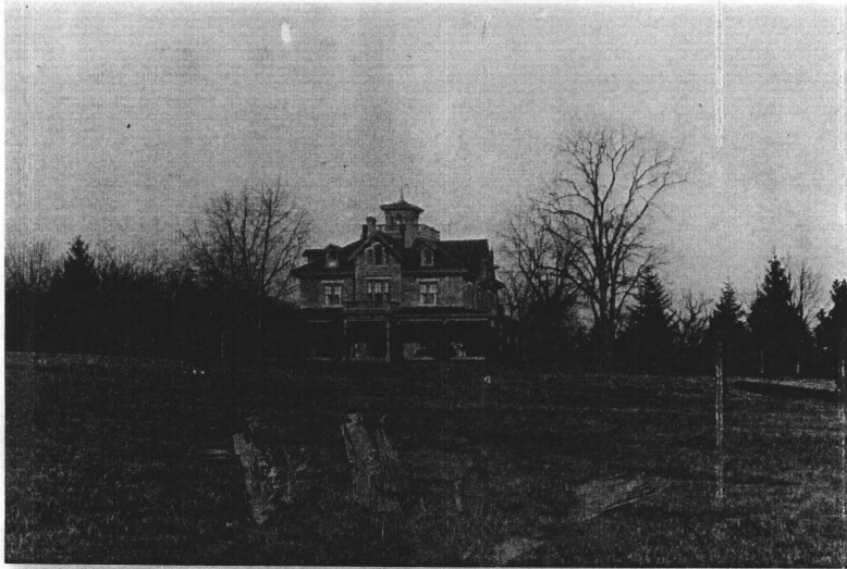
EXHIBIT 1 / Ruscombe 1886 – South elevation / front entry
