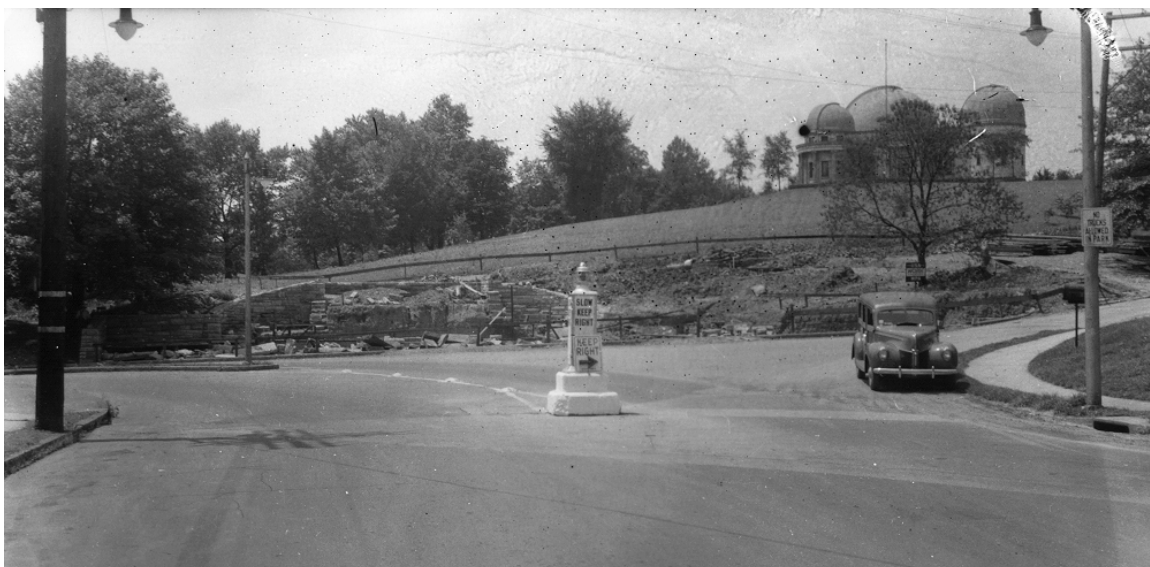
Figure 13. Riverview Avenue entrance under construction, 1940 (Pittsburgh City Photographer Collection)
