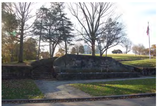
Photo 5: Double staircase and former fountain basin at Riverview entrance
