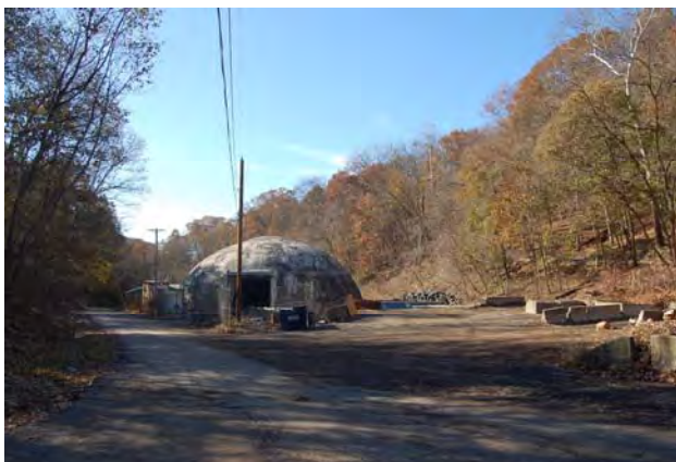
Photo 17: Public Works facility on Kilbuck Road near Grand Avenue entrance
