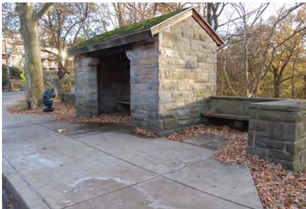
Photo 26: Bus shelter ensemble at Perrysville Avenue and Delaware Street.
