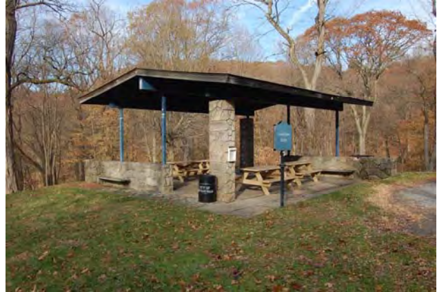
Photo 33: Locust Grove Shelter.
