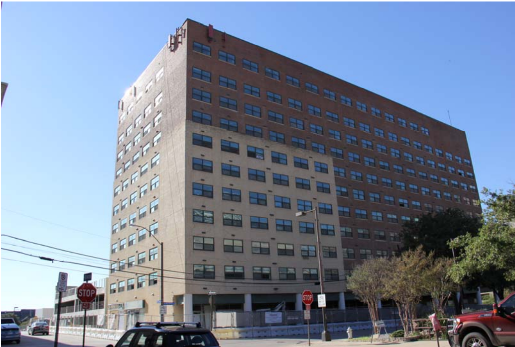
Photo 2 - South Elevation (West 2nd Street) at left and East Elevation (Burnett Street) at right. Camera facing Northeast.
