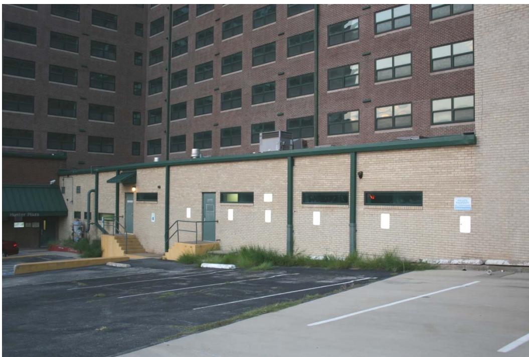
One story, tan brick wall at South Elevation. Camera facing Northeast.
