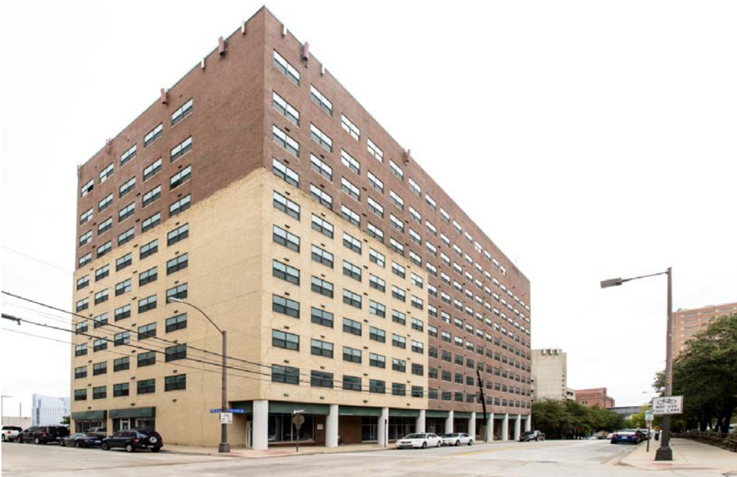
South Elevation (West 2nd Street) and East Elevation (Burnett Street). Camera facing Northwest. James F. Wilson, photographer. October 14, 2014.
