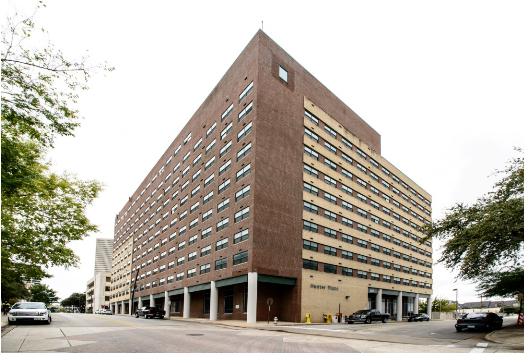
East (left) and North (right) elevations. Camera facing Southwest. James F. Wilson, photographer. October 14, 2014.
