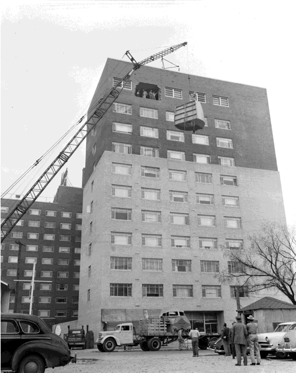
Mockup section of a DC-6 hoisted into the open hole in the South wall of the Fortune Arms apartments where it would be used in the American Airlines pilots and engineers school, 1957. Courtesy of UTA Special Collections Library. Fort Worth Star-Telegram 's historic photos of Fortune Arms.
