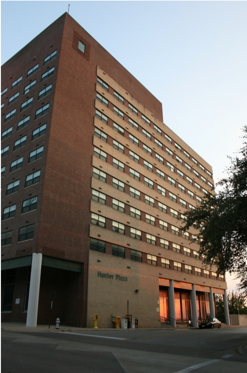
North Elevation. Camera facing Southwest. James F. Wilson, photographer. October 14, 2014.
