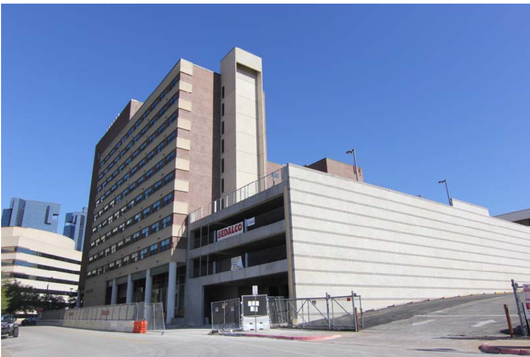
Photo 3 - North Elevation (West 1st Street) with garage in foreground. Camera facing Southeast.
