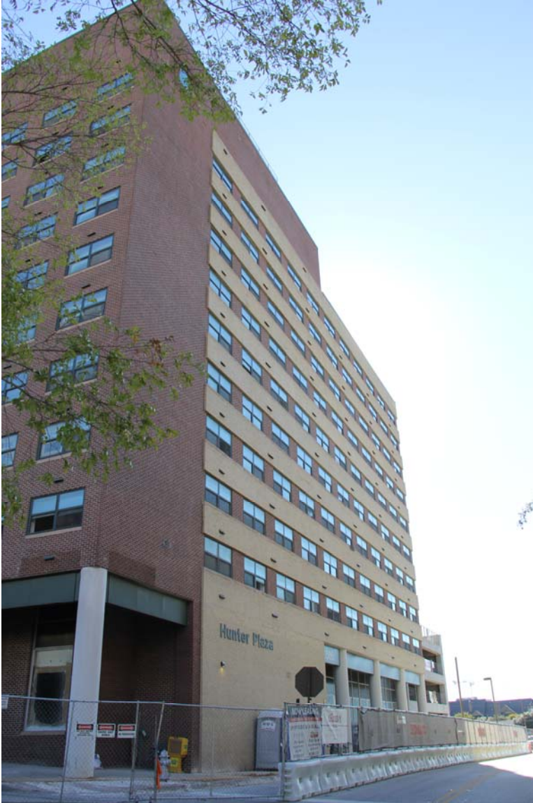
Photo 1 - Partial East Elevation (Burnett Street) at left) and North Elevation ( West 1st Street) at right. Camera facing West. Garage seen at far right (west) of North Elevation.
