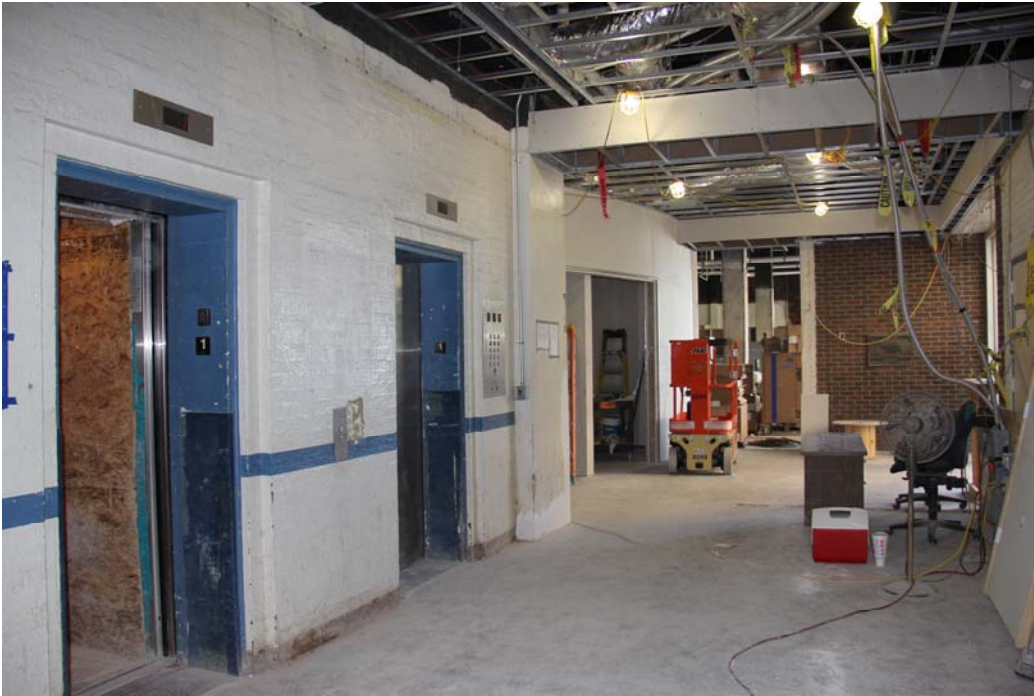
Photo 4 - View of the First Floor Lobby. Camera facing West.
