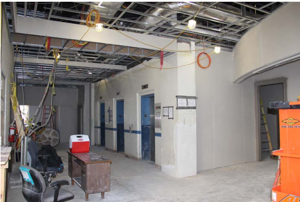
Photo 5 - View of the First Floor Lobby. Camera facing East.
