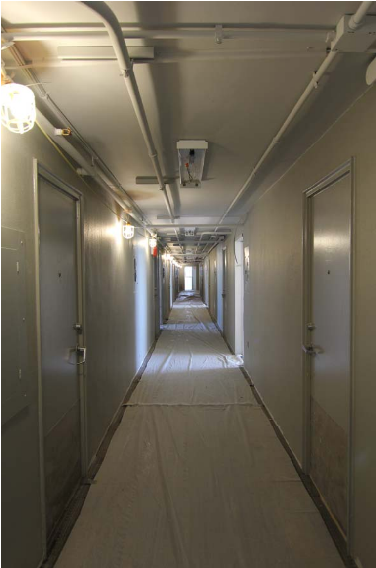
Photo 8 - View of typical Corridor at floors 2 - 9. Camera facing south.
