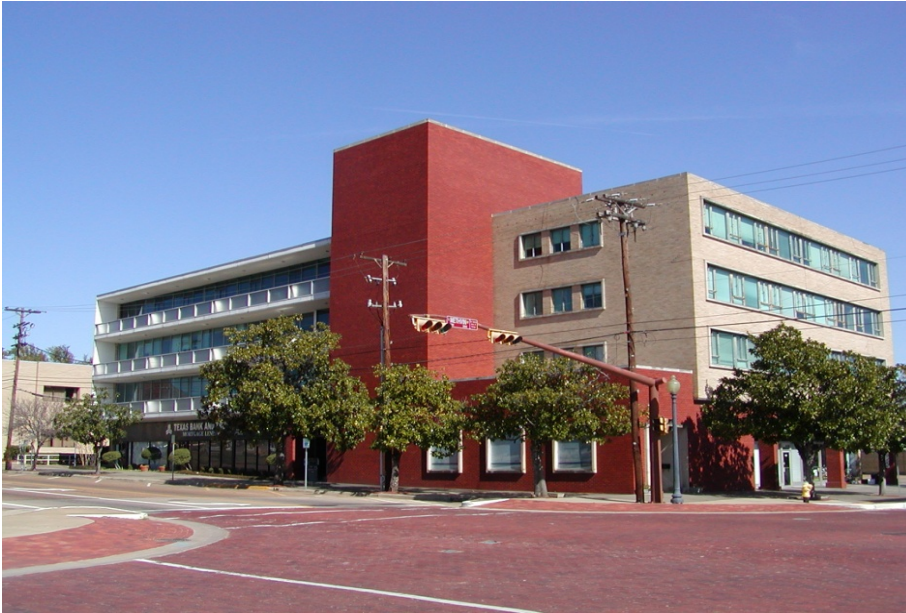
Office building in Kilgore, Texas c. 1950s
