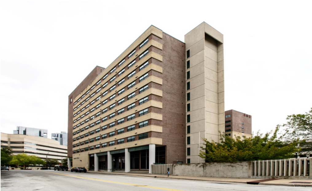
North facade (at West 1st Street) at left and West facade (facing patio). Camera facing Southeast. Concrete stair tower addition completed in 1973.
