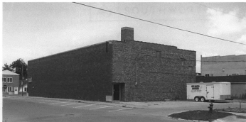
Figure 4 Current view of The Avery's long south side wall along 5 th Street (left) and the narrower rear wall and parking area. Tallgrass Historians L.C. photograph, 2007.
