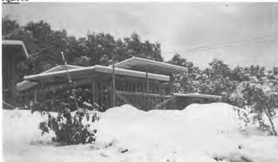
Photograph of house under construction, view facing southwest, 1949, courtesy of Theodore Thomas, Jr.
