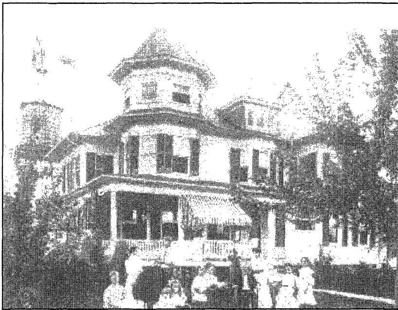
Figure 10. The "Ough House" in Friendship Heights in Bethesda, Maryland, is believed to have been designed and occupied by architect Richard Ough, the architect of the Palisades of the Potomac Land Improvement Company.
