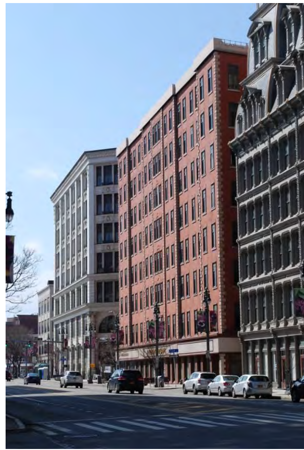
Former hotel in 2019 showing sheathing removed
