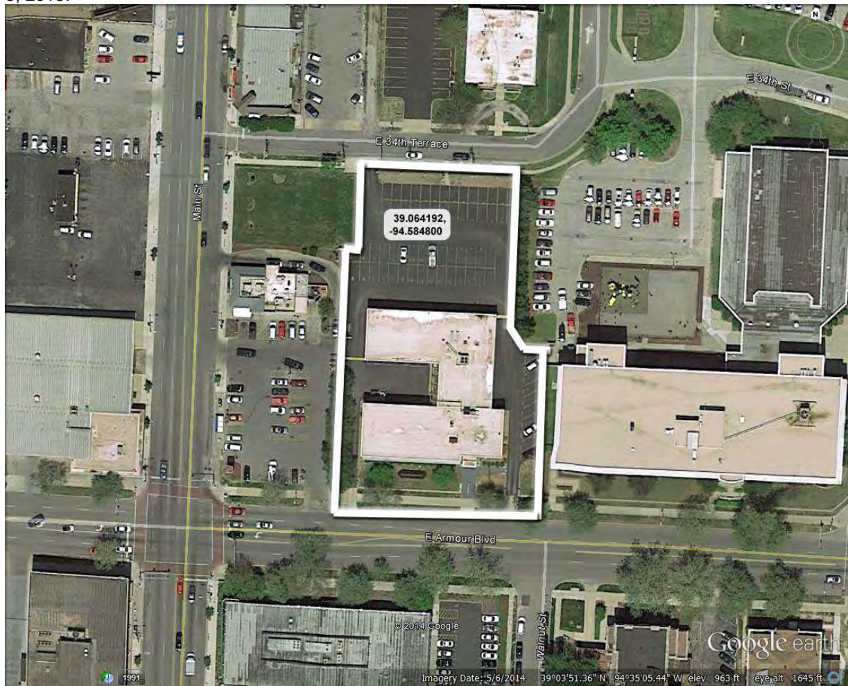
Figure 1. Site Map with National Register nominated property outlined. Google Earth. Accessed January 5, 2015.
