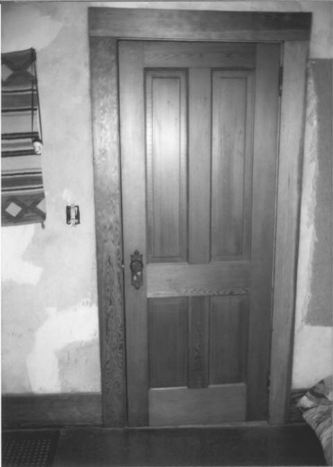
10 of 10 Typical four-paneled door and hardware.
