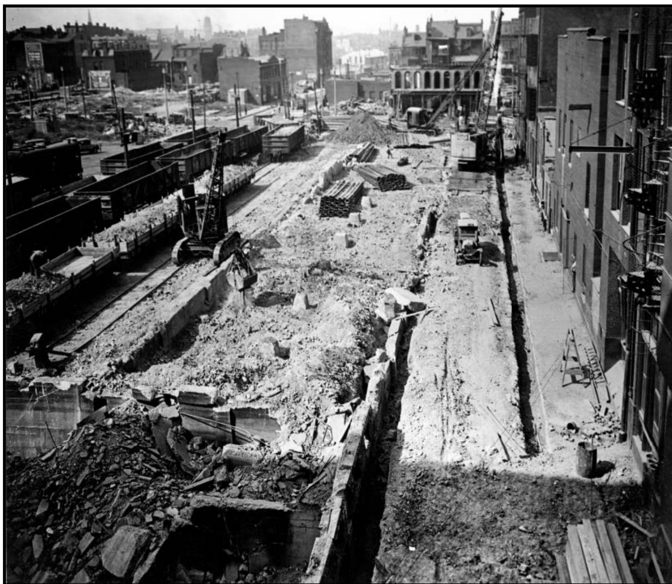
Figure 21: Photograph of site standing on Lucas Avenue between 12 th and 11 th Streets facing north, August 21, 1930. The exposed foundation is a portion of the former freight house. Source: Collection of Dale Jenkins, Illinois Traction Society.
