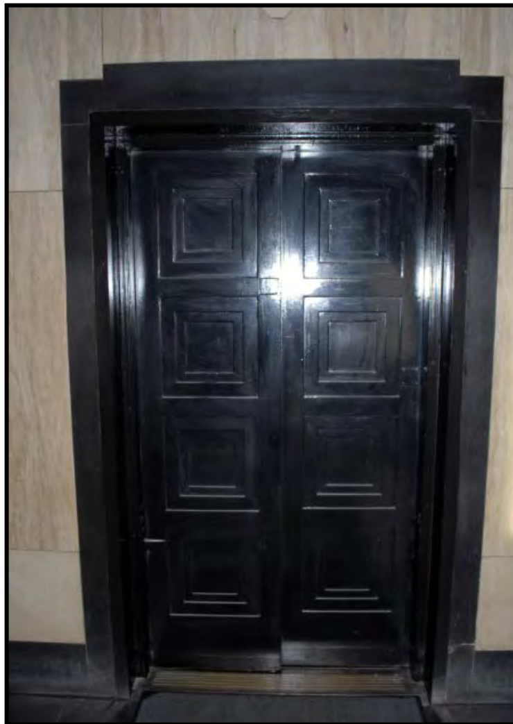
Figures 3A and B (top to bottom): Figure 3A shows one of the original elevator bays; Figure 3B is the original directory board. Source: Matt Bivens, 2014-2016.
