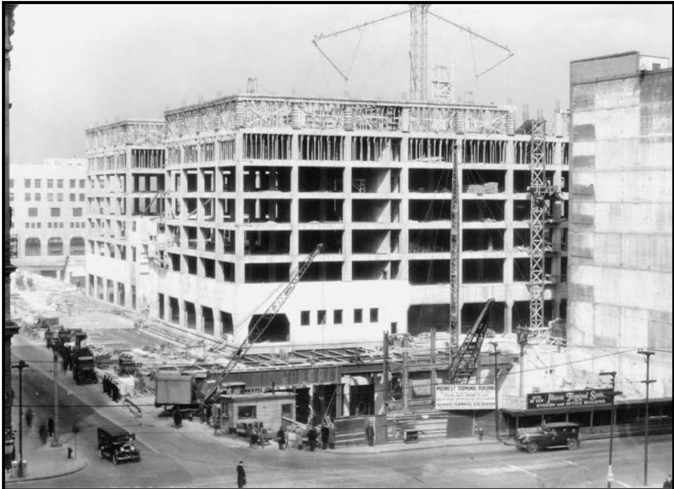
Figure 24: Photograph of construction, 1932. Source: Collection of Dale Jenkins, Illinois Traction Society.
