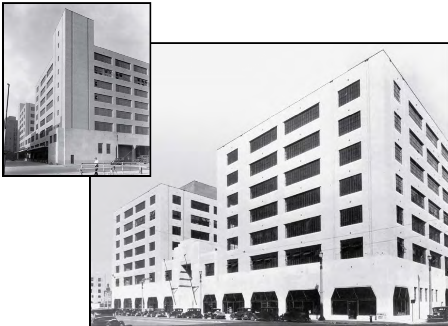
Figure 25: Photographs of completed construction, 1932. The larger image is the primary elevation; the smaller image is the rear, east elevation (left side) with a portion of the north elevation (right side). Source: Collection of Dale Jenkins, Illinois Traction Society.
