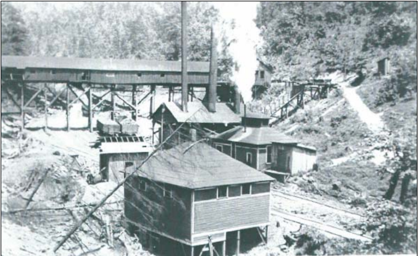
Figure 5: View of the Rex #2 Mine at LaFollette Coke Ovens, circa 1910. The building in the front is the tippie, with a powerhouse building located beneath the two smokestacks. (Source: John Van Huss, The Rise and Fall of Ivydell ; Campbell County Historical Society)
