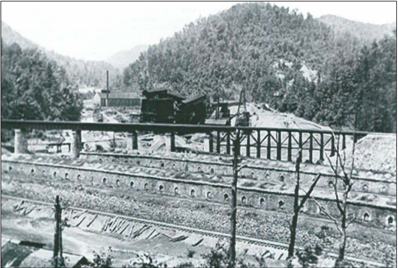
Figure 7: Overview of LaFollette Coke Ovens complex, approximately 1910. The east coke ovens are located in the foreground, with the coal washer and washed-coal bunker located in the center of the photograph, behind the L&N trestle. The west coke ovens are behind the coal bunker. (Source: John Van Huss, The Rise and Fall of Ivydell ; Campbell County Historical Society)
