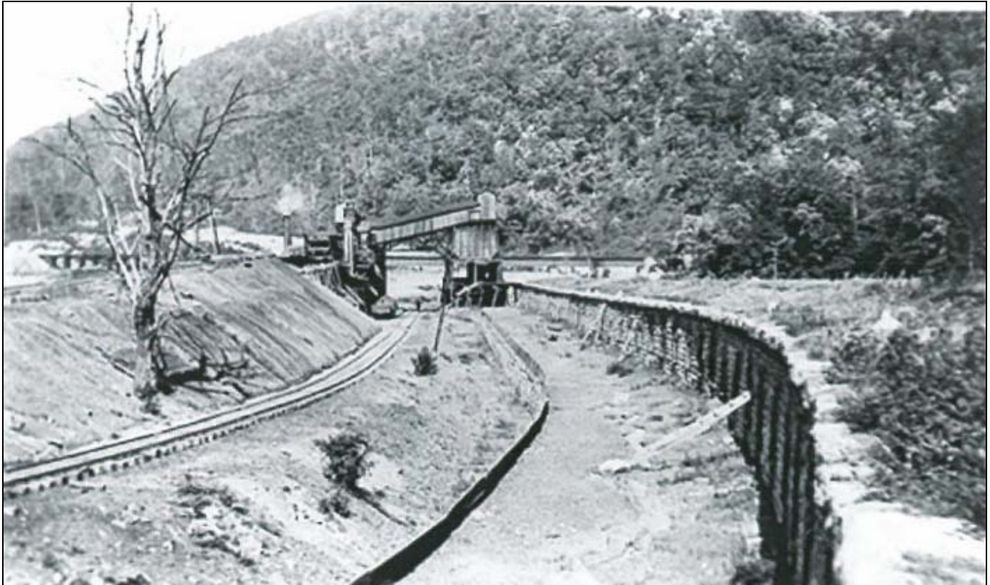
Figure 12: View of the west battery of coke ovens at LaFollette Coke Ovens and the coal washer and washed-coal bunker. No date attributed to photograph. (Source: John Van Huss, The Rise and Fall of Ivydell ; Campbell County Historical Society)
