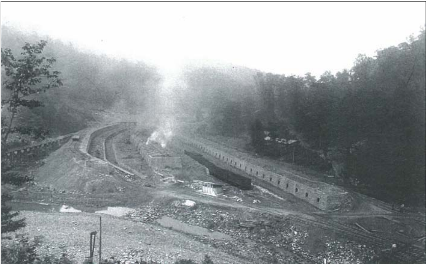
Figure 8: View of the east coke oven batteries at LaFollette Coke Ovens from present-day Highway 25W, approximately 1915. Trains with coke-racks are located between the two batteries. (Source: John Van Huss, The Rise and Fall of Ivydell ; Campbell County Historical Society)
