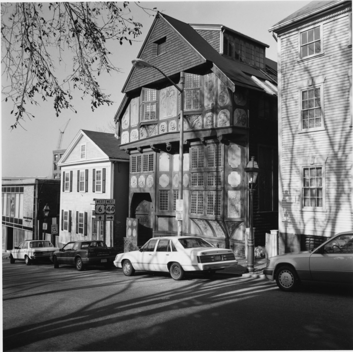
FLEUR-DE-LYS STUDIOS Providence, Rhode Island Front facade on Thomas Street Photo by B. Clarkson Schoettle, 11/91
