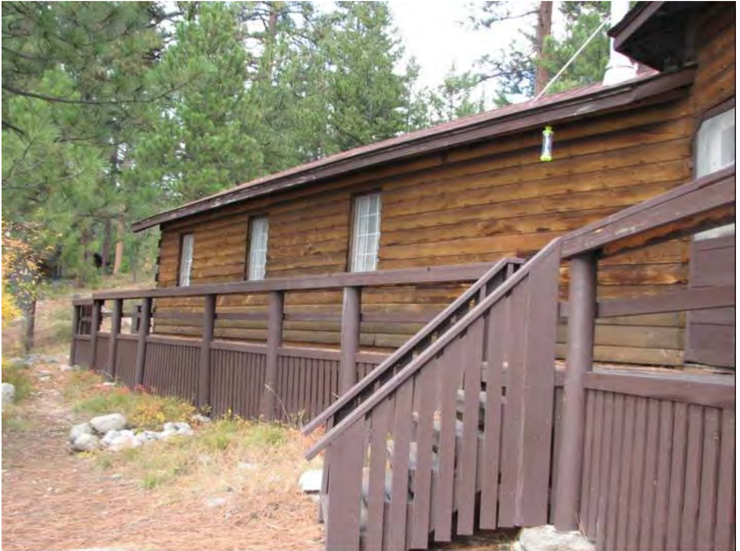
Photo 0007 Looking northwest along the south wall of the west wing.
