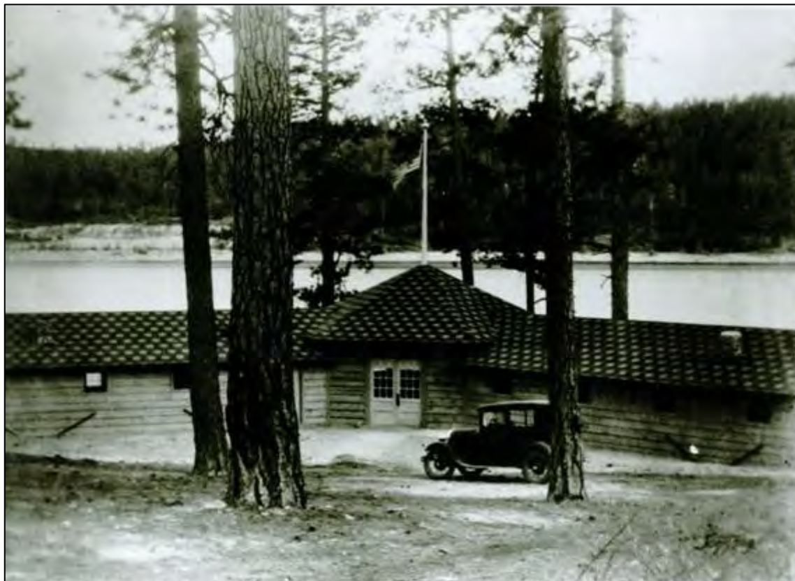
Figure 4. Photo of Hayward Lodge as originally constructed (BNF HF).
