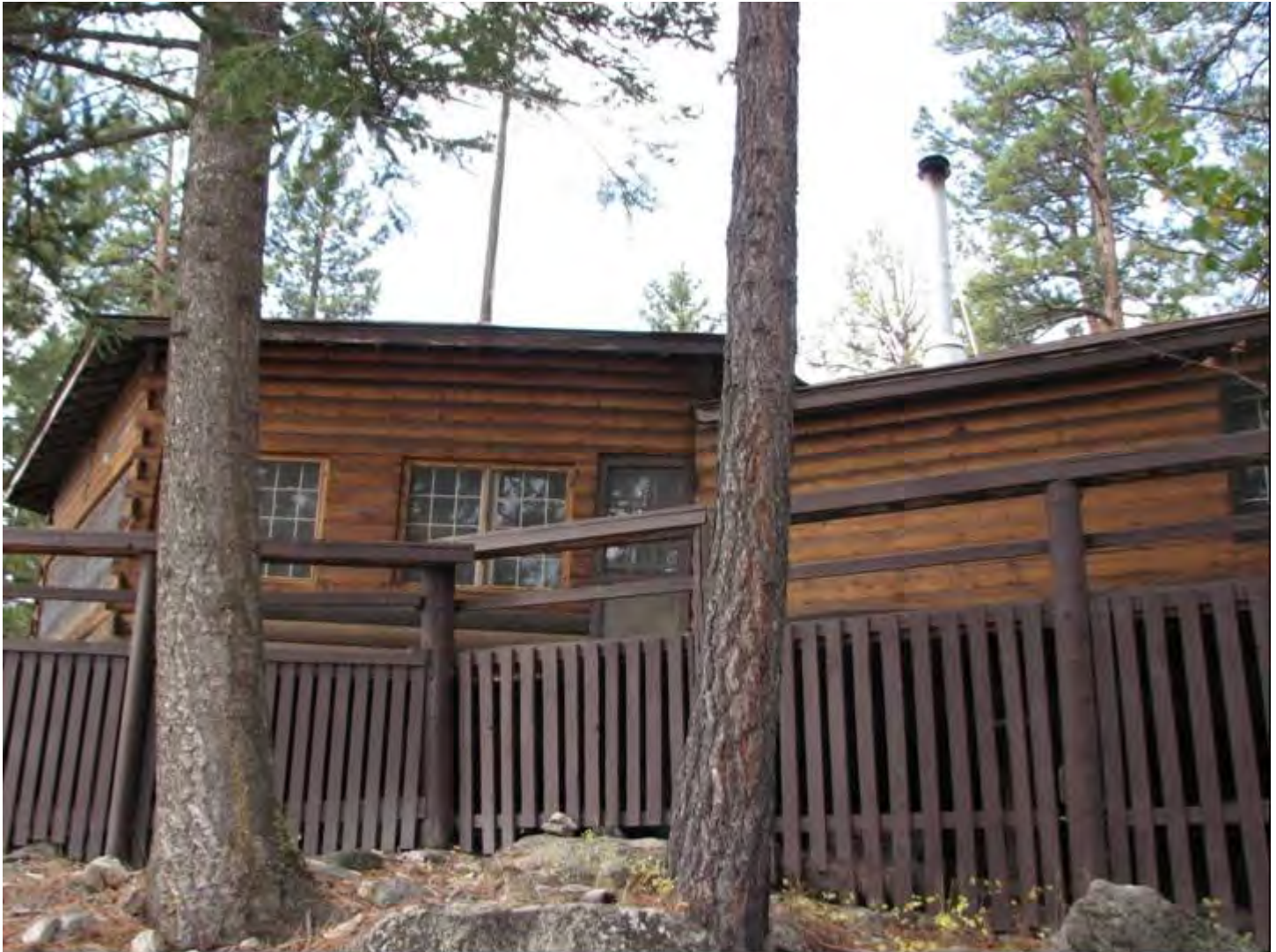
Photo 0005 Hayward Lodge: looking northwest to the south walls of the hexagonal component (left) and the east wing.
