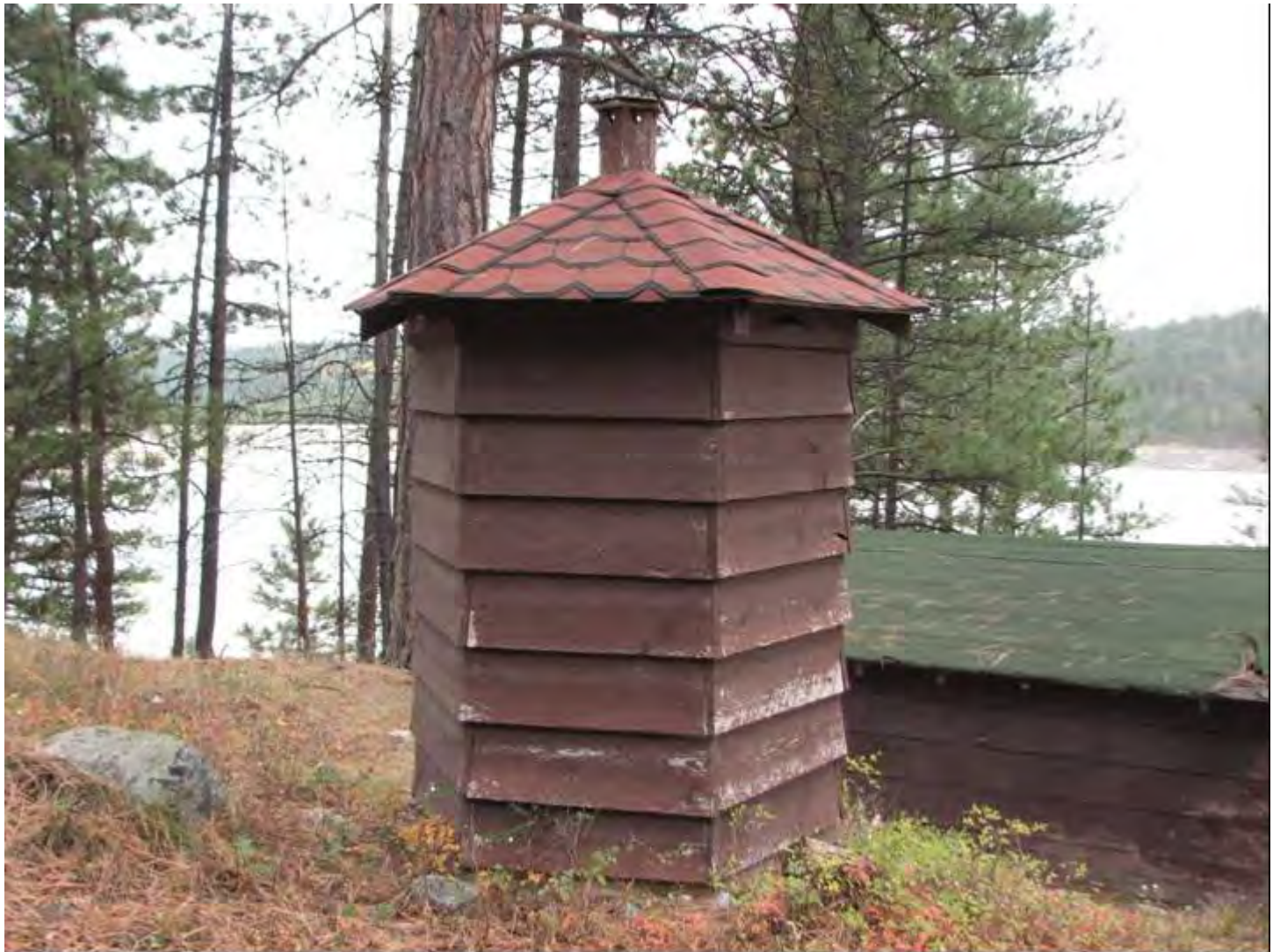
Photo 0013 Hayward Lodge outhouse: looking south to the rear of the outhouse.
