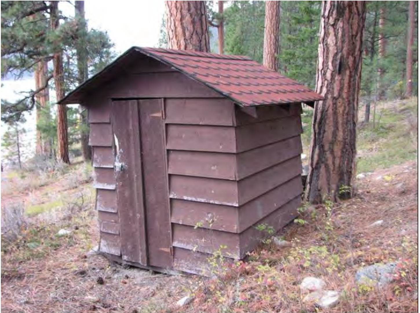
Photo 0016 Hayward Lodge generator shed: looking west to the front and northeast side walls.
