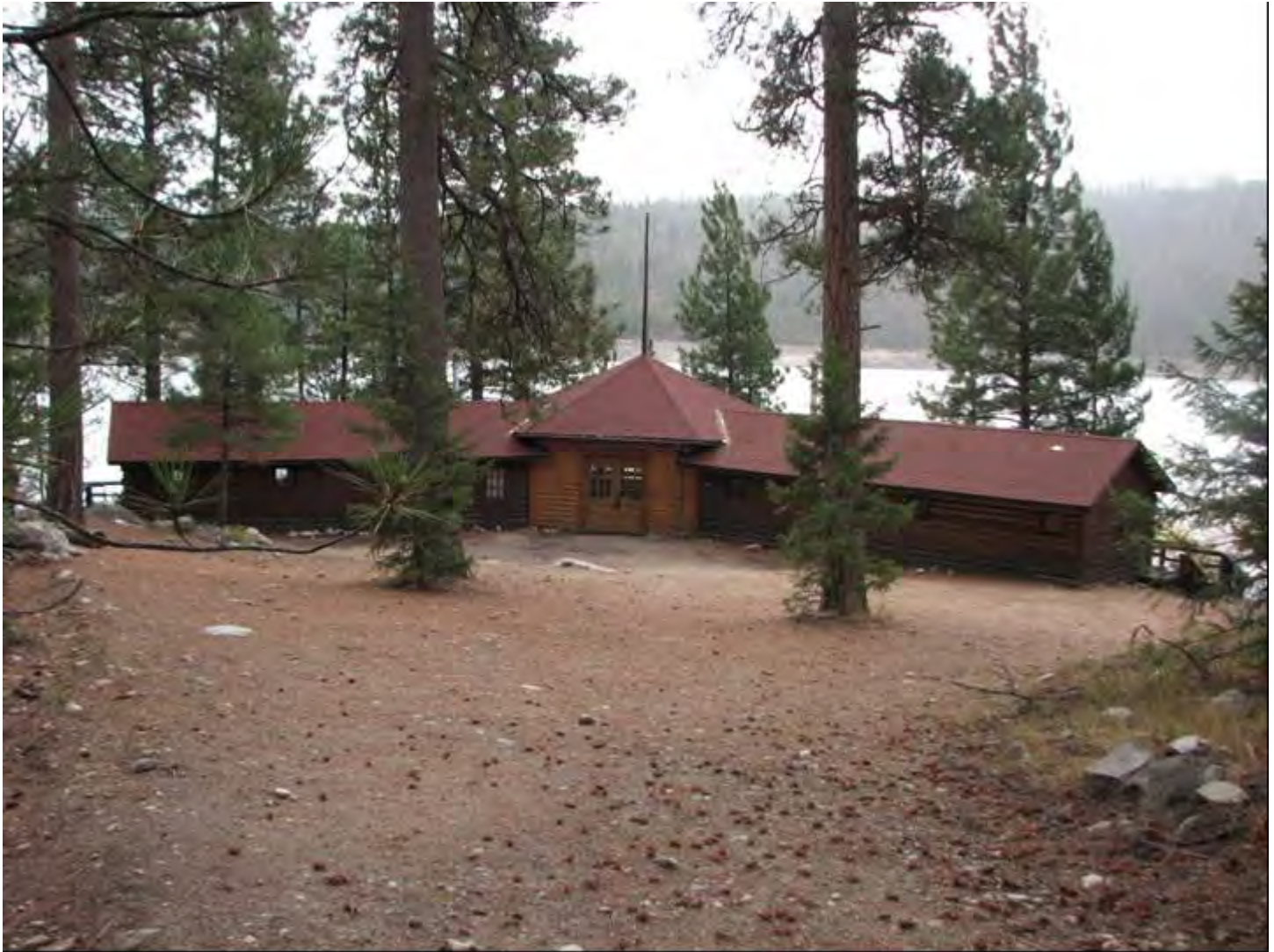
Photo 0002 Looking southeast to Hayward Lodge and the circular drive that accesses the north wall of the building.
