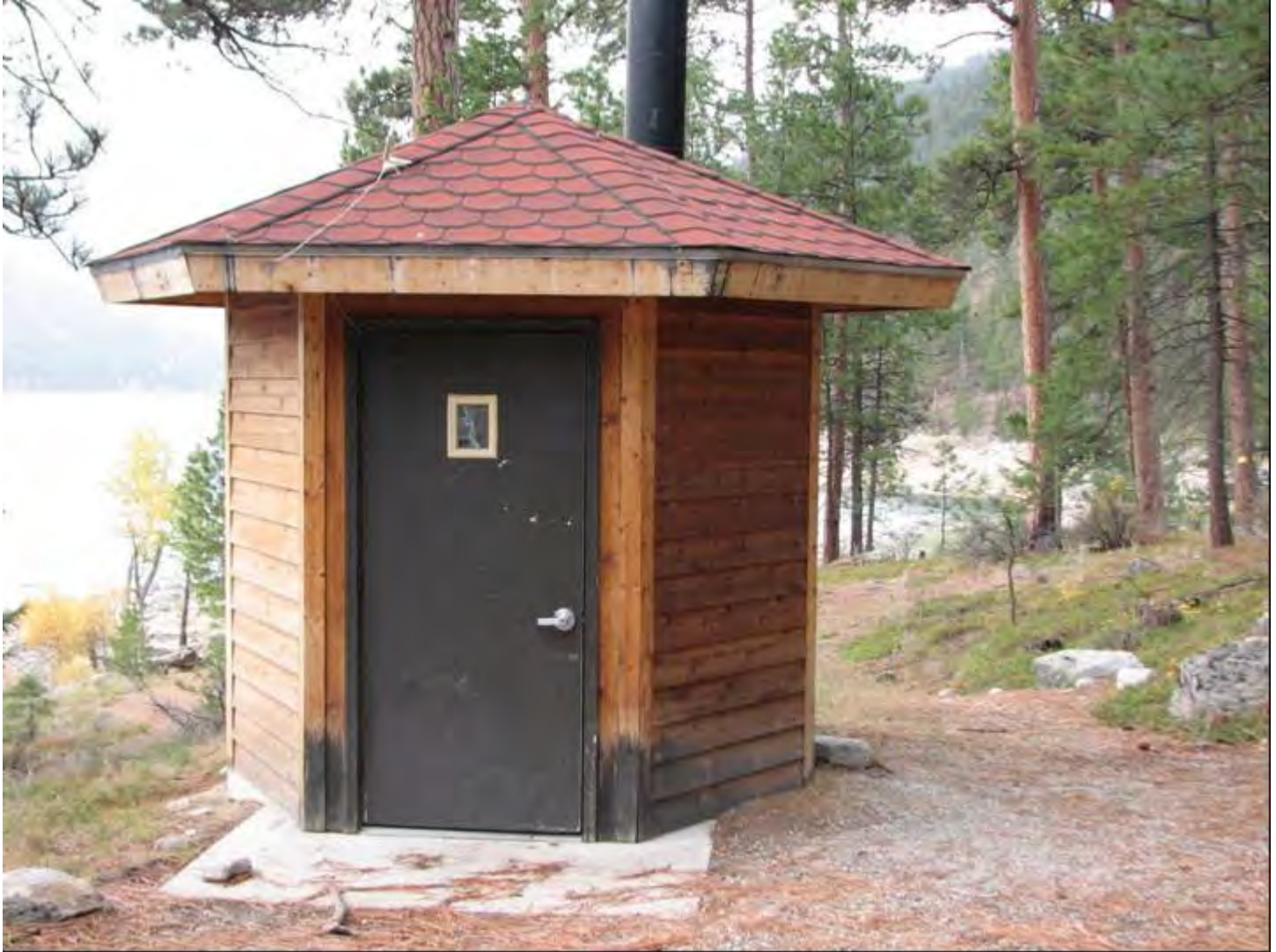
Photo 0018. Hayward Lodge modern vault toilet: looking west.
