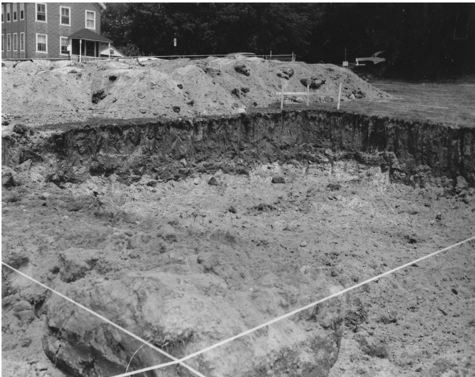
Figure 12. 1971 photo of digging for foundation at current site (Avery Memorial Association).
