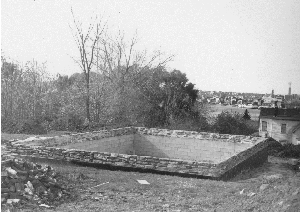
Figure 13. 1971 photo of foundation construction at current site (Avery Memorial Association).
