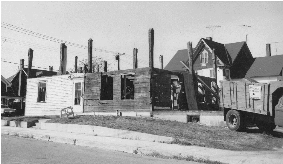
Figure 10. 1971 photo of deconstruction (Avery Memorial Association).
