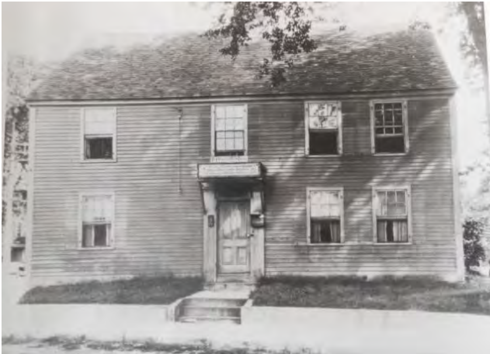
Figure 5. Undated photograph of Avery House taken prior to 1935, before construction of side ell and entrance porch (Avery Memorial Association).
