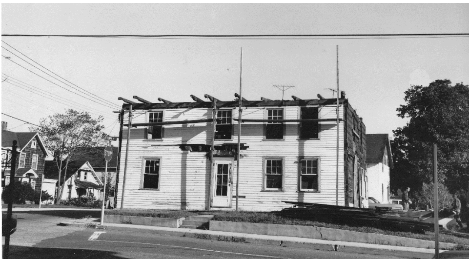
Figure 8. 1971 photo of deconstruction (Avery Memorial Association).
