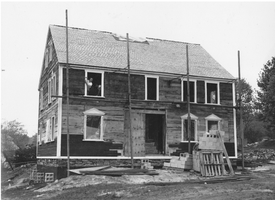
Figure 16. 1971 photo of reconstruction at current site (Avery Memorial Association).
