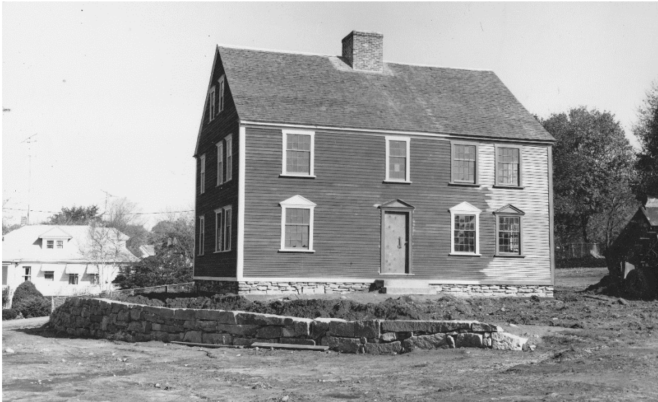
Figure 19. 1971 photo of reconstruction at current site (Avery Memorial Association).
