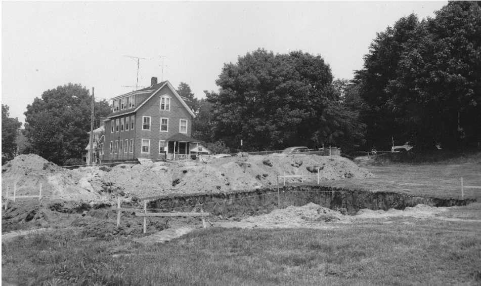
Figure 11. 1971 photo of digging for foundation at current site (Avery Memorial Association).
