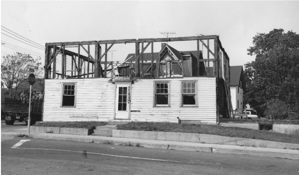
Figure 9. 1971 photo of deconstruction (Avery Memorial Association).
