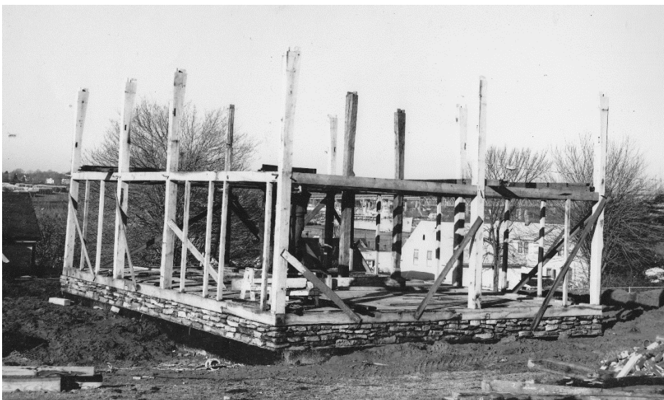
Figure 14. 1971 photo of reconstruction at current site (Avery Memorial Association).
