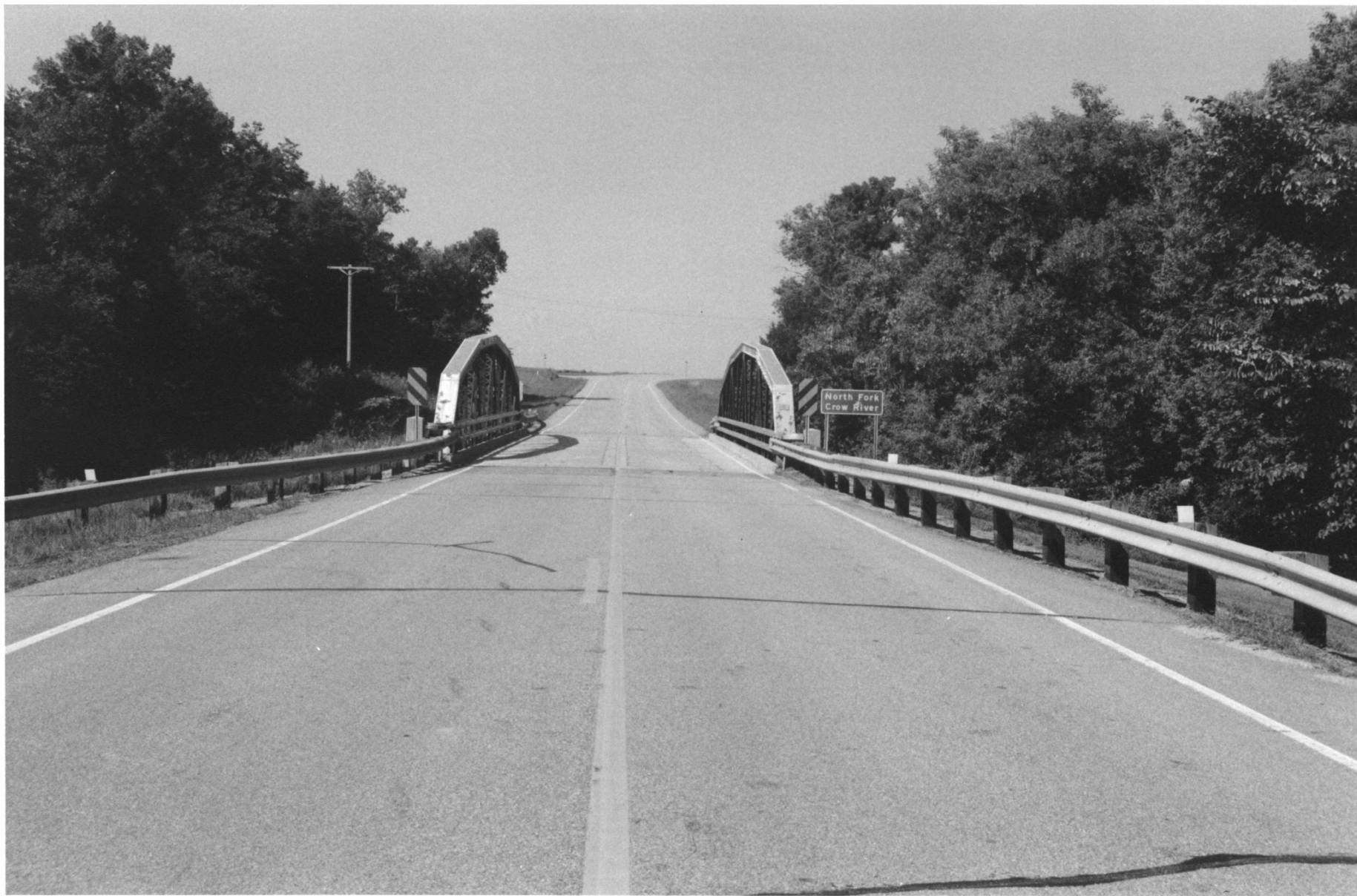
Bridge no. 5388 Mn Highway 24 over North Fork Crow River, Forest City Township Meeker Co., Mn 013059-4
