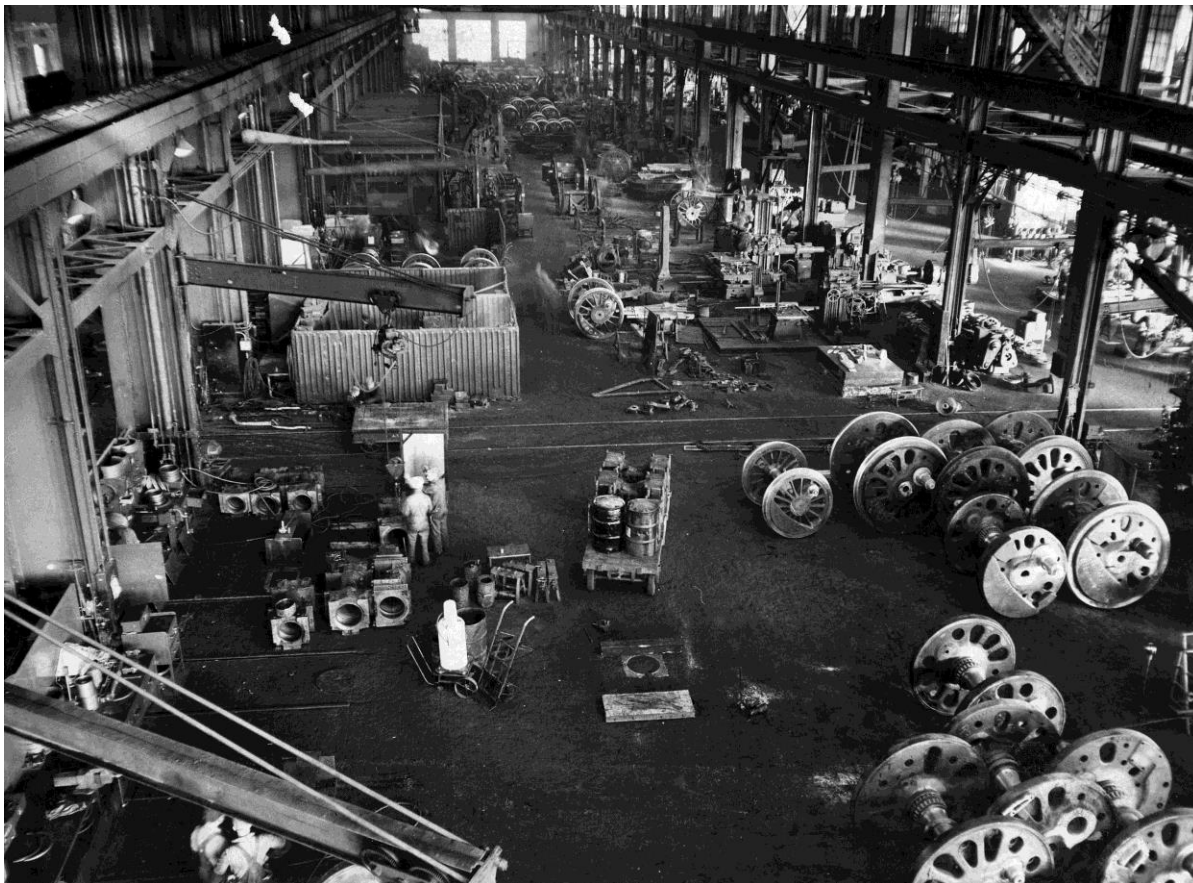
Figure 4. Machine shop with locomotive parts in the heavy machinery bay, looking east.
