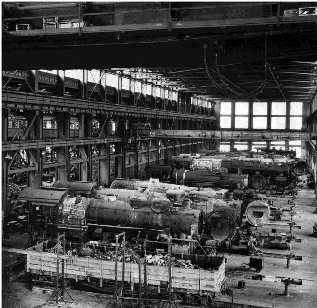
Figure 3. Machine shop with locomotives in the erecting bay, looking southwest. Note concrete pits and 250-ton bridge crane in background.
