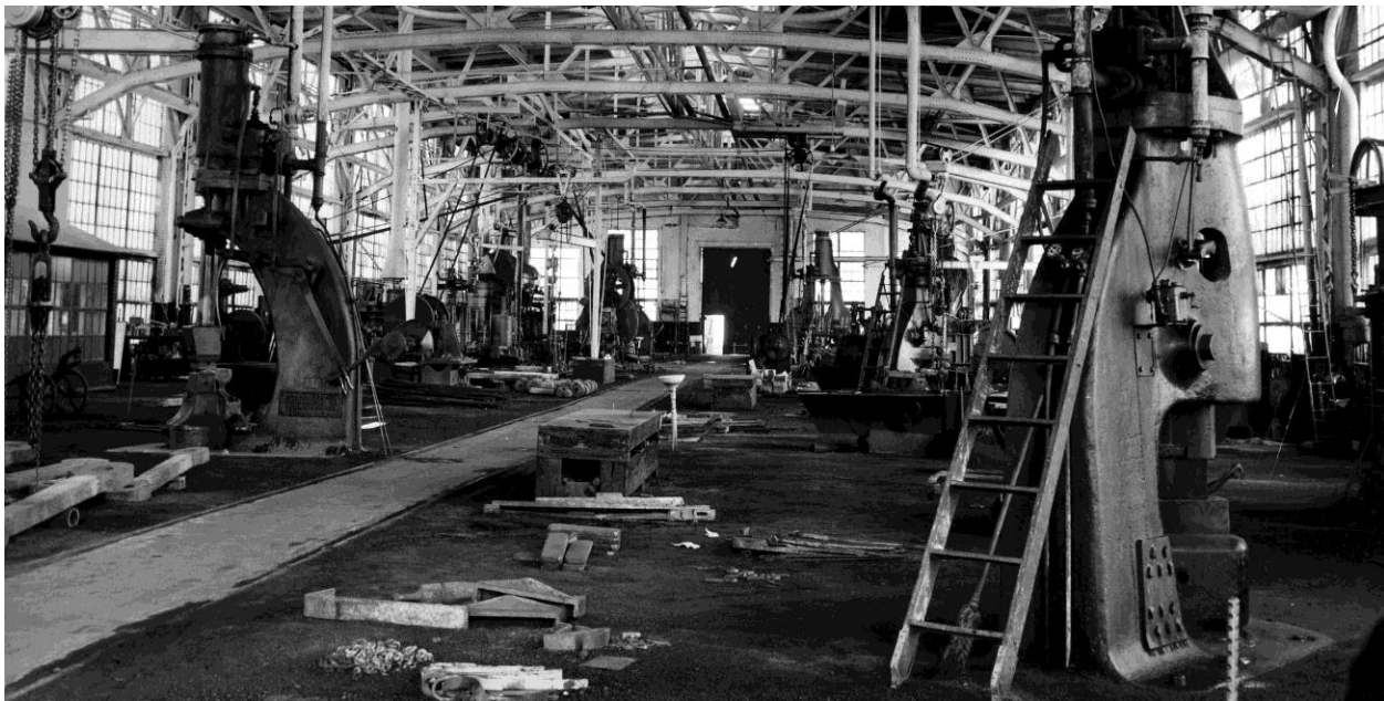
Figure 7. Blacksmith shop with large presses. Steel trusses span the interior.
