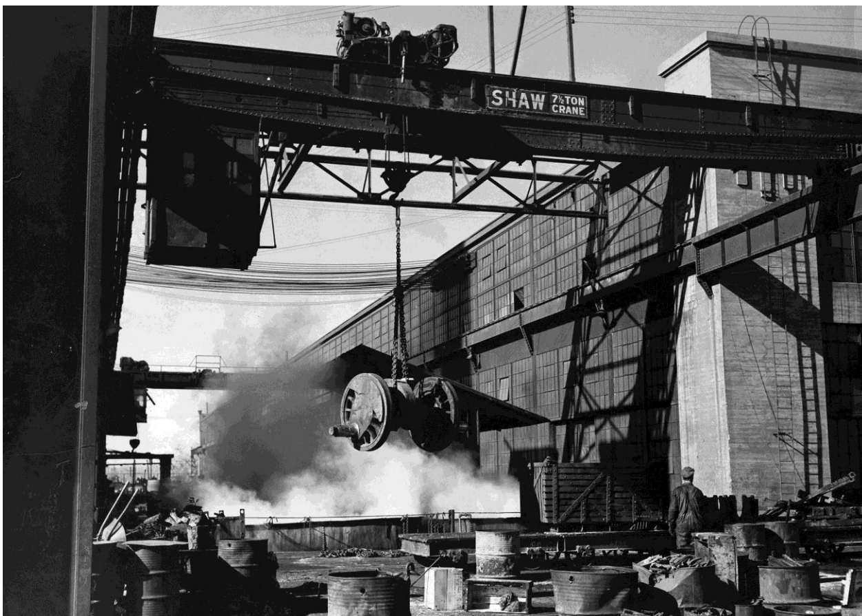
Figure 5. Crane runway with bridge cranes on the south side of the machine shop.
