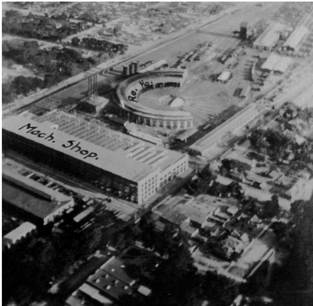
Figure 11. AT&SF shops with roundhouse, reservoir and tanks, power house and smokestack, and machine shop. View looking southwest.
