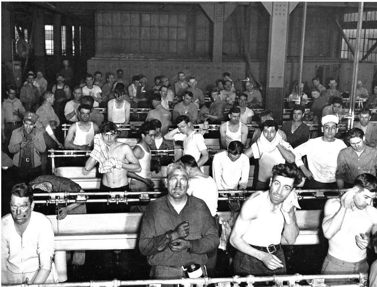
Figure 12. Washroom on mezzanine in machine shop with workmen washing up at the end of the day.
