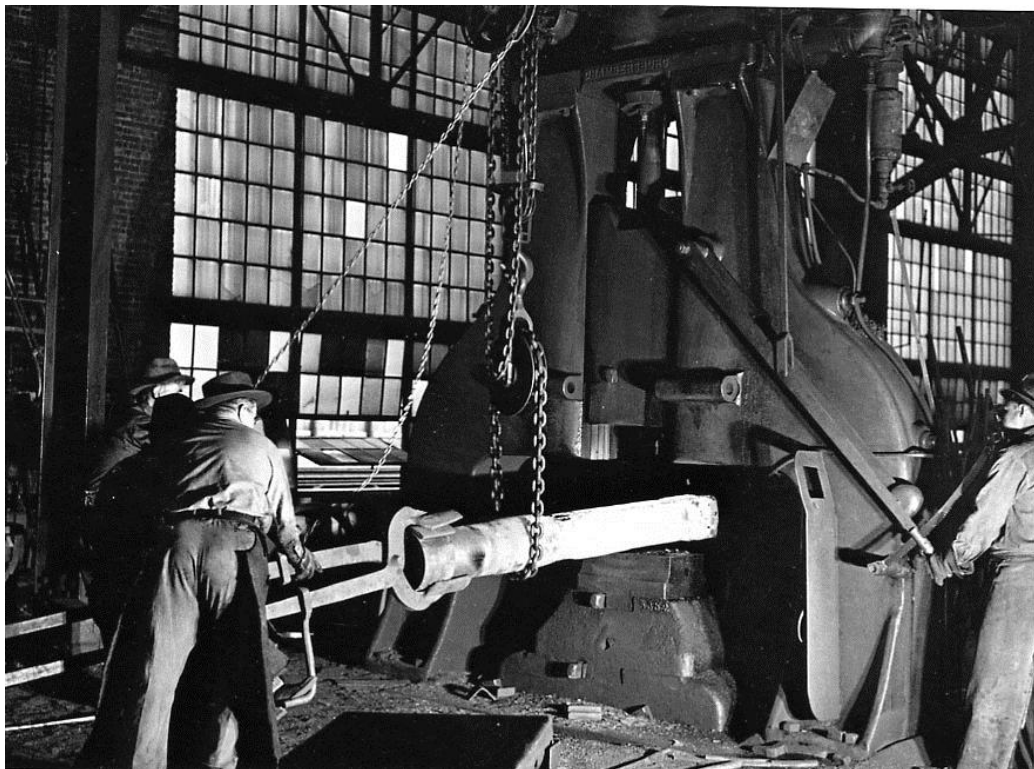
Figure 8. Blacksmith shop with men hammering a drawbar with a steam hammer.
