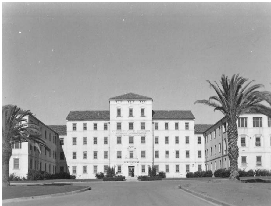
Figure 76: Subarea 4—Neuropsychiatric (N.P.) Hospital, Building 258 (extant), view north (VA Archives, nd)
