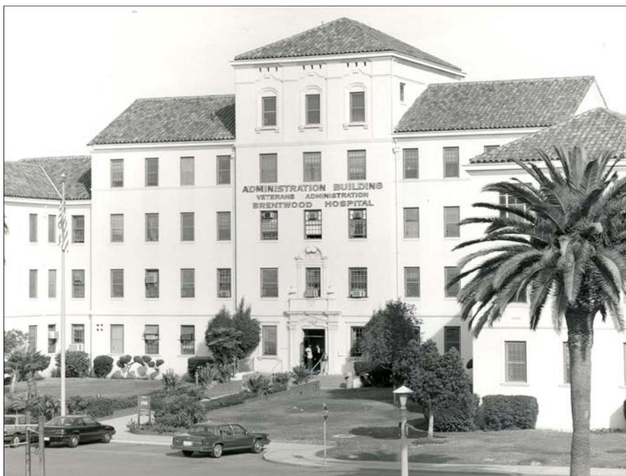
Figure 78: Subarea 4—Neuropsychiatric (N.P.) Hospital, Building 258 (extant), view northwest (VA Archives, circa 1980s)
