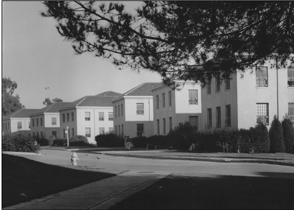
Figure 79: Subarea 4—Neuropsychiatric (N.P.) Hospital, Buildings 206 (left) and 207 (right, extant), view southeast (VA Archives, nd)
