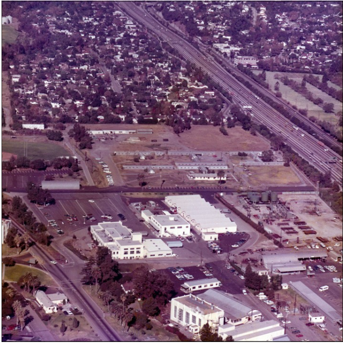
Figure 94: Subarea 5—Utility, view north (VA Archives, circa 1984)
