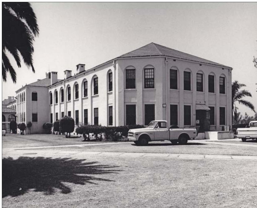
Figure 72: Subarea 4—Neuropsychiatric (N.P.) Hospital, Building 156 (extant), view southwest (VA Archives, 1972)
