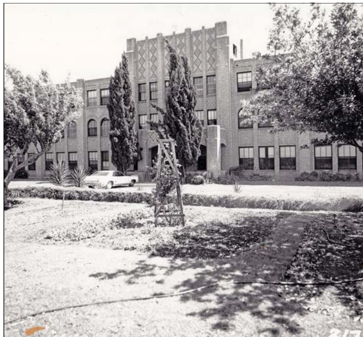
Figure 65: Subarea 3—Research, Building 116, view northwest (VA Archives, nd)
