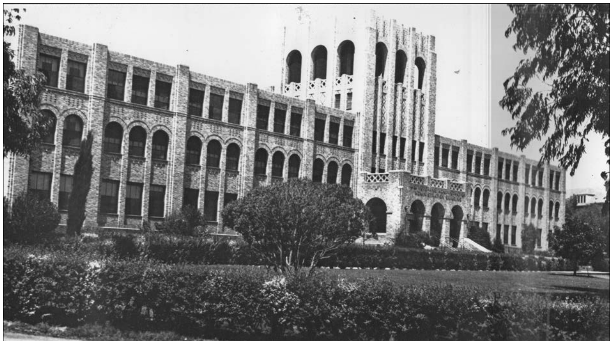
Figure 62: Subarea 3—Research, Building 114, view northeast (VA Archives, nd)
