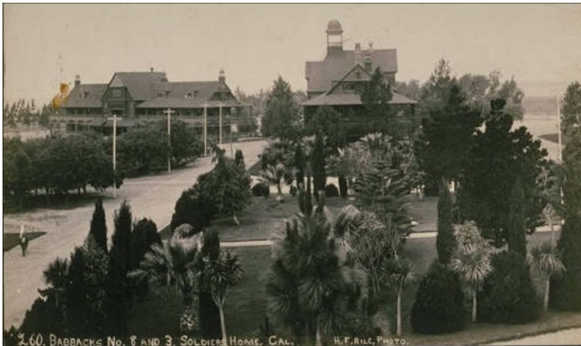
Figure 14: Subarea 1—Domiciliary, Barracks #8 (left, not extant) and #3 (right, not extant), view west (Santa Monica Public Library, 1890)
