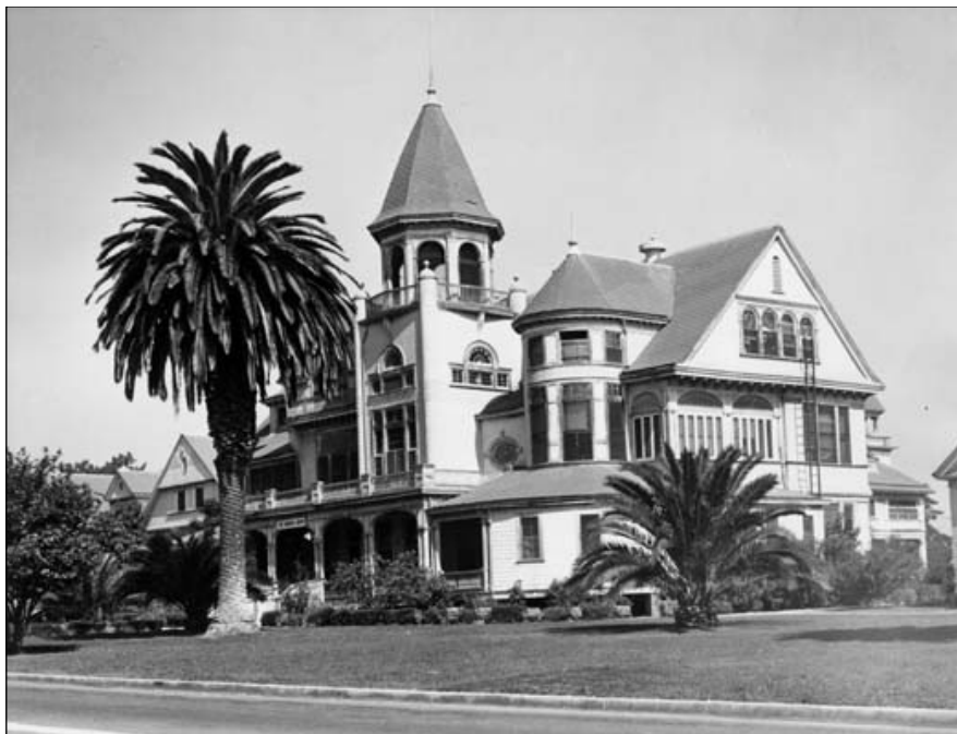
Figure 28: Subarea 1—Domiciliary, Barrack #6 (not extant), view north-east (Los Angeles Public Library, 1939)
