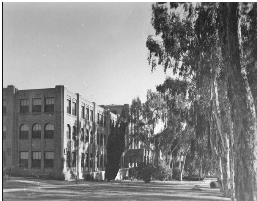
Figure 67: Subarea 3—Research, Building 115, view south (VA Archives, nd)
