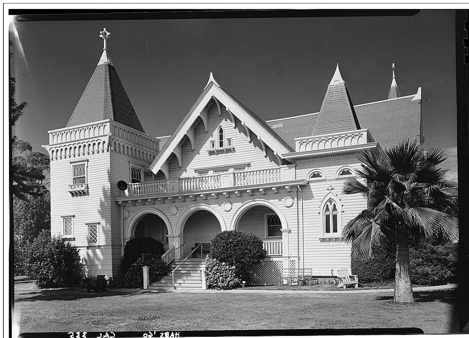
Figure 40: Subarea 1—Domiciliary, Chapel, view north (HABS CAL,19-LOSAN,12A-1, 1960)
