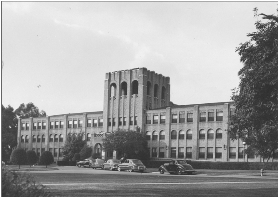
Figure 64: Subarea 3—Research, Building 114, view northeast (VA Archives, nd)
