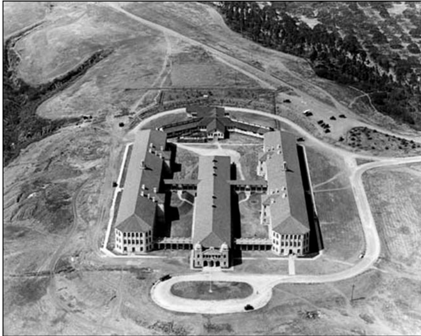
Figure 69: Subarea 4—Neuropsychiatric (N.P.) Hospital, Buildings 156, 157, and 158 (extant), view northwest (VA Archives, circa 1930)
