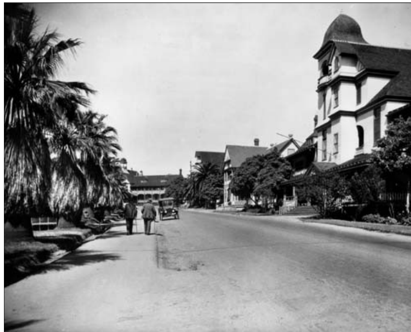
Figure 18: Subarea 1—Domiciliary, view west, note Barrack #1 (not extant) at right (Los Angeles Public Library, circa 1915)
