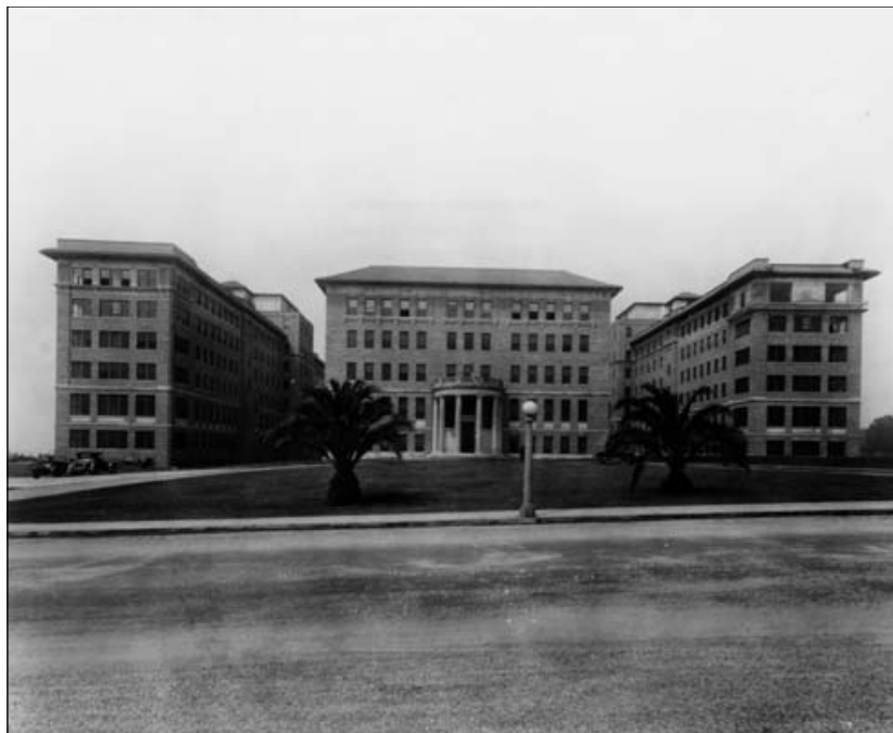
Figure 98: Subarea 7—General Hospital, Wadsworth Hospital (not extant) under construction, view west (Los Angeles Public Library, circa 1925)
