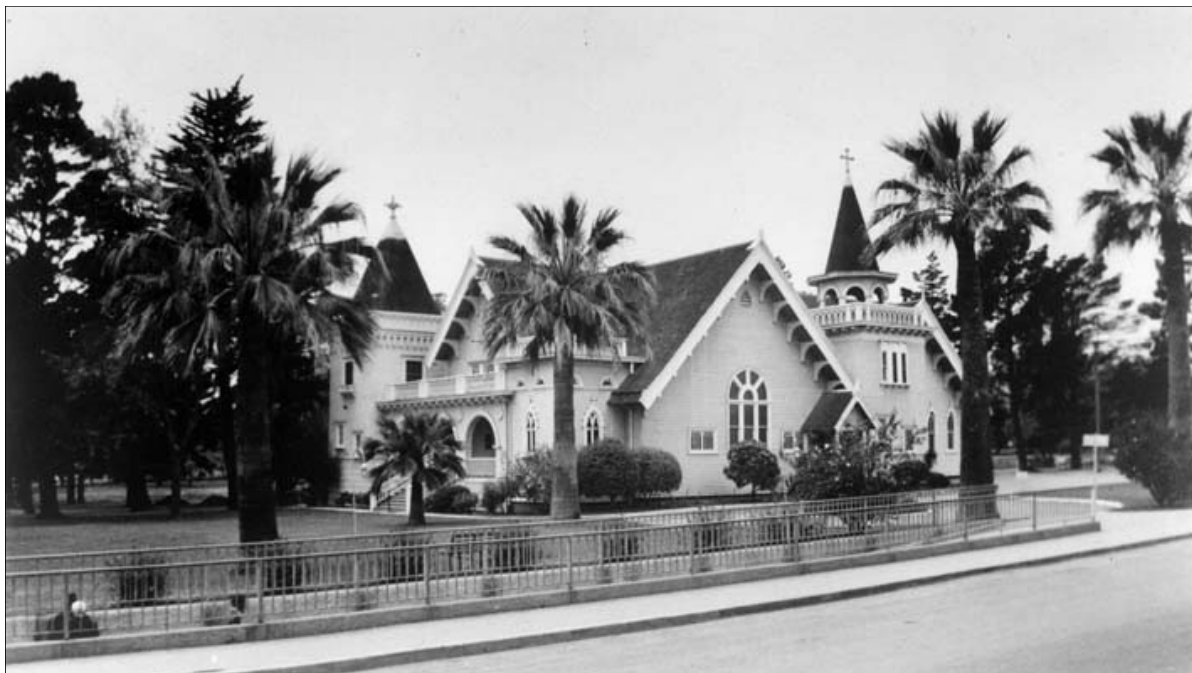
Figure 36: Subarea 1—Domiciliary, Chapel, view northwest (Los Angeles Public Library, 1941)
