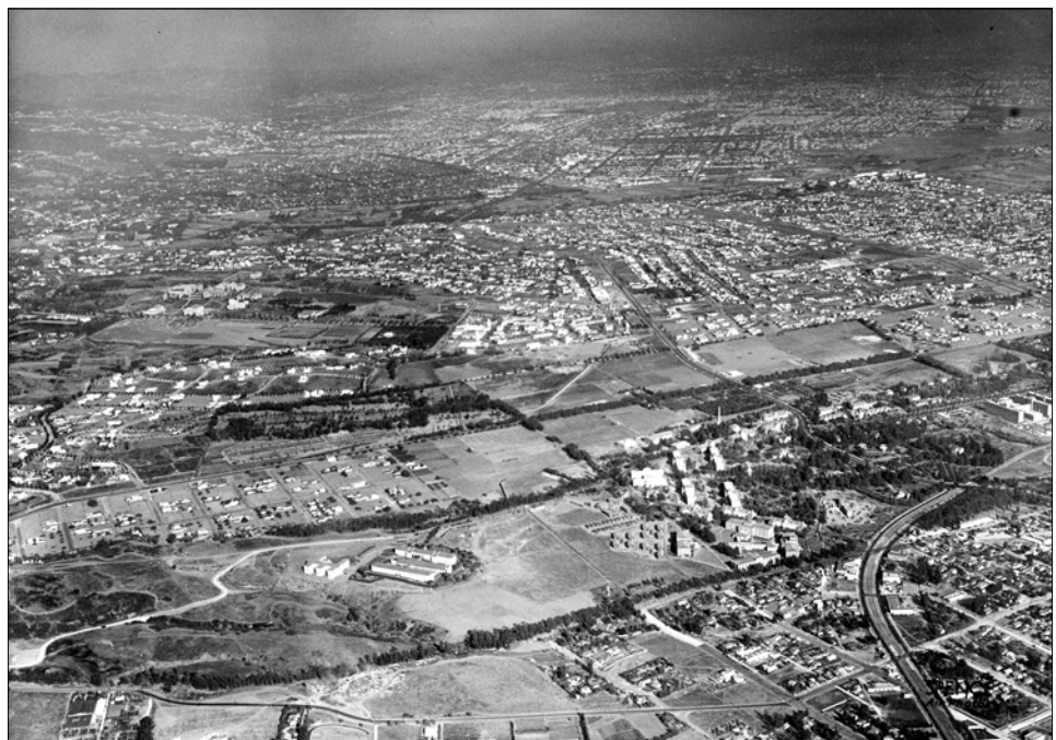
Figure 4: Aerial view of campus, view southeast (University of California Los Angeles Air Photo Archives, Spence Collection, 1938)
