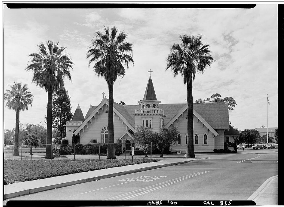
Figure 39: Subarea 1—Domiciliary, Chapel, view west (HABS CAL,19-LOSAN,12A-1, 1960)
