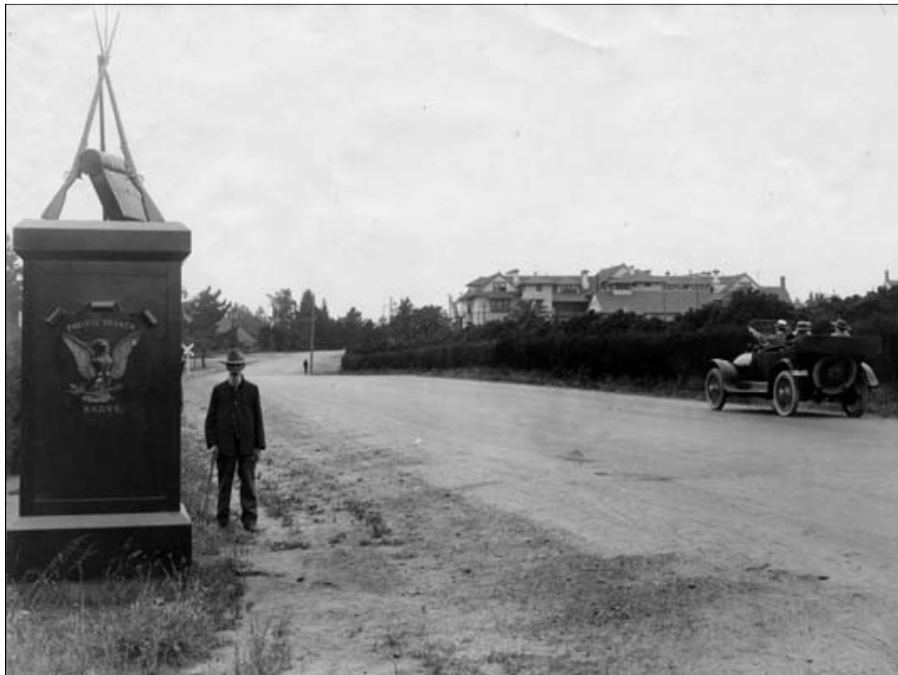
Figure 61: Subarea 3—Research, gate at San Vicente Boulevard, view east, note railroad crossing in background (Los Angeles Public Library, circa 1915)
