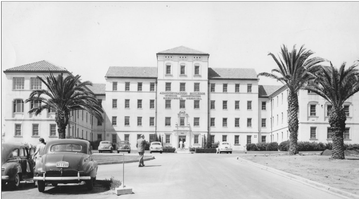
Figure 75: Subarea 4—Neuropsychiatric (N.P.) Hospital, Building 258 (extant), view northwest (VA Archives, circa 1950s)
