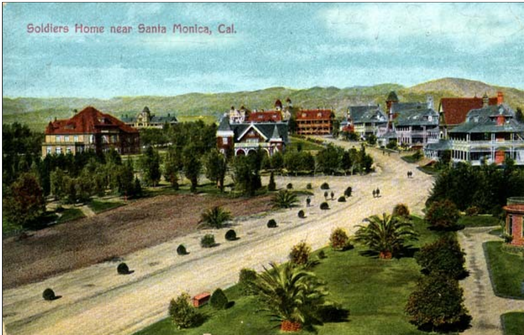
Figure 6: Subarea 1—Domiciliary, view northwest along Bonsall Avenue (Los Angeles Public Library, circa 1900)
