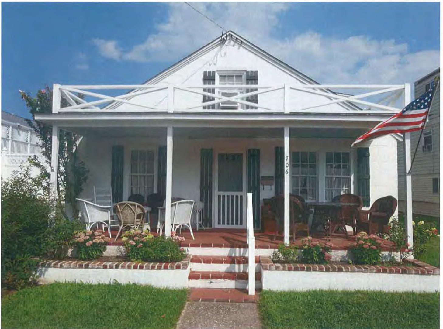
MD_WorcesterCounty_CraigCaptainRobertSCottage_0001.tif West façade 1 of 16
